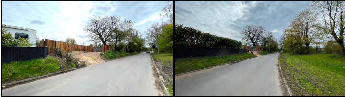
Figure 2 - Photographs of Site from Hitchin Road
