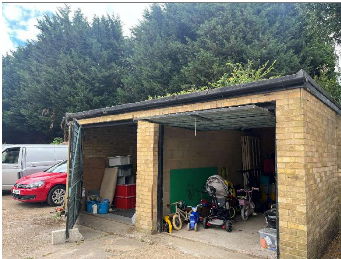
Figure 2: View of B1 taken from the northern elevation
