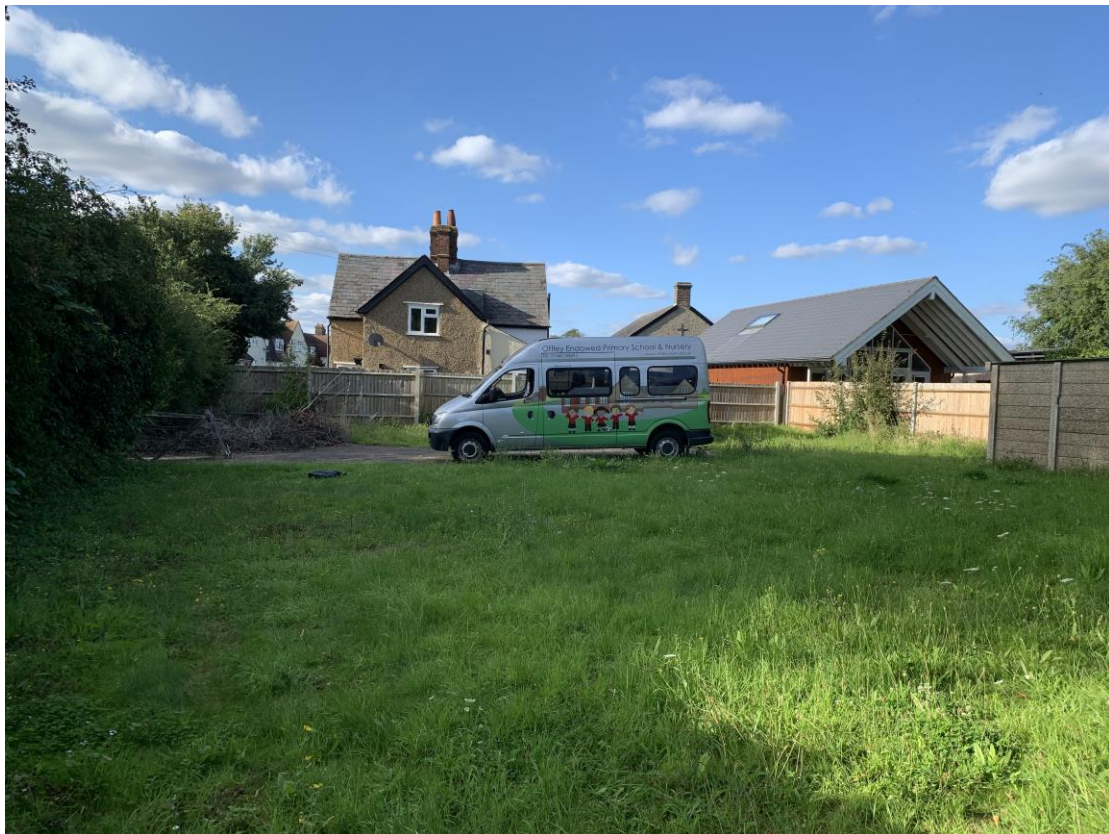
Photo B showing overhang to Classroom roof on north boundary.
