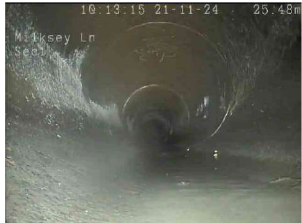
7b70e5a9-b297-4289-a504-2282be5e6a94.png, 00:01:30, 25.50 m Roots, fine at joint, finish
