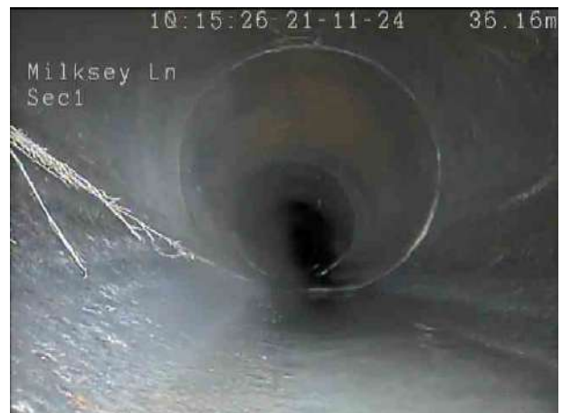
eb8eaf-11ce-49ac-99d1-1b747c865bb6.png, 00:03:41, 36.60 m Roots, fine at joint, finish
