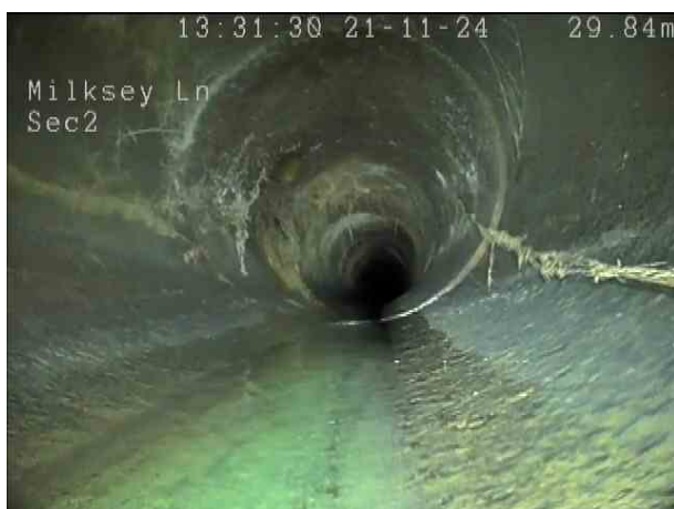
22677a1c-9702-415a-b762-6022f4cc53ea.png, 00:02:26, 30.30 m Roots, fine at joint
