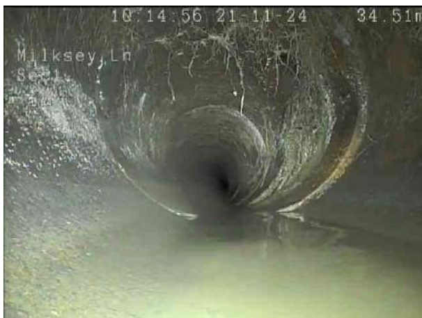
f539d5c1-cff1-4d3c-b9ef-aa45644b736d.png, 00:03:10, 35.00 m Junction at 2 o'clock, 250mm dia
