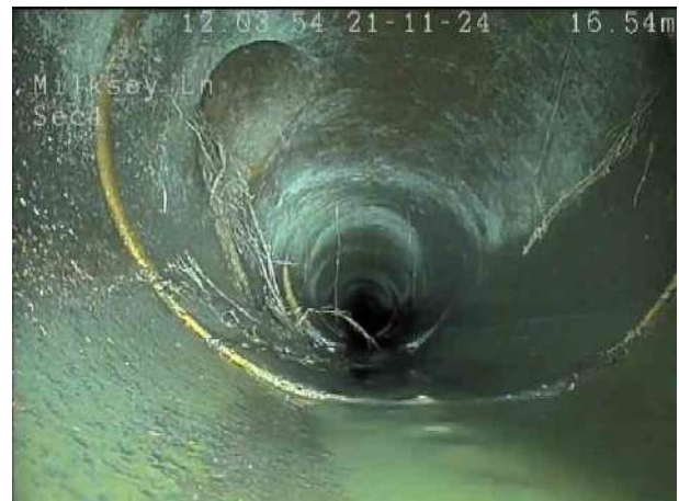
777f24de-9b4a-467c-a4c1-97b24560e6a4.png, 00:01:31, 16.90 m Junction at 10 o'clock, 150mm dia
