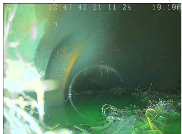
4eba2138-032a-41ca-878b-b013038afdcd.png, 00:01:40, 10.30 m Junction at 9 o'clock, 225mm dia
