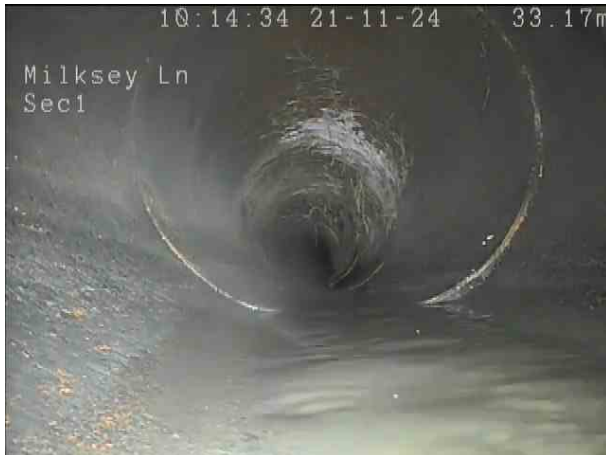
93e7a674-413d-43cd-a0ed-10f057f7ce26.png, 00:02:48, 33.50 m Roots, fine at joint, finish
