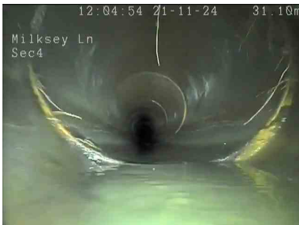
630009ea-0182-45c2-8f0f-673835fbabb3.png, 00:02:30, 31.30 m Roots, fine at joint
