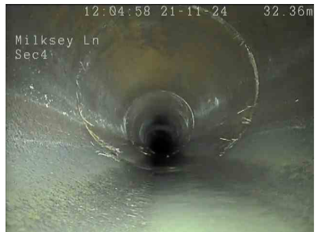
ced64048-de0d-4066-a821-b95732ef483e.png, 00:02:35, 32.80 m Roots, fine at joint
