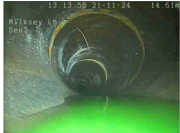
76ad6ec8-b119-4354-9085-b3d31c6acbea.png, 00:01:50, 15.00 m Roots, fine at joint
