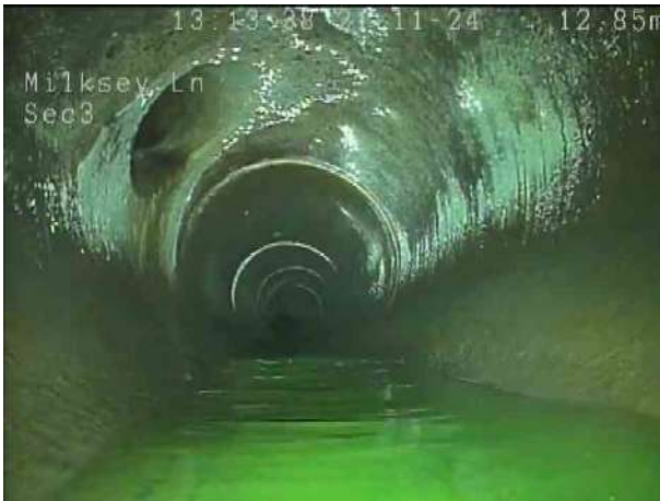
ced530b9-5c45-4fb0-bd8a-c44cf9934782.png, 00:01:38, 13.20 m Junction at 10 o'clock, 150mm dia
