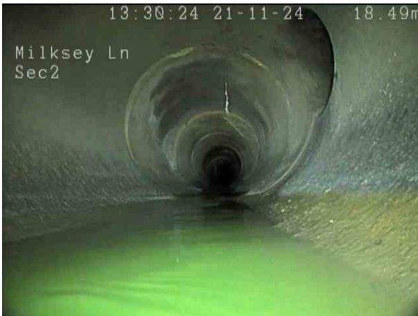
cc336df9-275d-4a12-b918-de934bef365d.png, 00:01:20, 19.00 m Junction at 2 o'clock, 150mm dia
