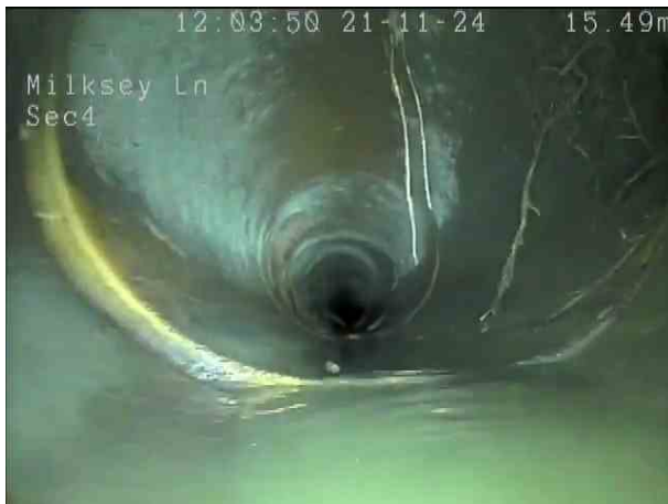
a0bce399-a450-4d3d-a9e2-3ac84516f48a.png, 00:01:27, 15.80 m Roots, fine at joint
