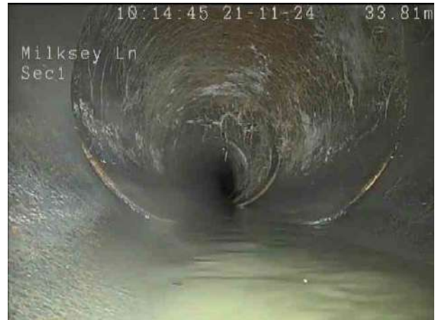
d3dc2325-8fee-4084-b3ff-8aad911865d1.png, 00:03:00, 34.00 m Roots, fine at joint, start
