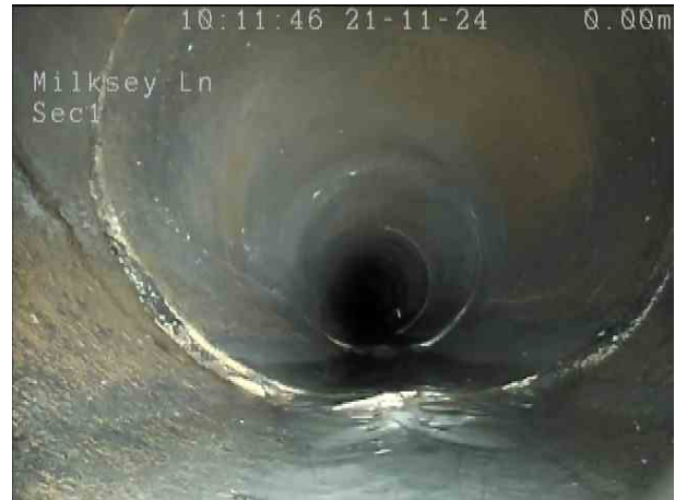
71a36dd9-3d53-40b7-b06d-b984787a84b6.png, 00:00:01, 0.00 m Water level, 5% of the vertical dimension, Running live
