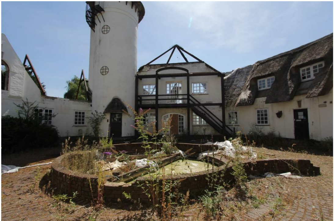
View of the existing internal courtyard
