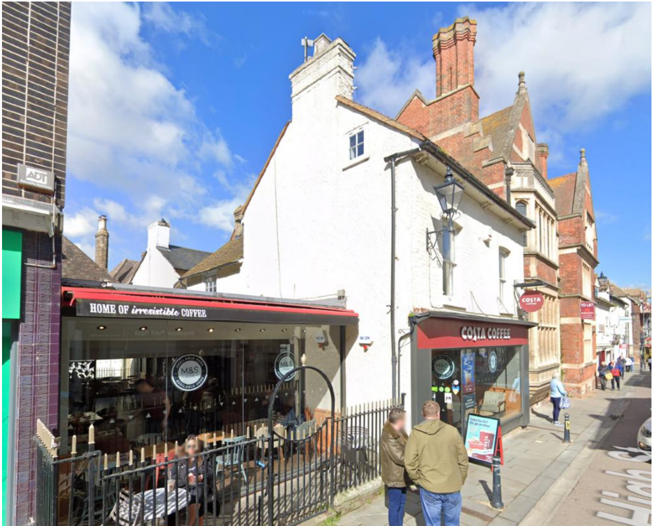
Figure 1 - Costa Royston Front Elevation (Courtesy of Google Maps)
