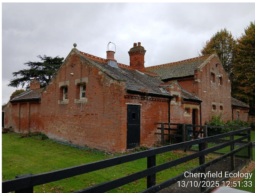
Figure 12: Rear of B3.
