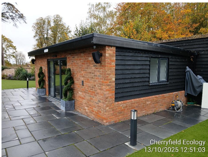
Figure 18: Exterior of B5.
