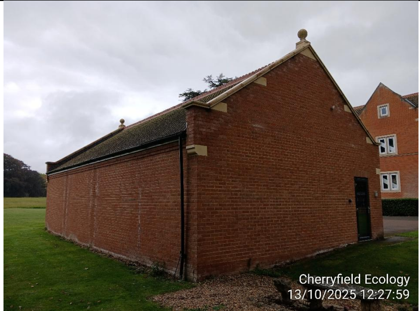
Figure 9: Rear of B2.
