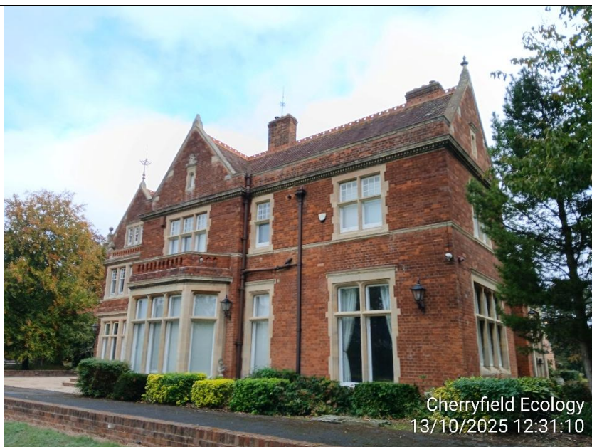
Figure 5: Exterior of B1.
