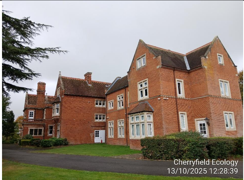
Figure 3: Exterior of B1.
