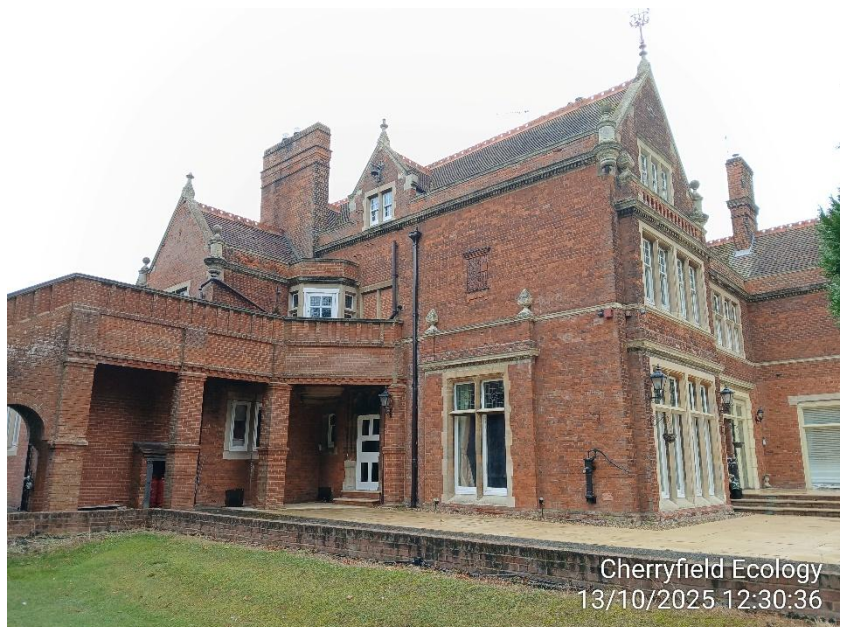
Figure 4: Exterior of B1.
