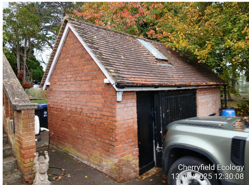
Figure 16: Exterior of B4.
