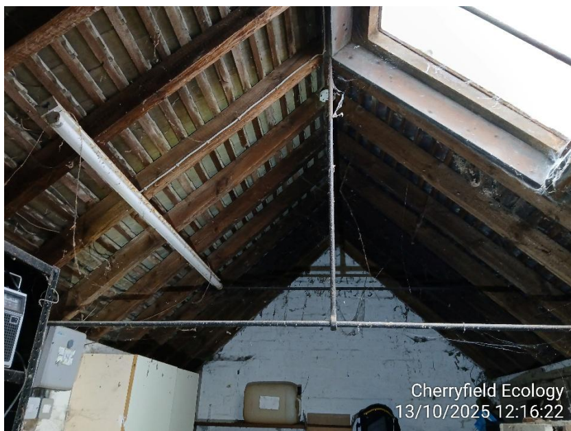
Figure 17: Interior of B4.
