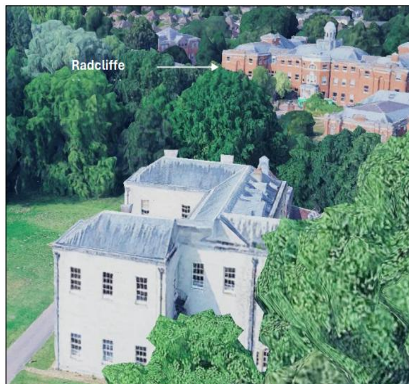
Figure 8: 3D illustrative views of the spatial relationship of The Priory and its associated Listed Buildings and Radcliffe House (Source: Google Earth, 2026)
