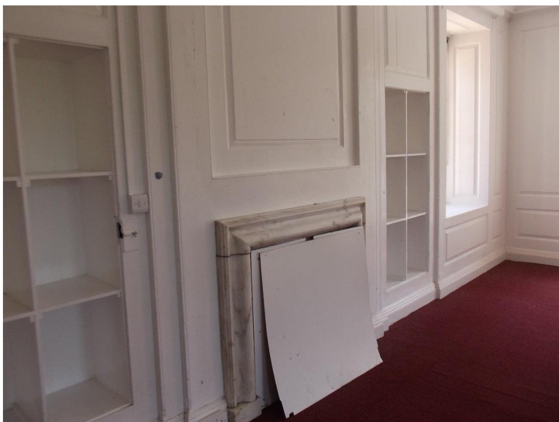
64. Fireplace in east wall
