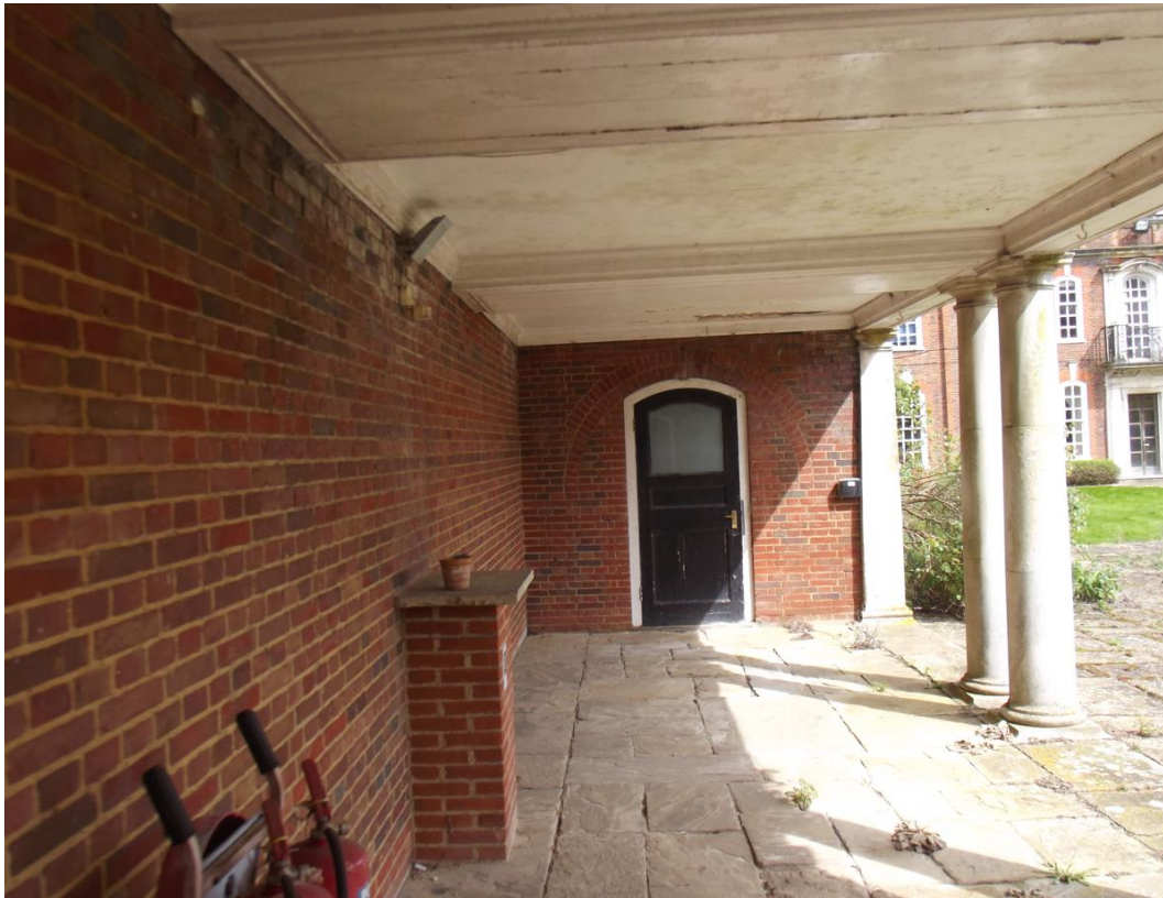
107. Loggia looking to east pavilion
