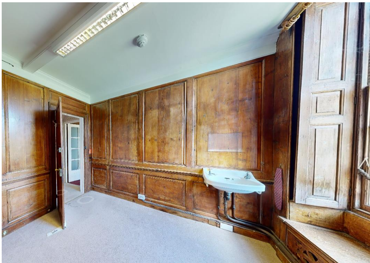
35. Main north bedroom with window seat and shutters and Lutyens panelling, but with 20 th century sink
