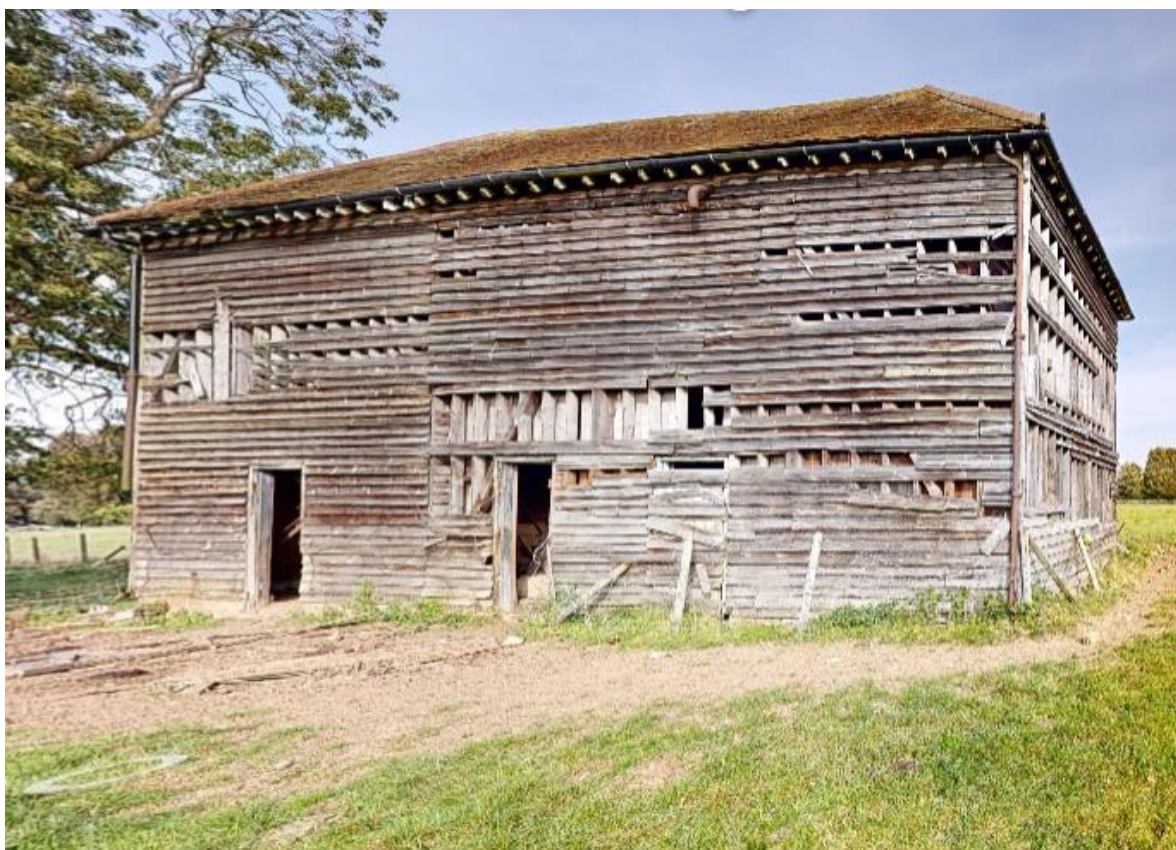
121. Tank House west elevation
