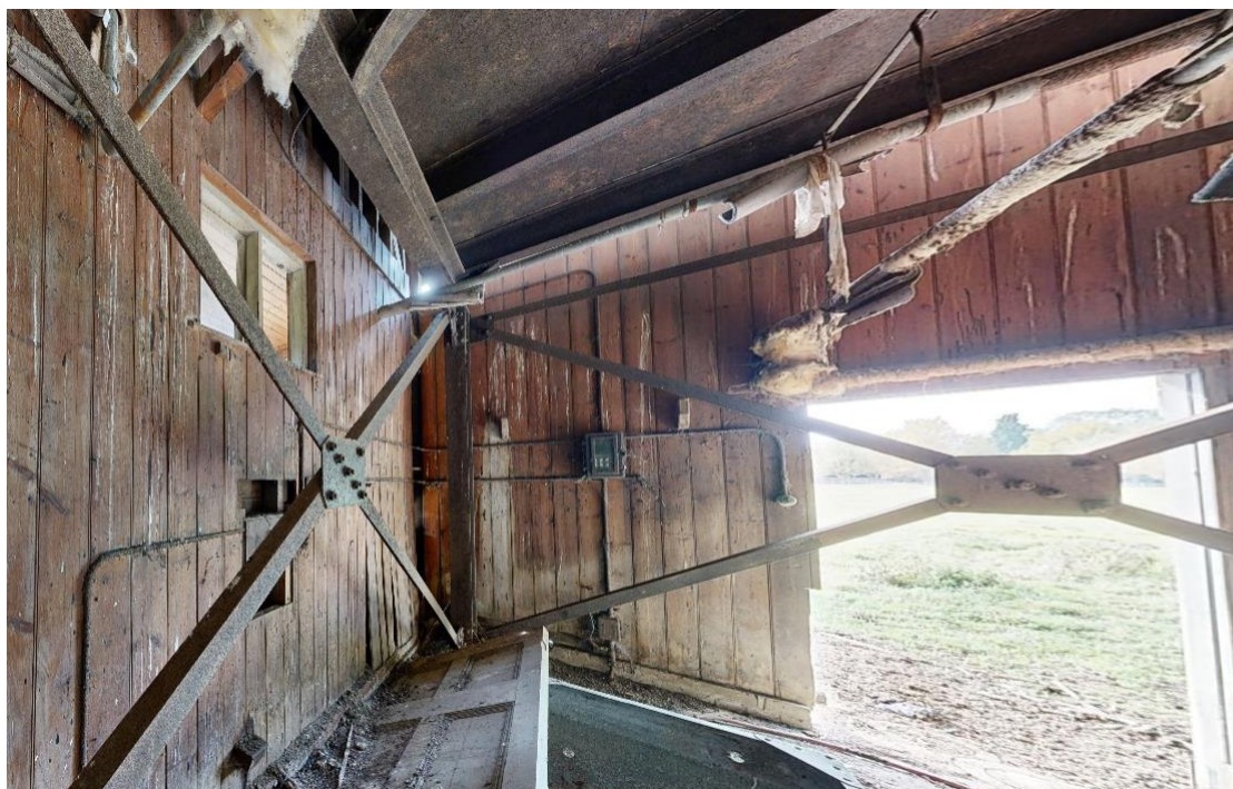
122. Tank house north section looking west showing metal restraining braces
