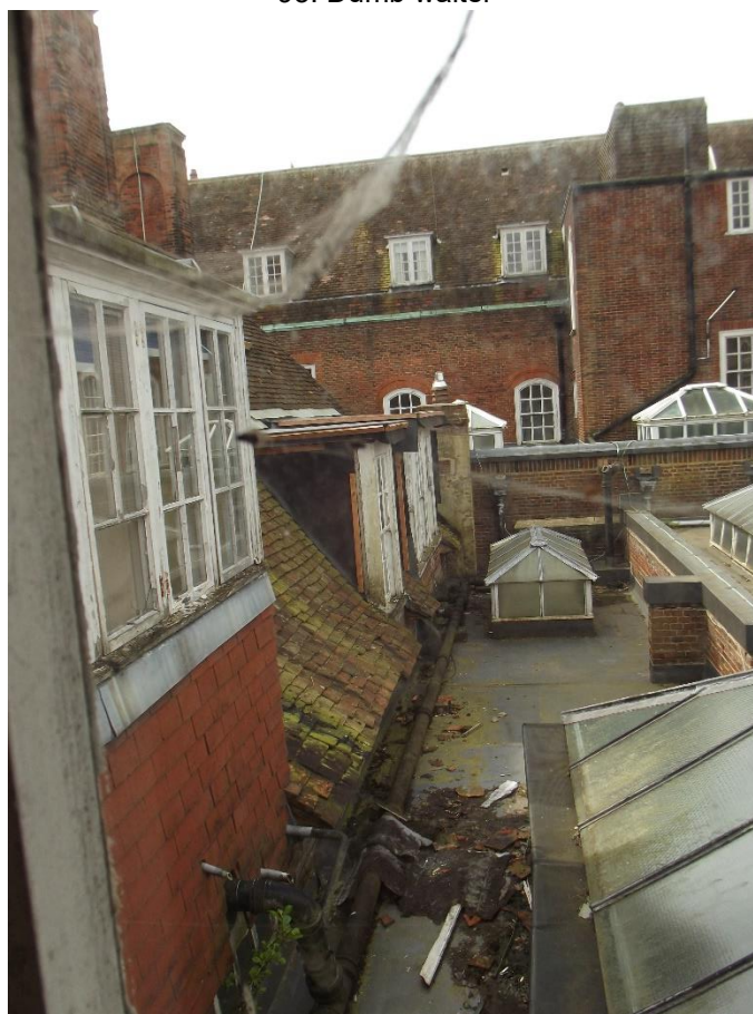
94. Rooftop view across the school dining room with roof lanterns. The pair of taller lanterns to the rear light the school hall
