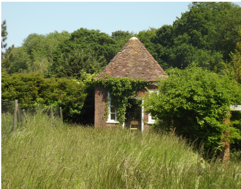
111. The belvedere from the west
