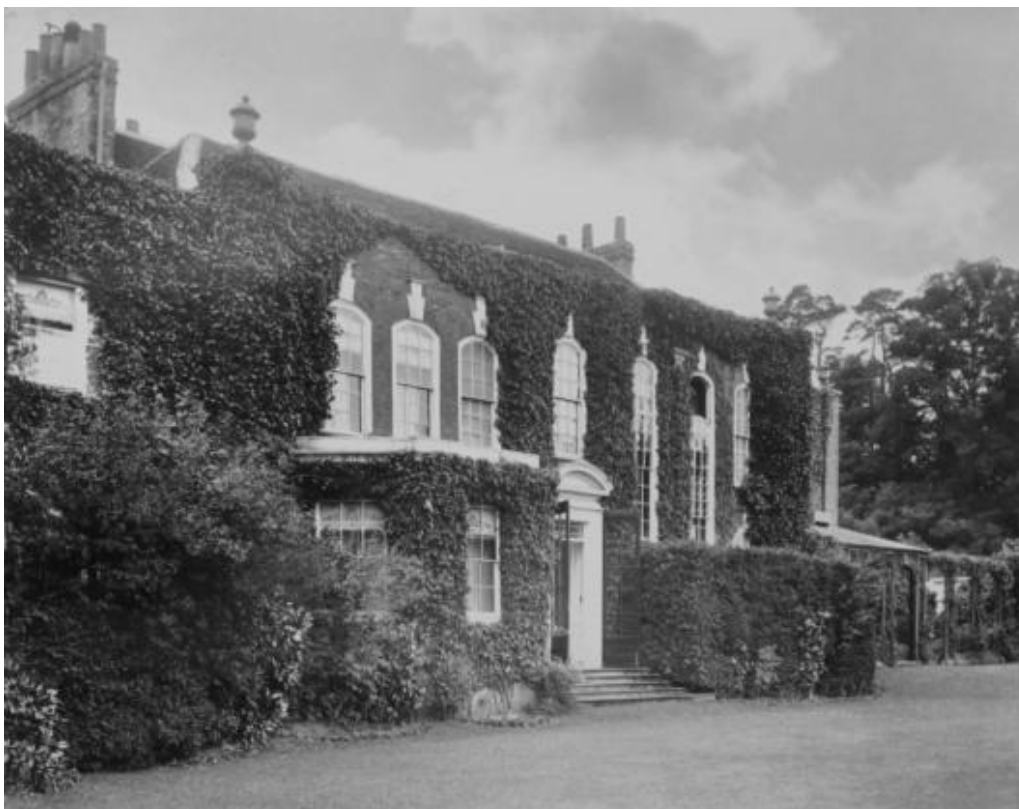
Fig. xxii North Elevation details including the bay window and the rear of the verandah.
