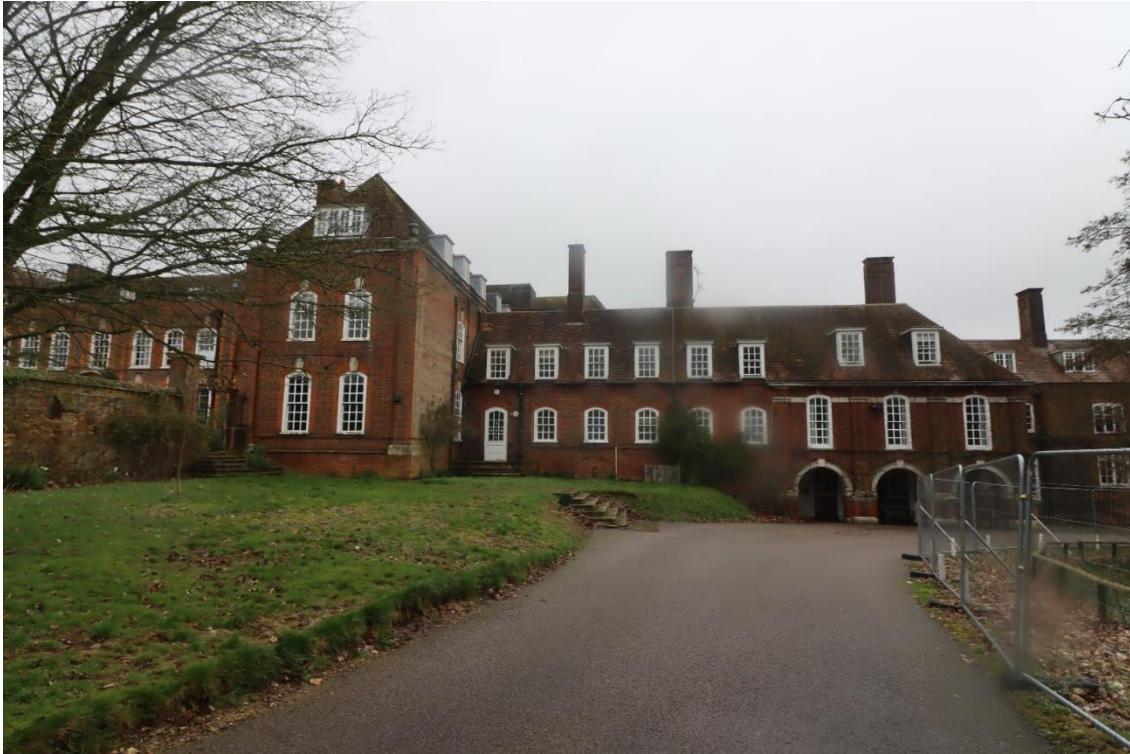
7 East (service) wing with East Annexe extended by Lutyens 1911-13
