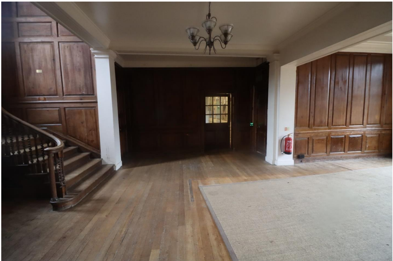
22. Staircase Hall looking east. The half glazed door is later and leads into the corridor connecting the Old House with Lutyens service wing and the dining room. A second door next to the stairs leads to a back door in the north wall.
