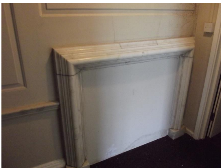
57. Former bedroom fireplace located in corridor
