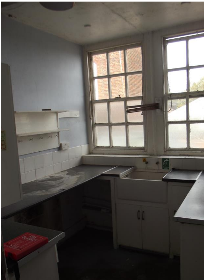
39. Second floor north side
