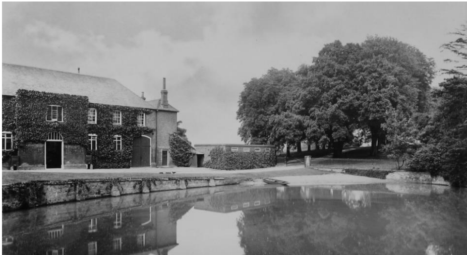
Fig. xx Stable range with 19 th century extension, wall and gateway on the eastern end
