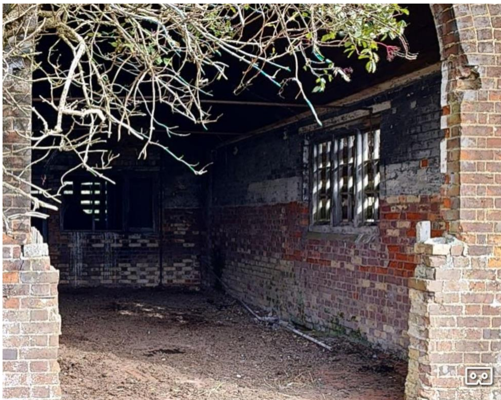
118. Central section interior
