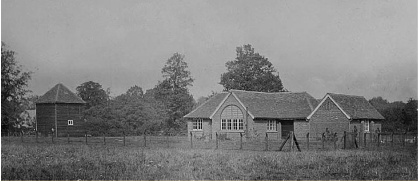
Fig. lxxv Pumping Station c.1913 with Tank House on the left
