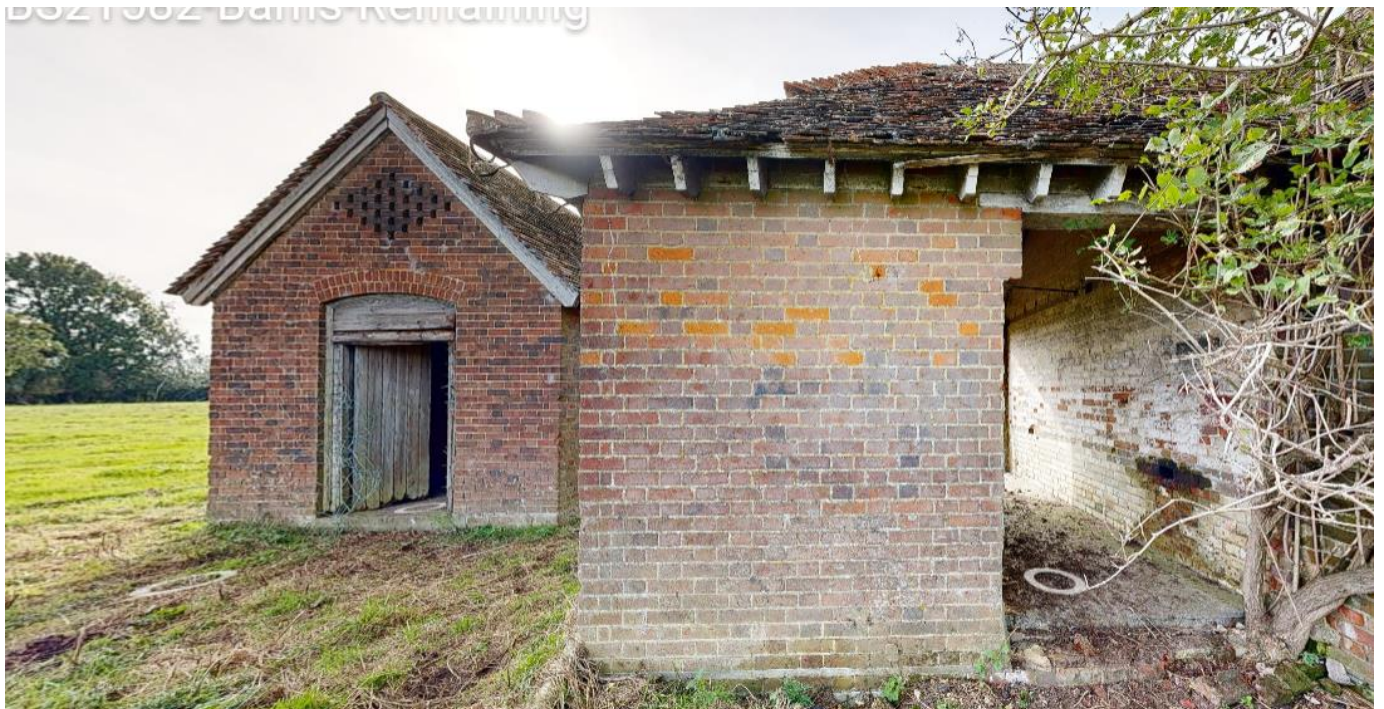
116. Pump House east elevation with well house to the left & south wing of central section to right
