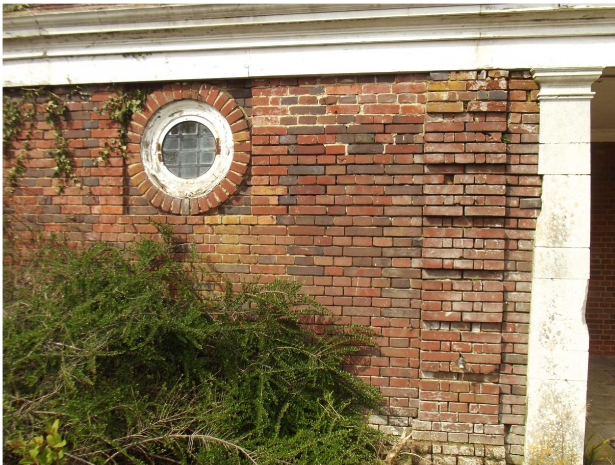
109. Brickwork repair on south wall of west pavilion
