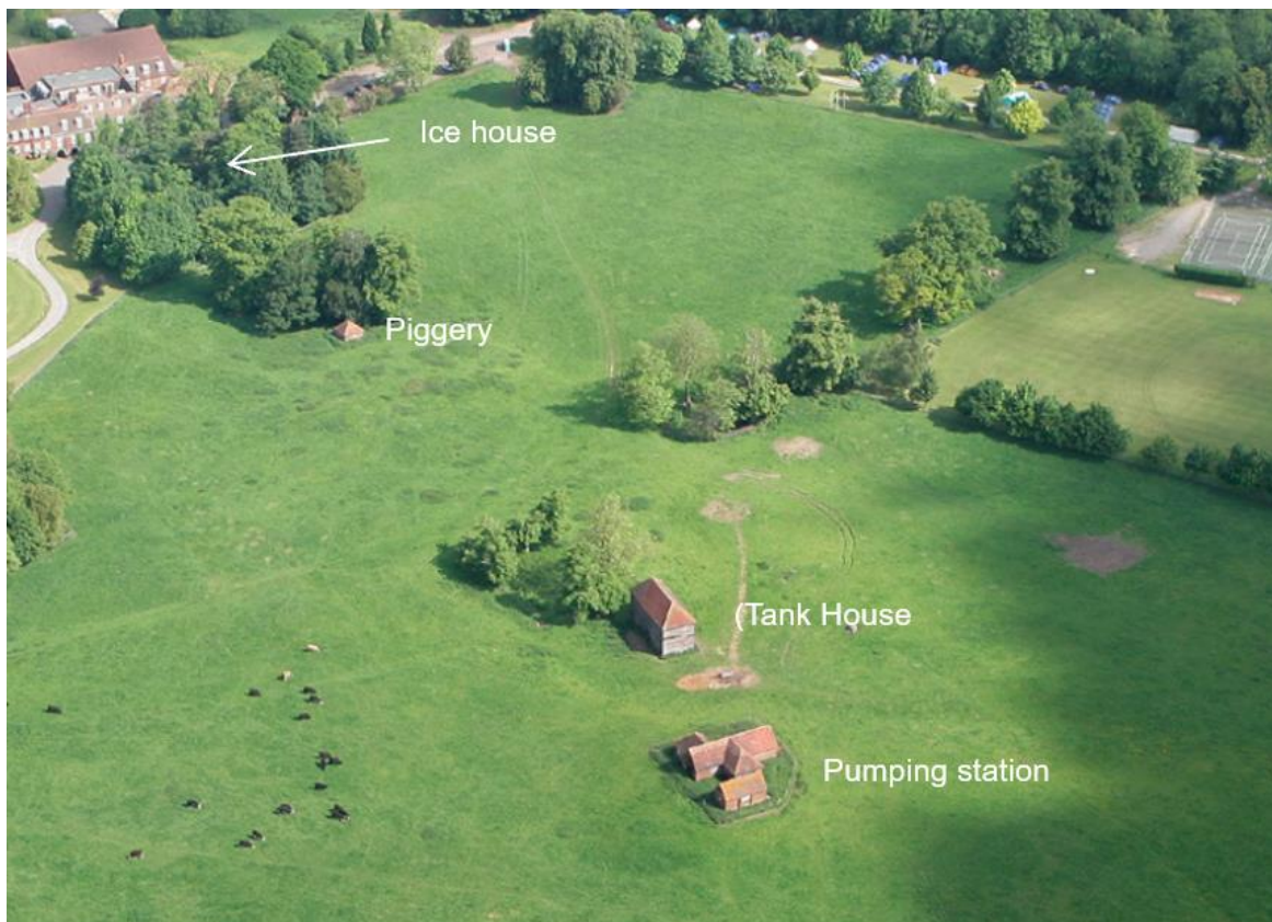
Fig. Ixxiv Surviving Park Buildings
