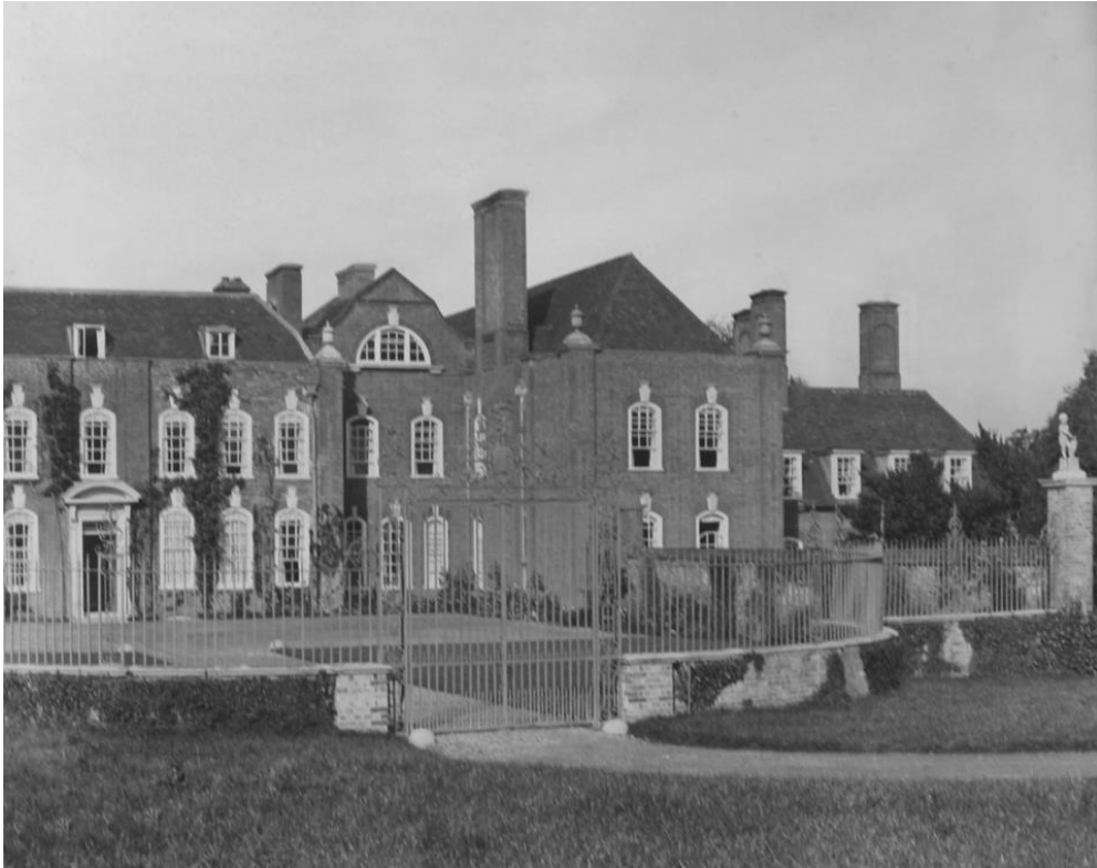
Fig. xxix South Front Old House (left), East Link, East Wing (centre) and Coach House Stable (right). This predates the additional window for the reconfiguration of the Housekeeper area. (Weaver 1913)
