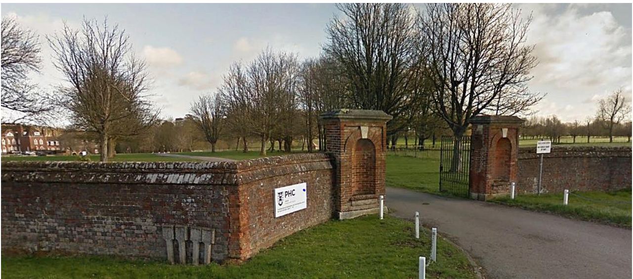
Fig. lxxx Main entrance gates, walls and piers
