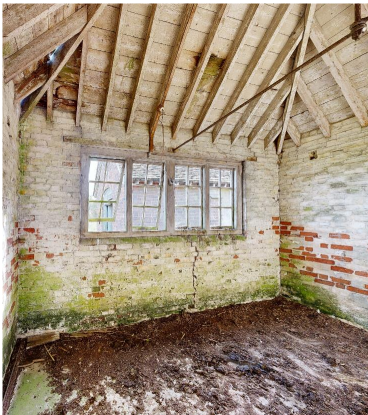
119. South wing interior
