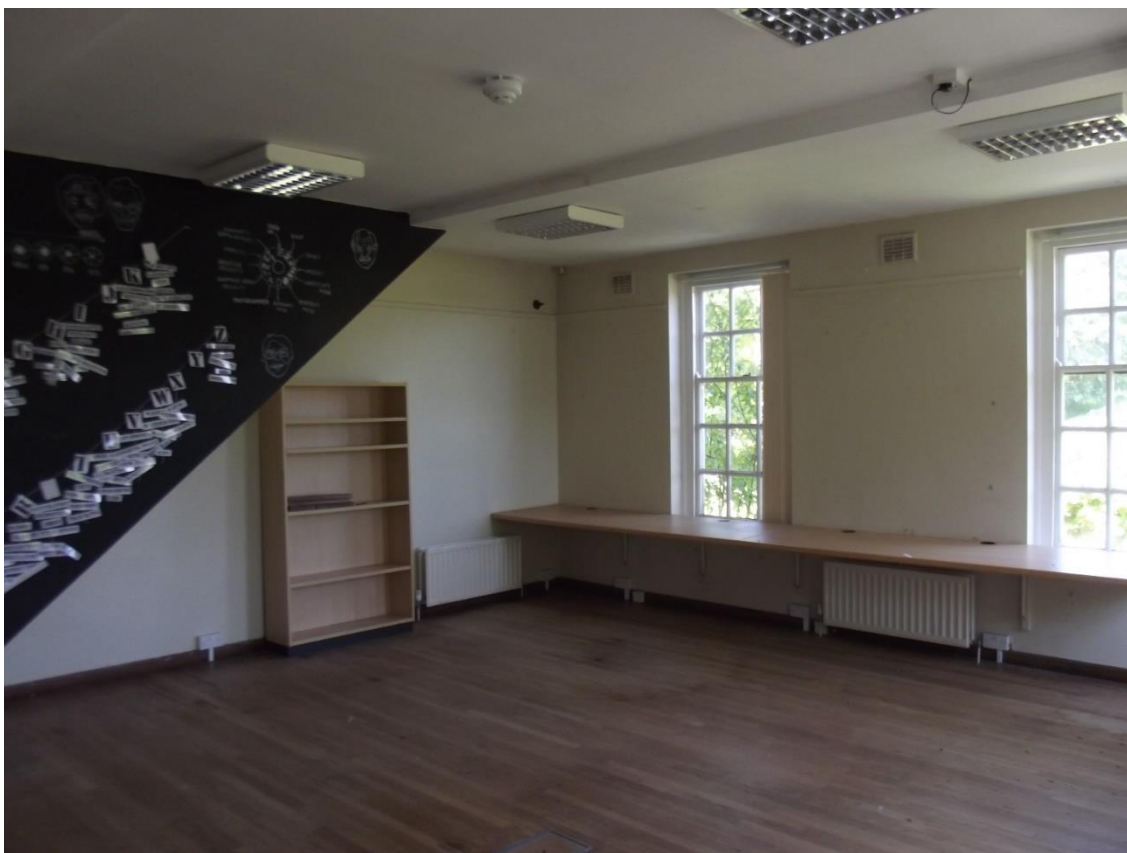
1960s extension looking west
