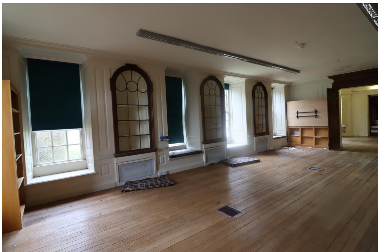
47. Drawing Room windows and cupboard on west wall
