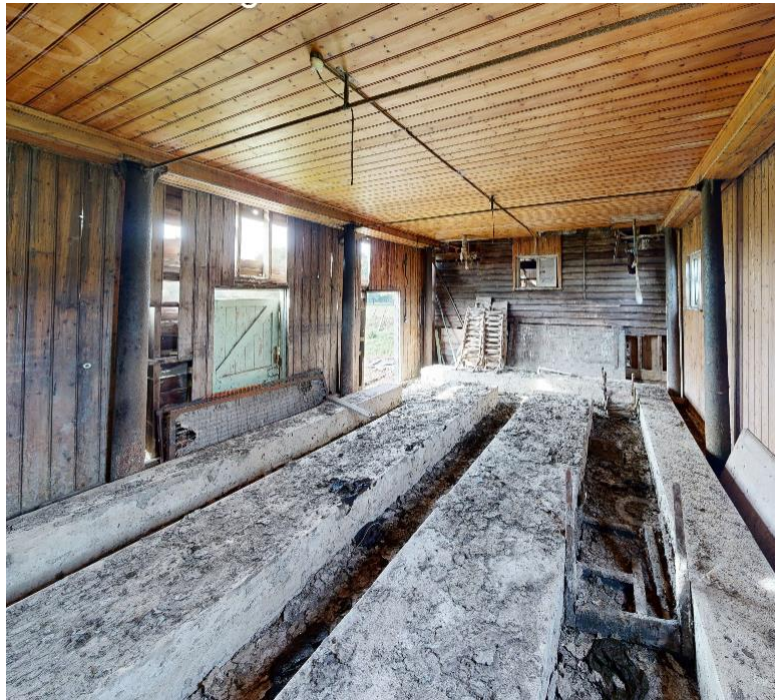
125. Tank House south section showing cast iron pillars and concrete floor supports for water tank
