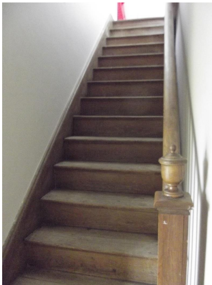
53. Stairs within the 1960s extension
