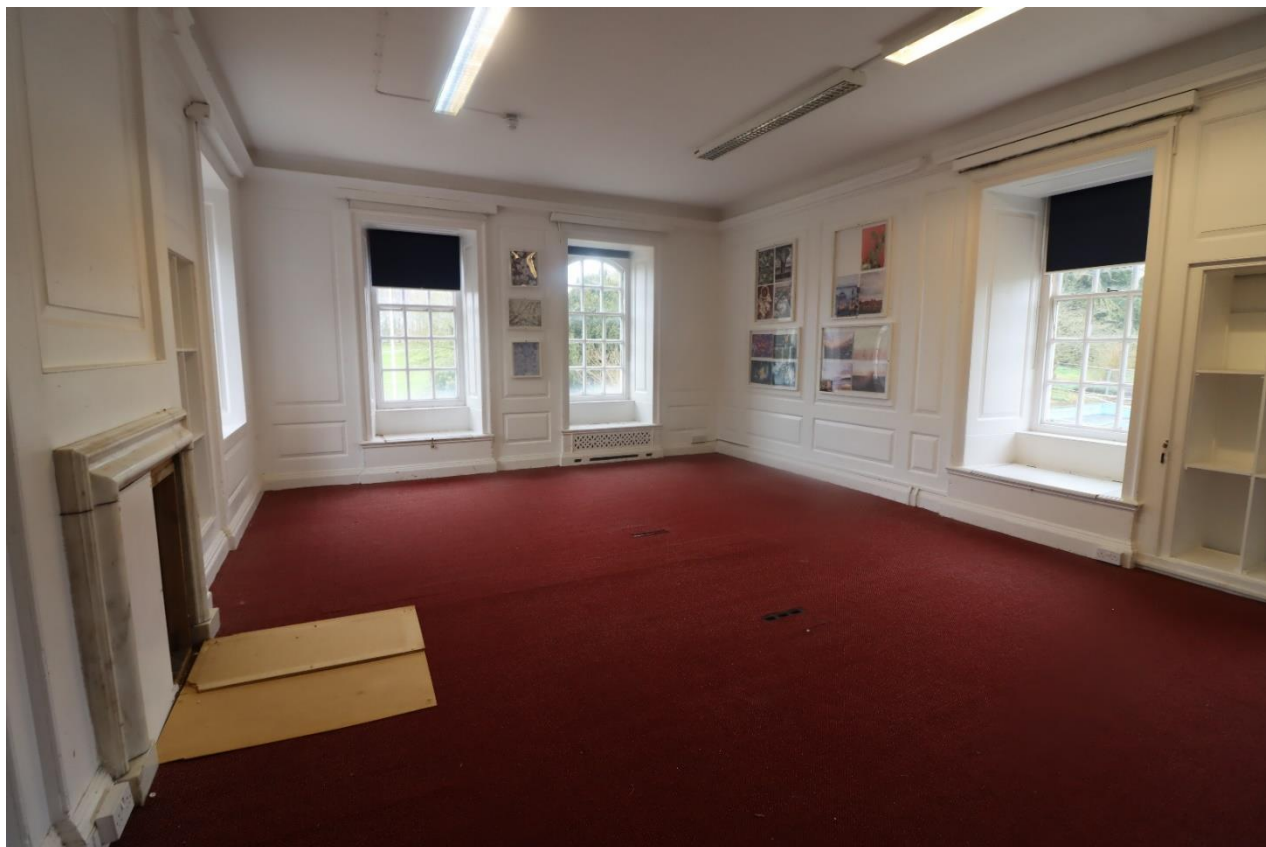
63 South end room of West Wing looking south
