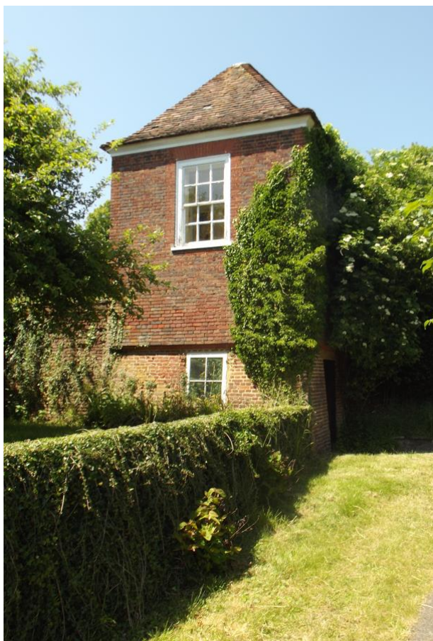
112. Belvedere from the south showing basement room
