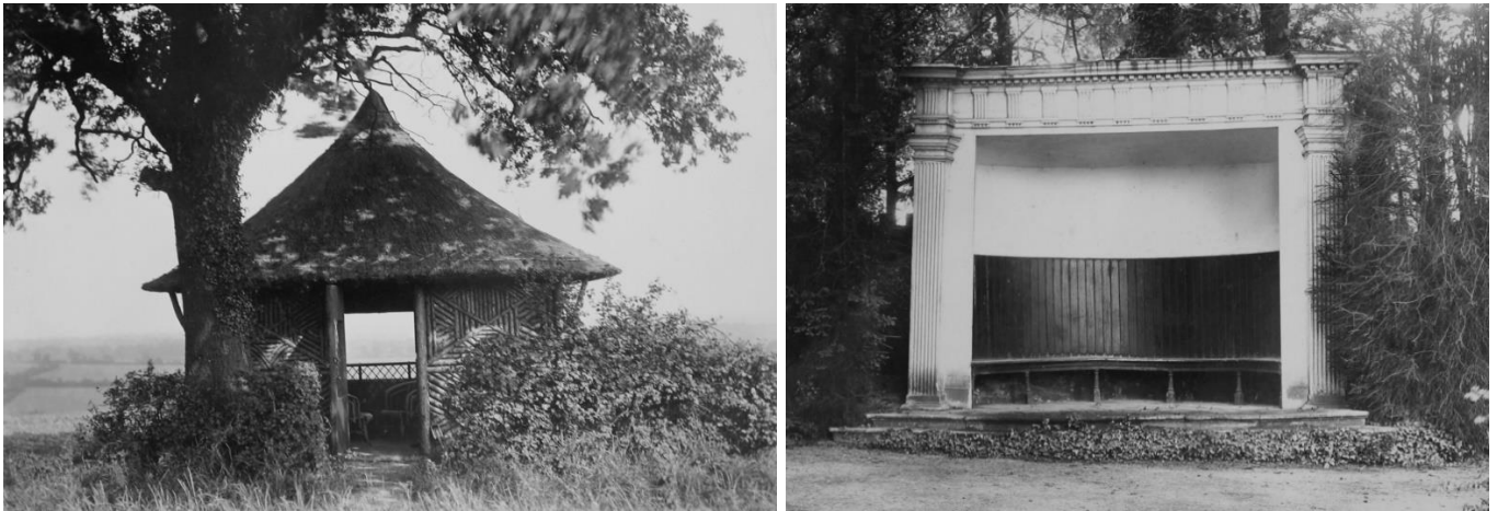
Fig. Ixxi Summer house and shelter 1913
