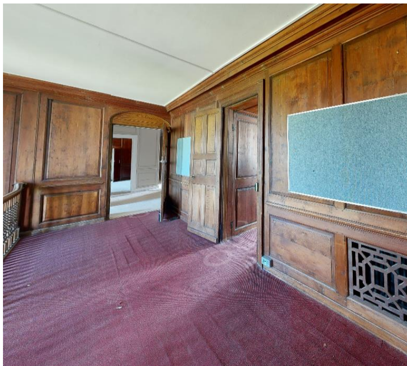
27. First floor landing
