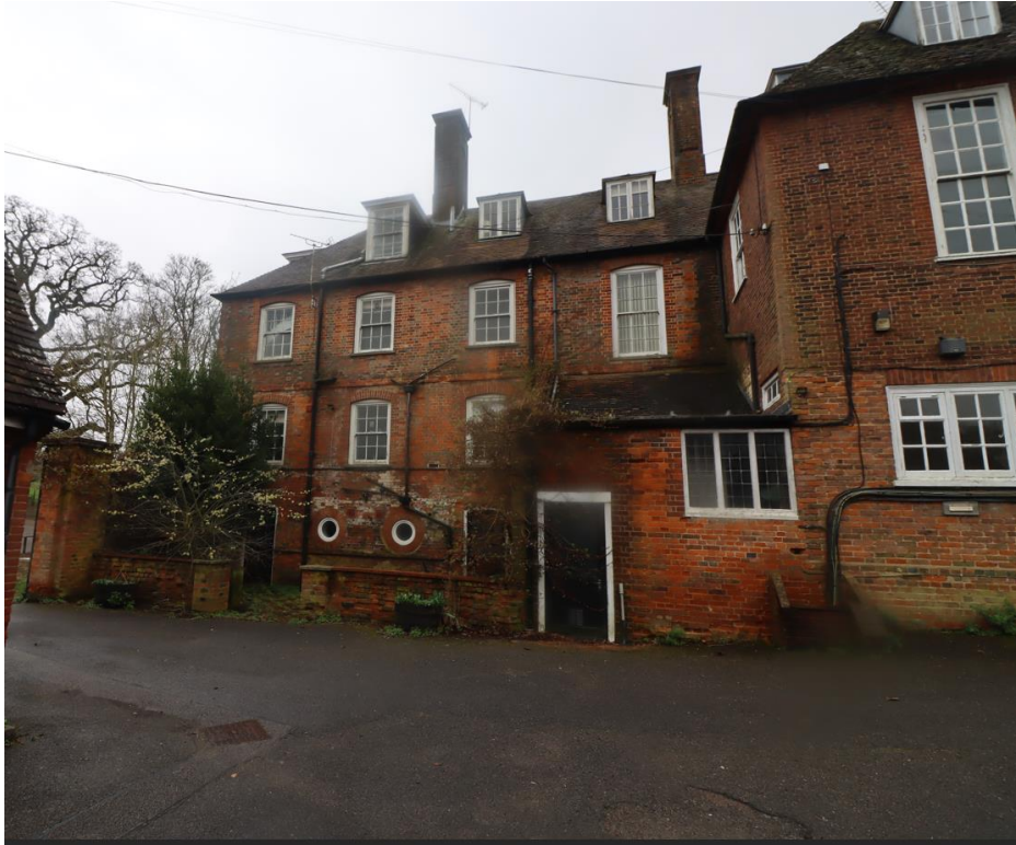
9 Rear of former stables with circular windows of the 1890s amid traces of whitewash behind a former yard wall, with a 20 th century store to the right. There is rebuilding above the string course and dormers inserted as the building became used for additional accommodation
