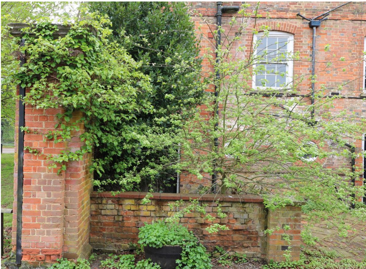
8. Gable end of former stables showing differences in brickwork and rebuilding after 1888 fire
