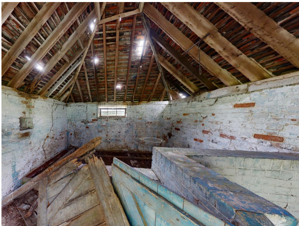
129. The Piggery interior looking east
