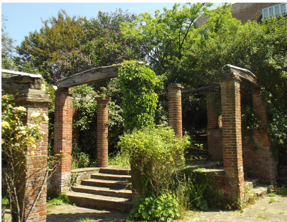
110. Pergola garden with mix of round and square columns
