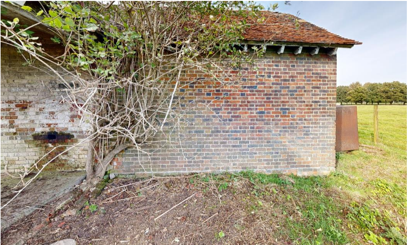
117. Pump House central section from the south
