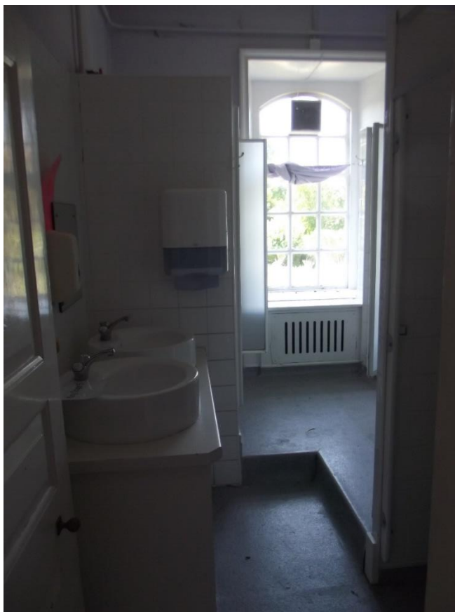
65. Inserted bathroom on first floor of link block
