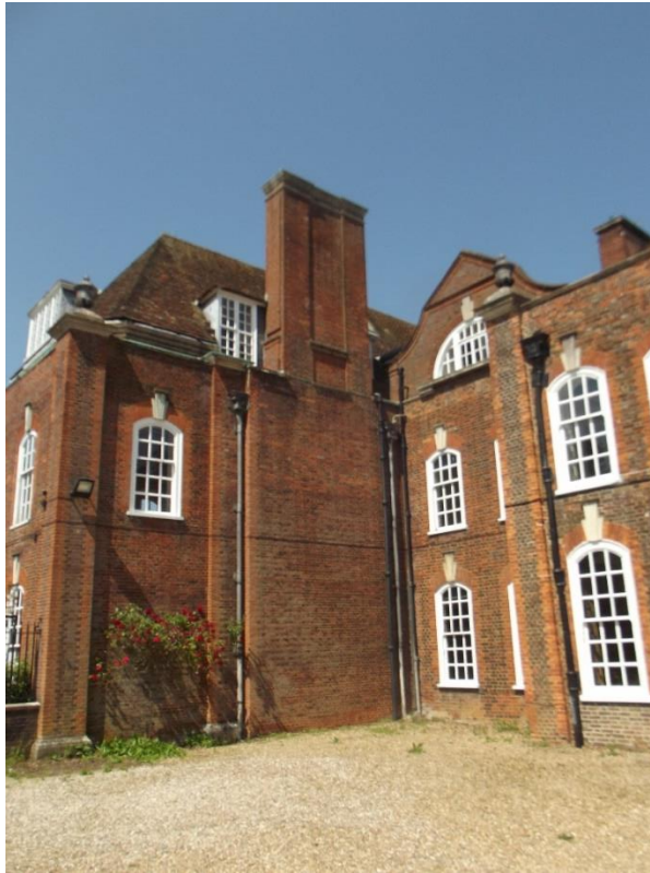
5. West wing east elevation with chimney stack
