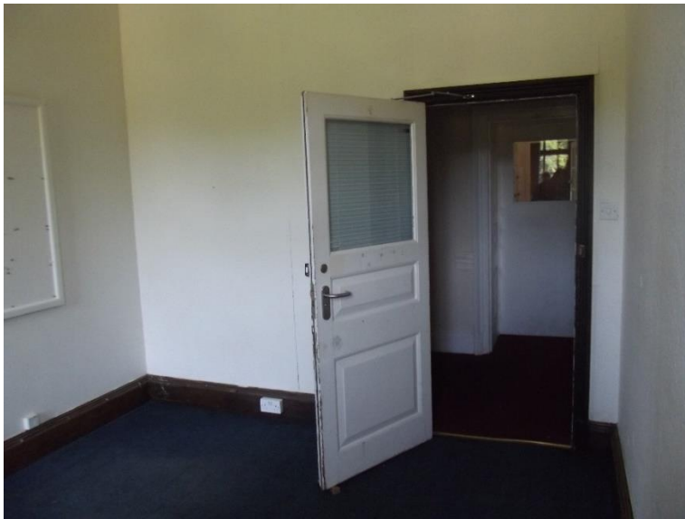
60. New room formed by subdivision
