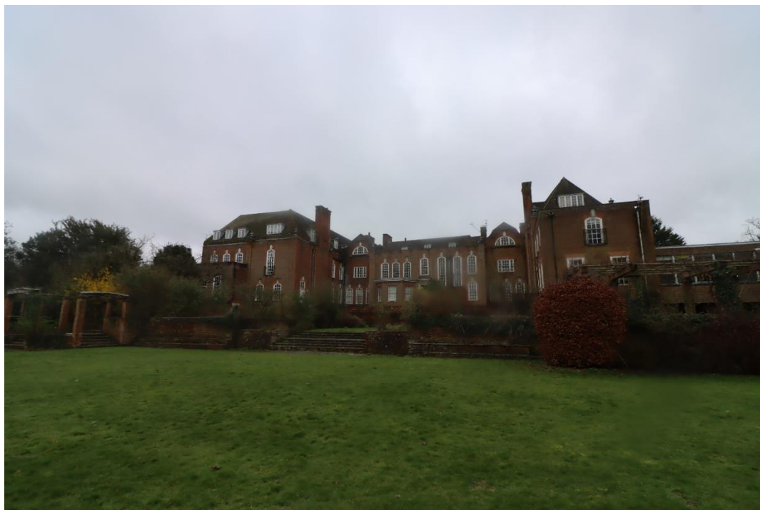
13. Rear elevation long view across the north lawn
