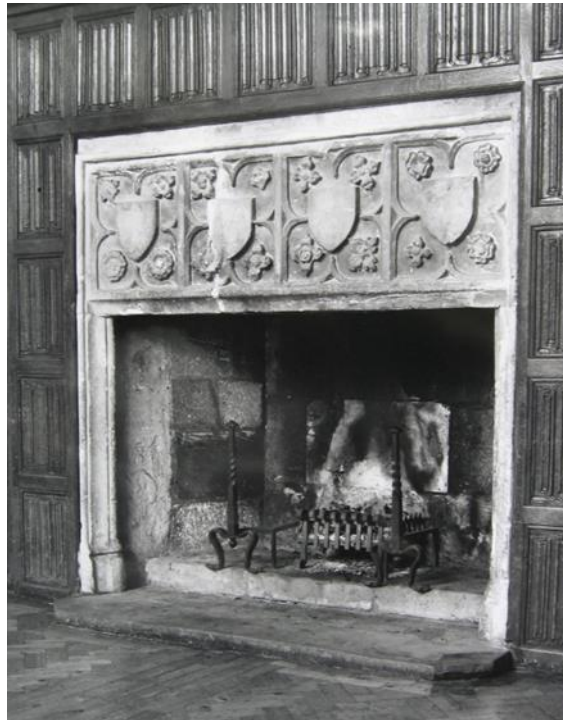
Fig. liii Fireplace within Housekeepers' area circa 1890 (The layout of this area was altered to remove partitions and open the room to a single space)
