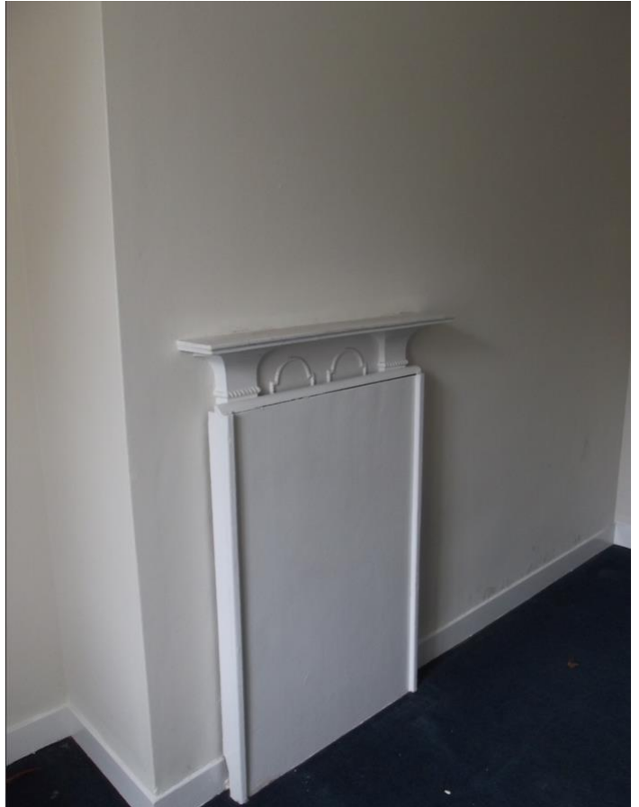
40. Second floor south side
