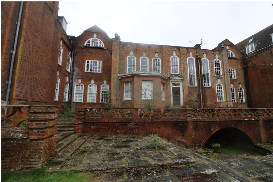
12. Rear elevation of Old House, with Lutyens east and west links and the Halseys' bay window to the dining room ca. 1840s. The wall pool and steps form part of Lutyens original north garden layout.
