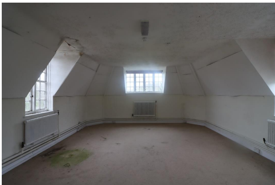
68. West Wing second floor south end room
