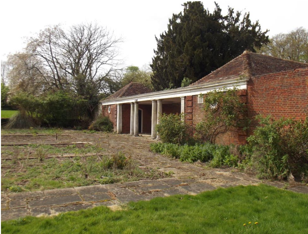
105. Pavilions and loggia
