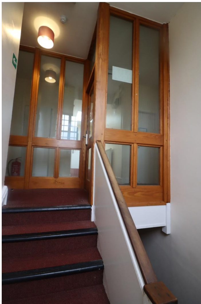
67 Second floor stair lobby
