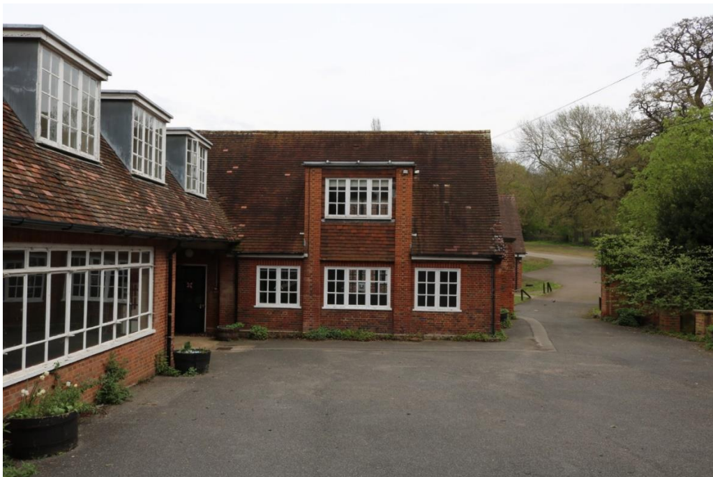
96. Teaching Block south-west side. The section on the left is of late 20 th century date, whilst the projecting wing hides the 1918-35 building
