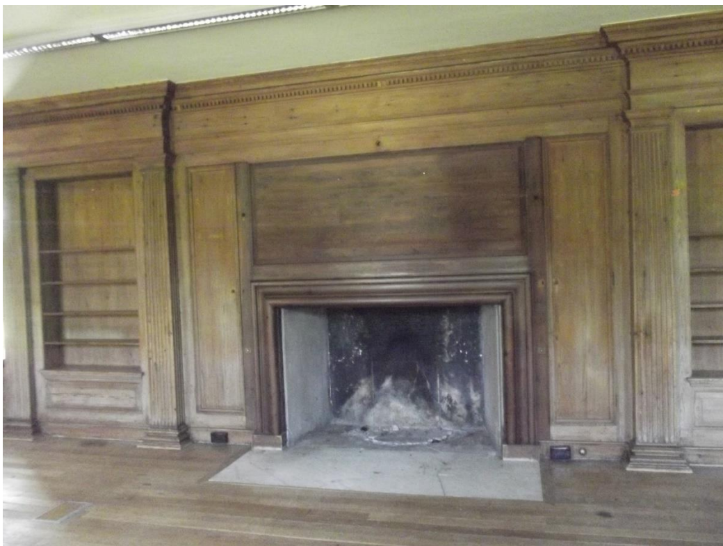
50. Smoking Room fireplace on east wall
