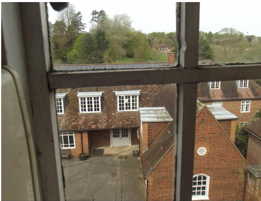
88. View from rear first floor rooms looking north to the outbuilding (now the Teaching Block)
