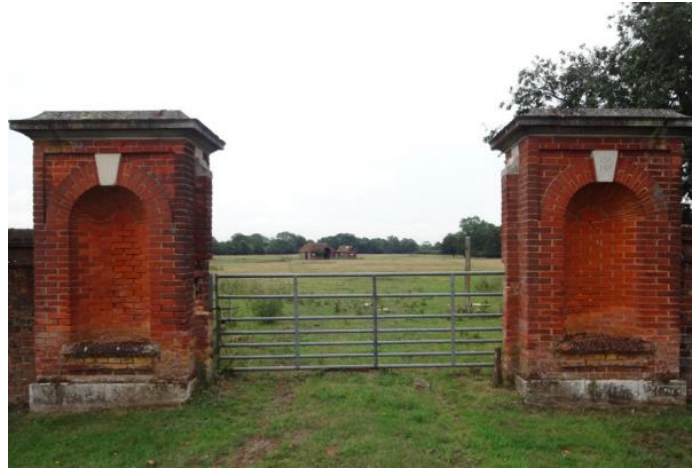
Fig. lxxxi Gates to pumping station
