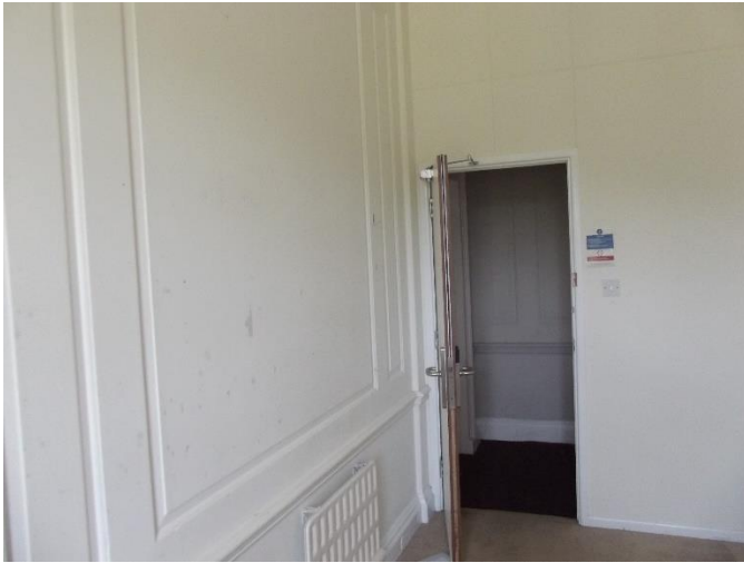
58. School rooms retaining Lutyens panelling
