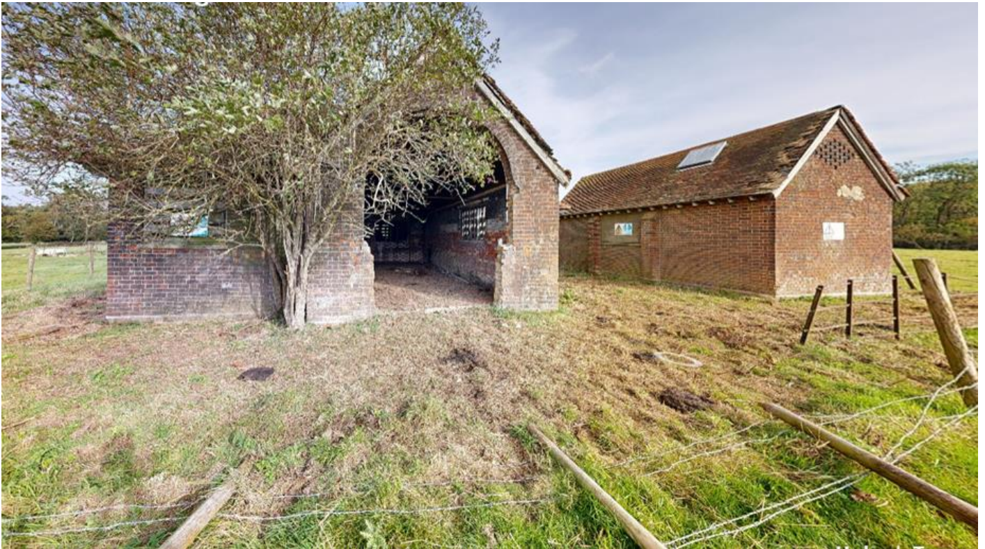
115. Pump House west elevation
