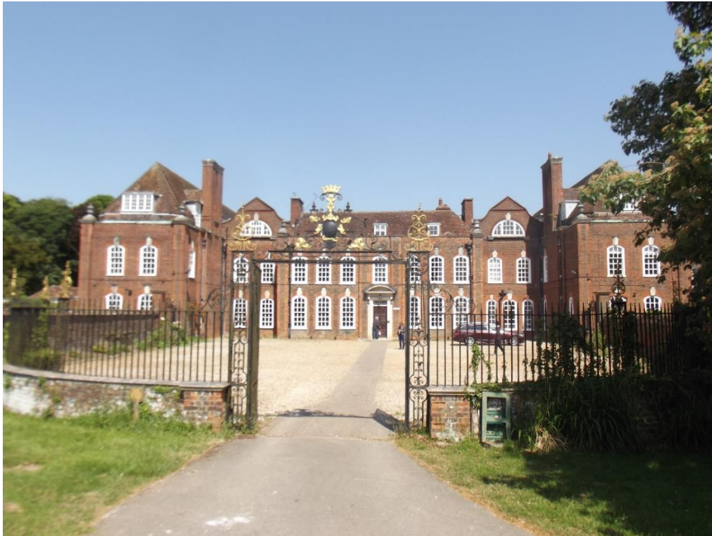
1. South elevation Old House central within front courtyard, recessed links to either side connecting to Lutyens west and east wings
