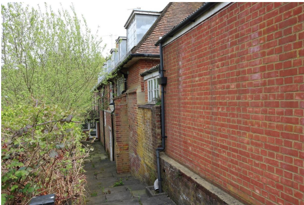
97. Teaching block west side, with earlier building to the rear and heightened in 1979
