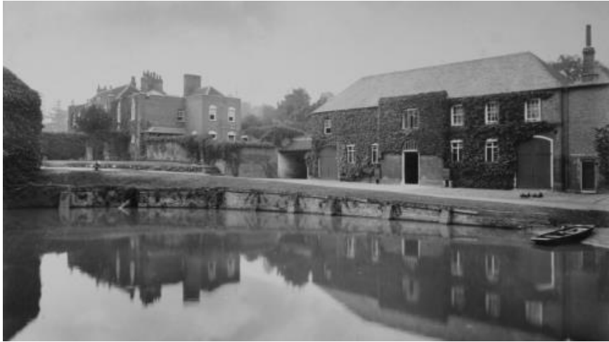
Fig. xix House and stable coach house range (right) with projecting central bay and simple roof without the clock tower, rebuilt after the fire of 1888
