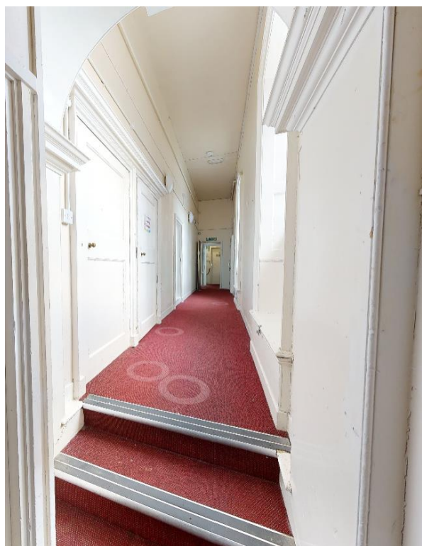
83 Corridor on north of East Wing with rooms on the left
