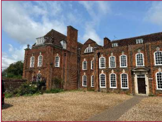
a) The main historic building at the former Princess Helena College.
