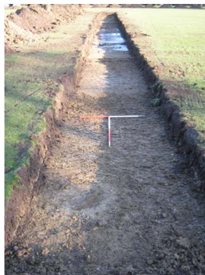
DP 26. Trench 7. Looking east.
