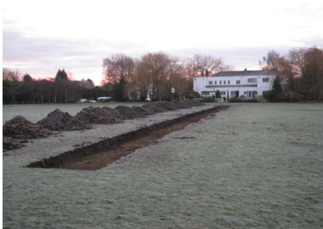
DP 1. The site. Looking south-south-east.
