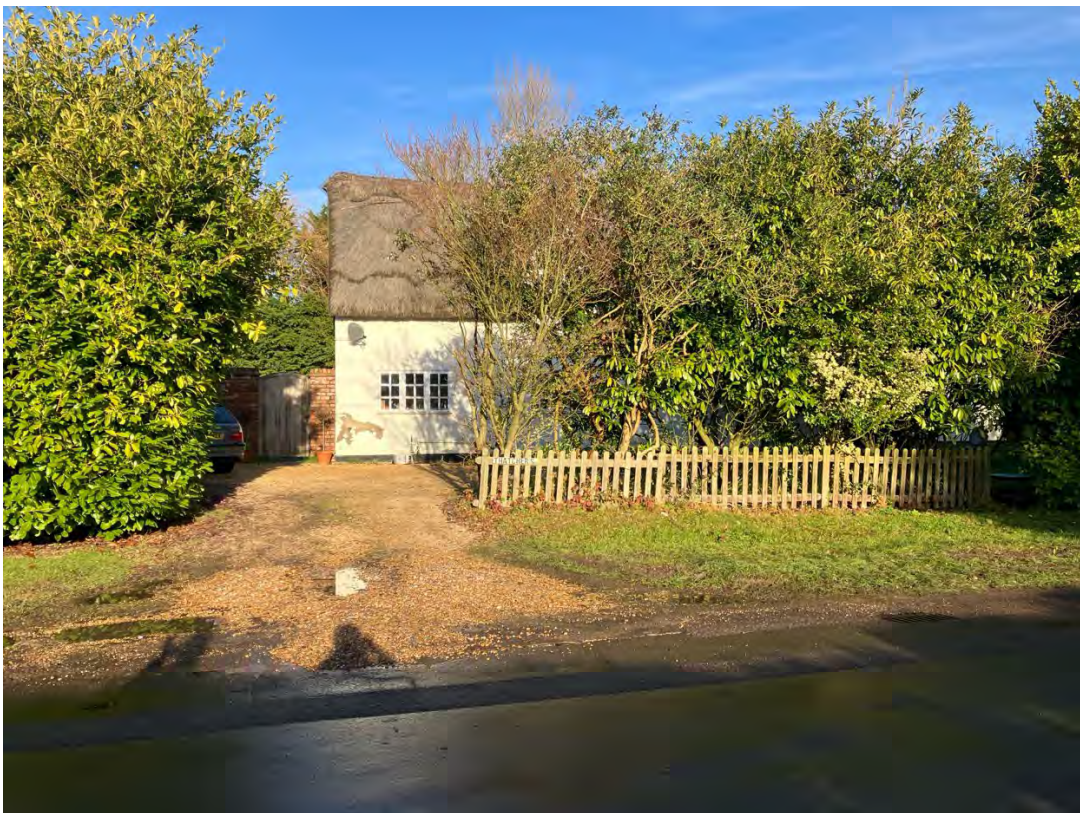
Plate 18: View of Thatchers Cottage looking north towards the study site (not visible)
