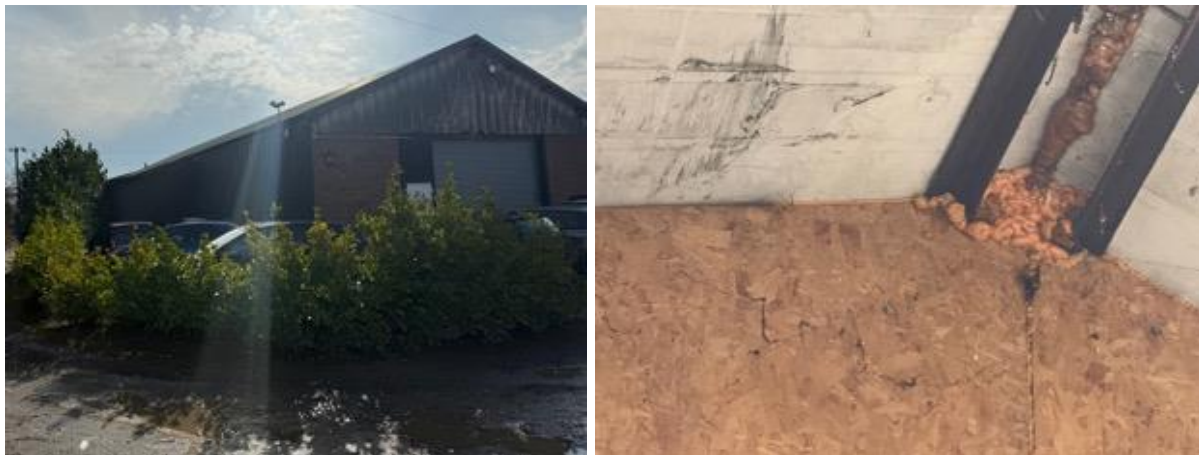
Figure 3-7 Front of Barn C showing Laurel hedge
