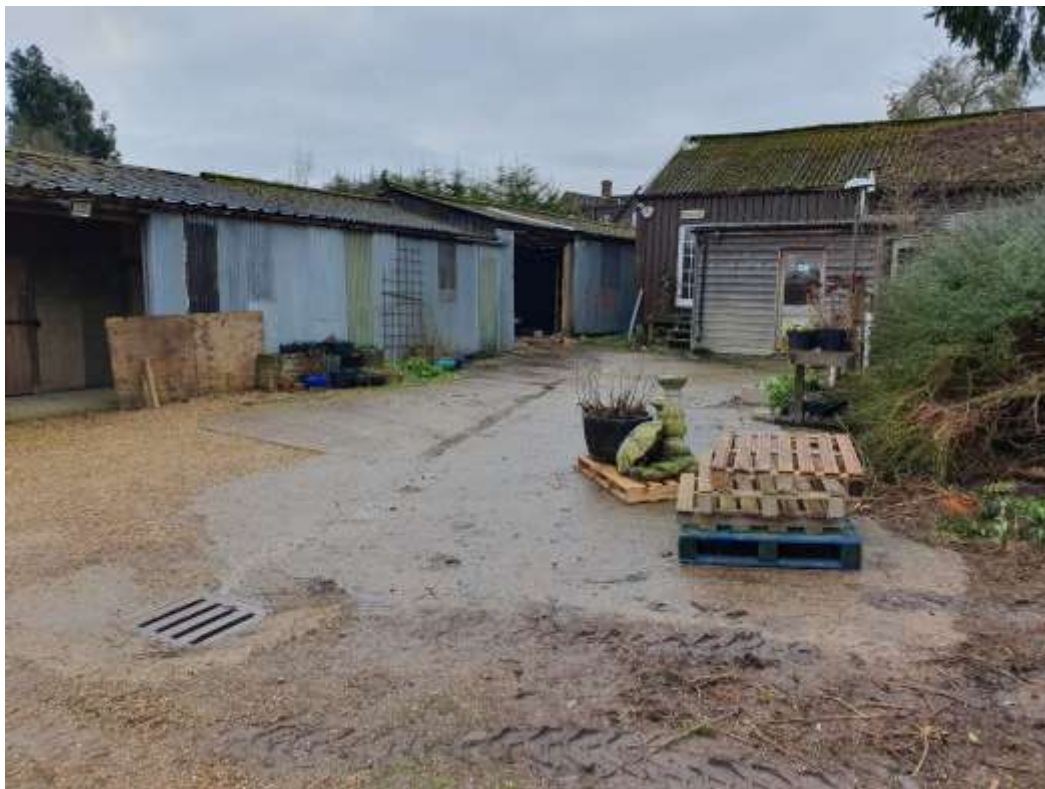
Photo 8: Builder's yard buildings and office building, facing south-west
