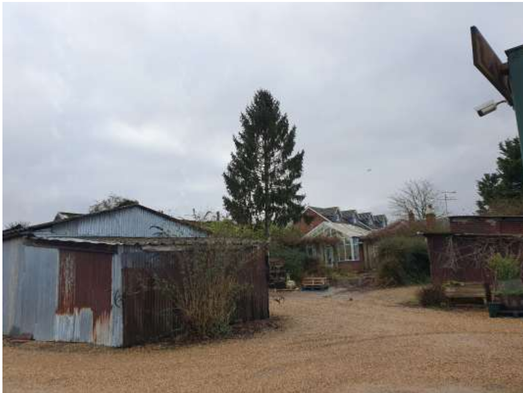
Photo 3: Existing builder's yard buildings and tree (~14m) adjacent to existing residential building.
