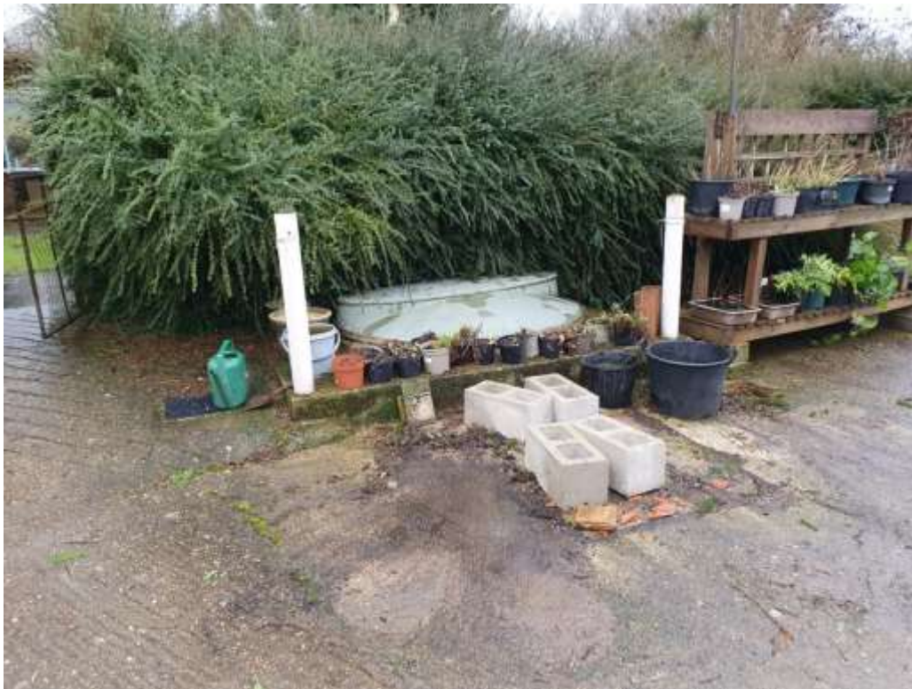
Photo 11: Septic tank located adjacent to office building in southern area of site.
