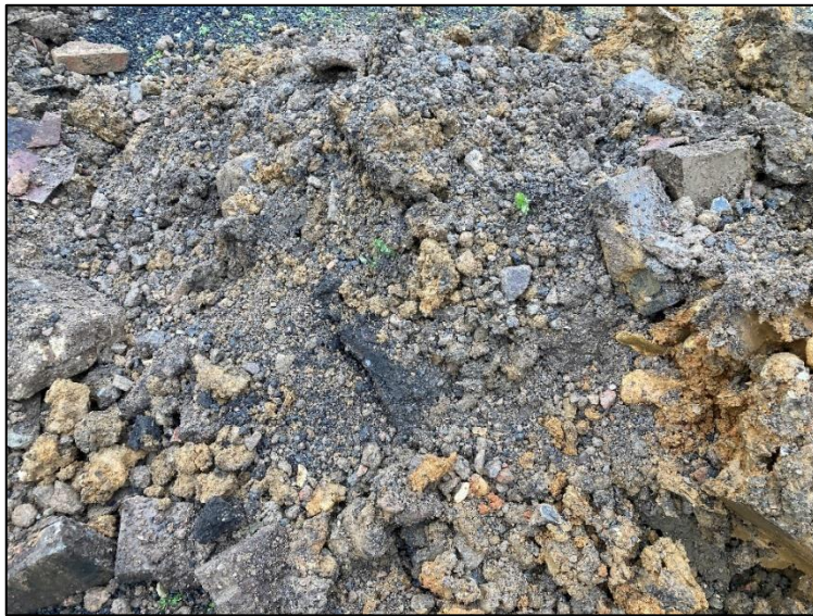
Figure 6-B: Made Ground excavated from TP02
