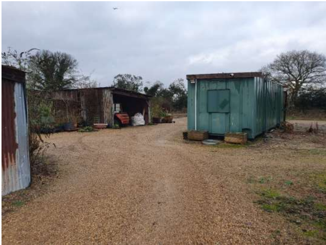
Photo 1: Existing portacabin structure and builder's yard building facing north-east.
