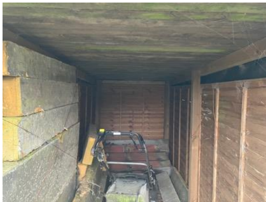
Photograph 9: B6 - tractor storage shed; timber construction with some insulative blocks
