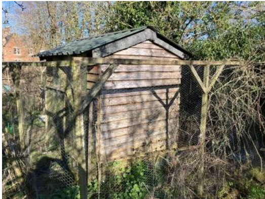
Photograph 7: B4 - timber walled, metal roofed chicken coop
