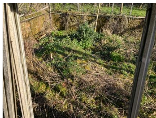
Photograph 12: Parcel PR5 - unfinished glasshouse (brick base and supports, no walls)
