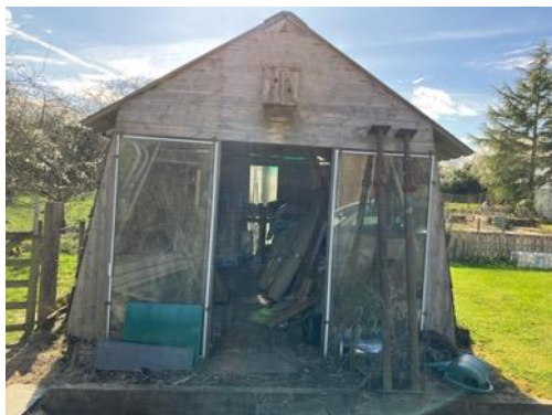
Photograph 5: B2 - storage shed
