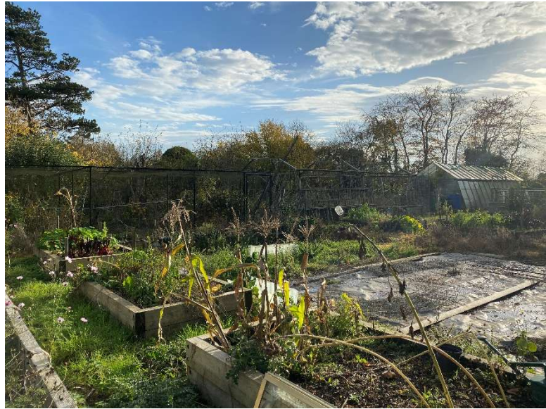
Photograph 1: View looking south east showing existing kitchen garden and derelict glasshouses to be demolished.
