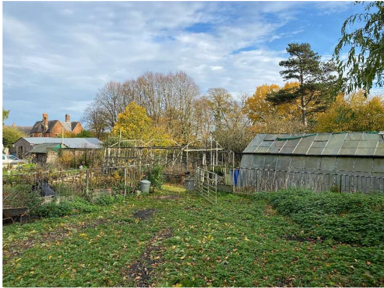
Photograph 3: View looking north east showing workshop, store shed and derelict glasshouses to be demolished.
