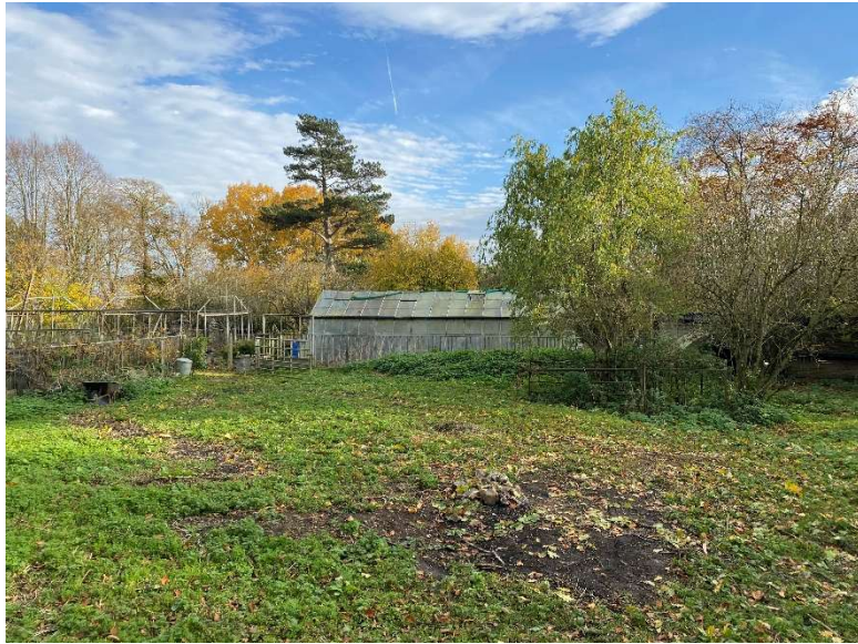
Photograph 5: View looking east showing existing glasshouse to be demolished.
