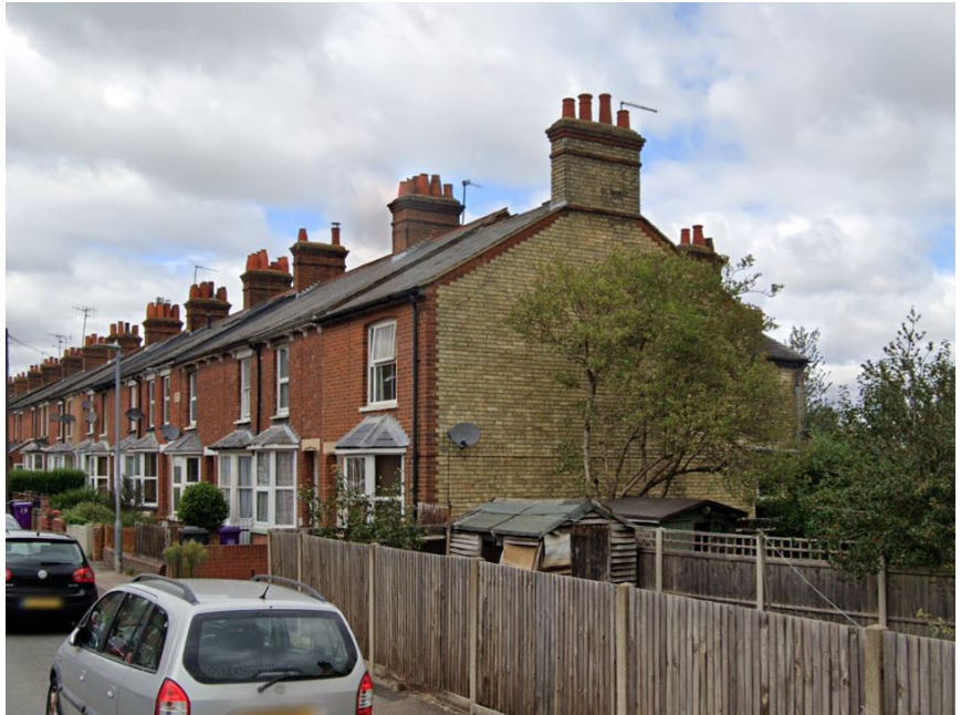
View of current end of terrace gable from Balmoral Road of no. 84 in the foreground and the rest of the terrace stretching away to the left
