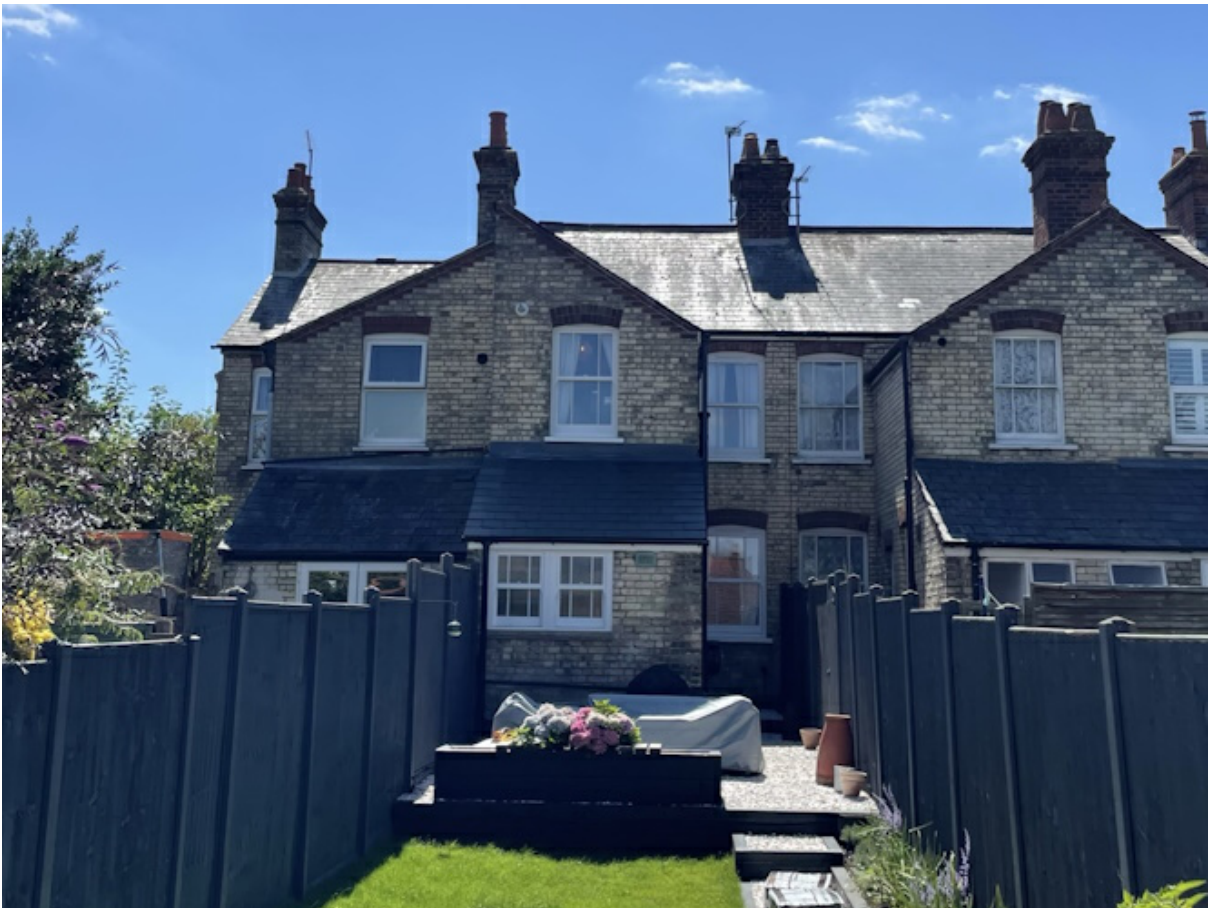
Rear view of no. 83 Balmoral Road from the rear garden with no. 84 on the left and no. 82 on the right
