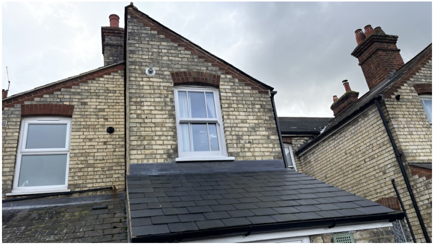
Close up rear view of no. 83 Balmoral Road from the rear garden with no. 84 on the left and no. 82 on the right
