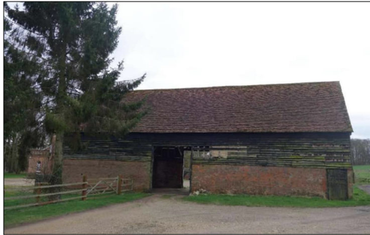
Plate 51: View looking S showing N-facing elevation of Grade II listed Barn
