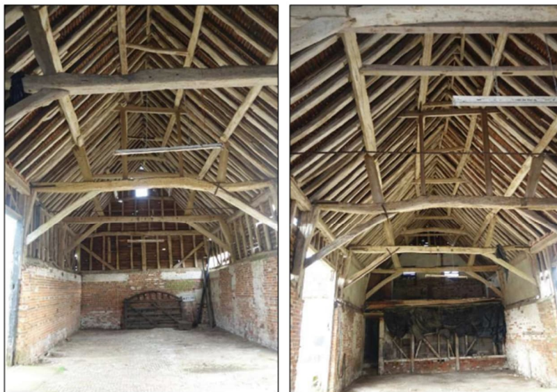
Plate 55: View looking E showing central and E portion of Barn with queenpost roof structure
