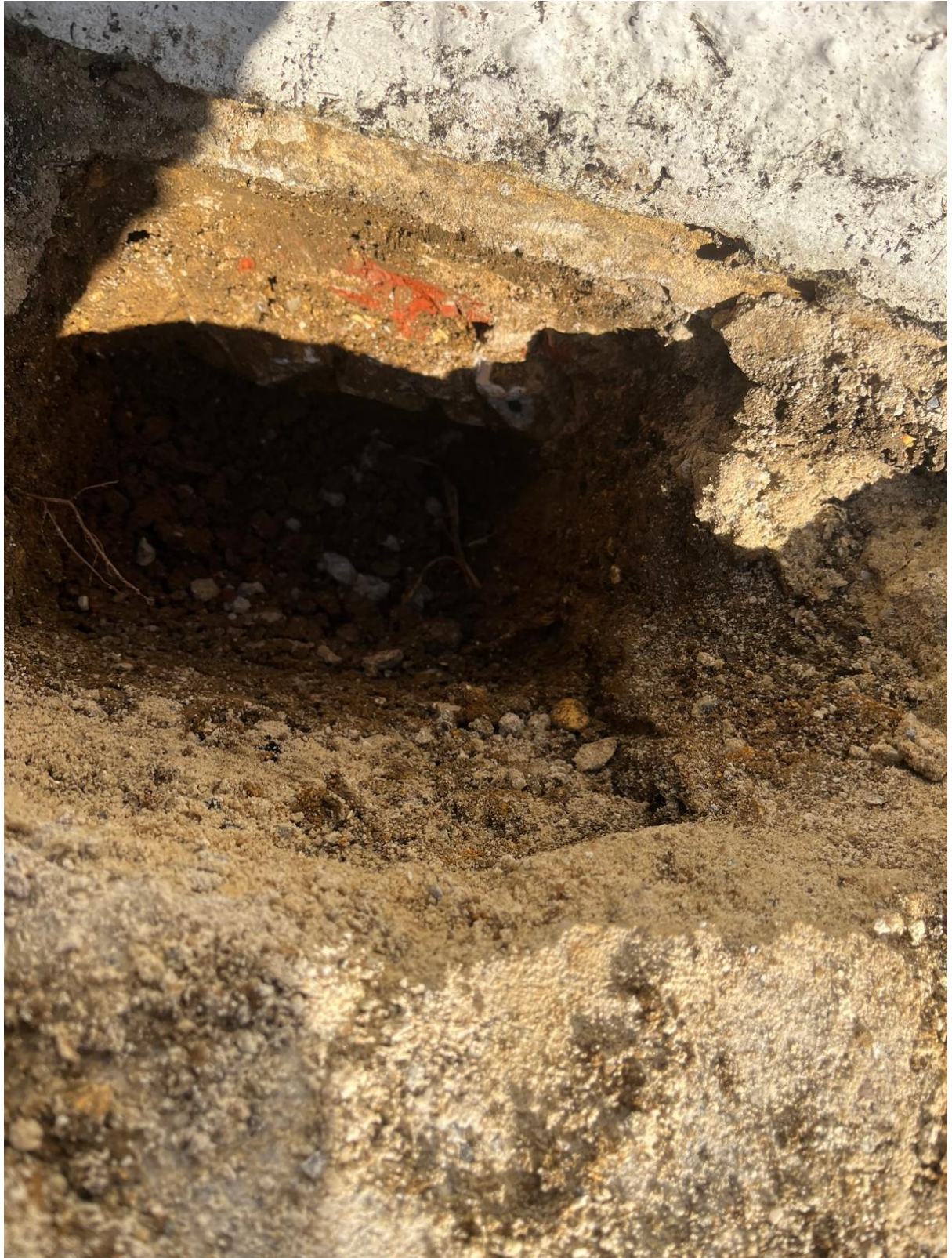
Figure 2 - Trial Pit showing no foundation
