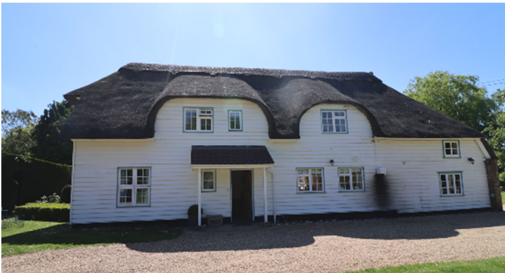
Image 10: Side North-West Elevation
