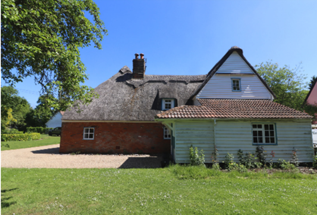
Image 9: Front South –West (Road facing) Elevation
