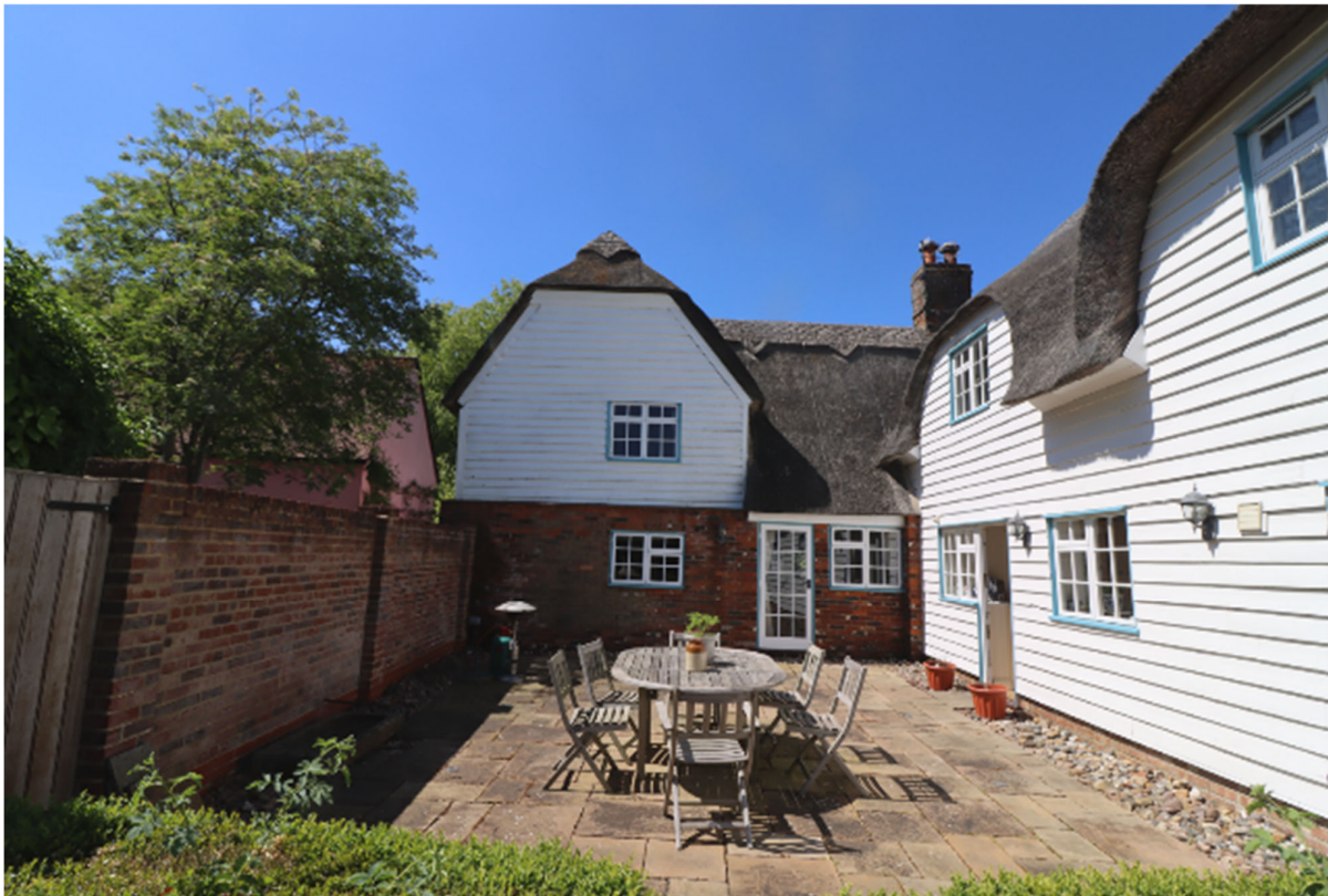
Image 12: Rear North-East elevation of old range - S.E. to the right.
