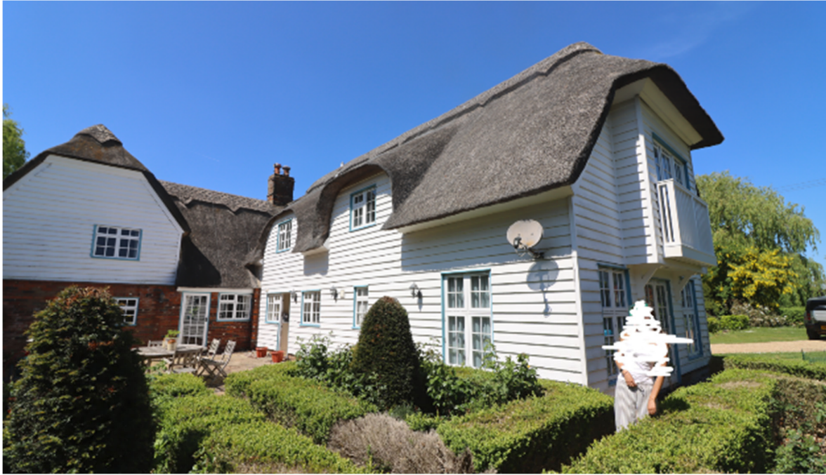
Image 11: Rear North-East elevation & Side South-East Elevation
