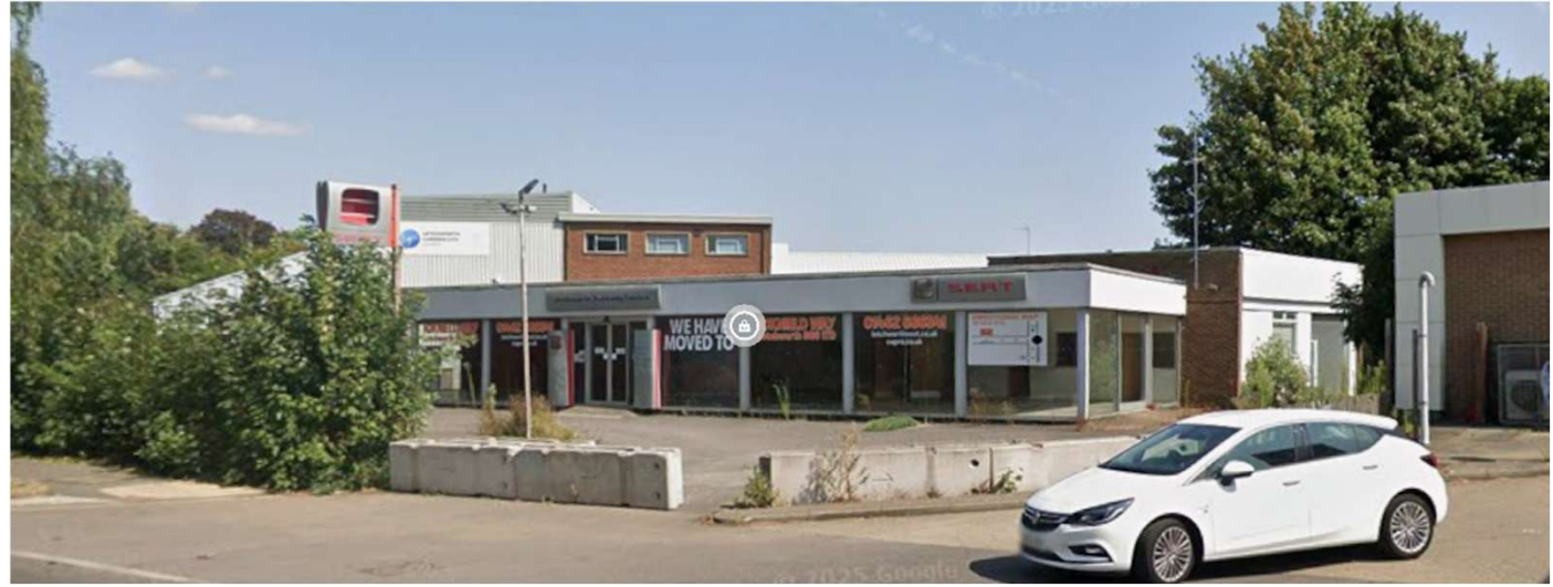
The existing showroom building, viewed from the site entrance
