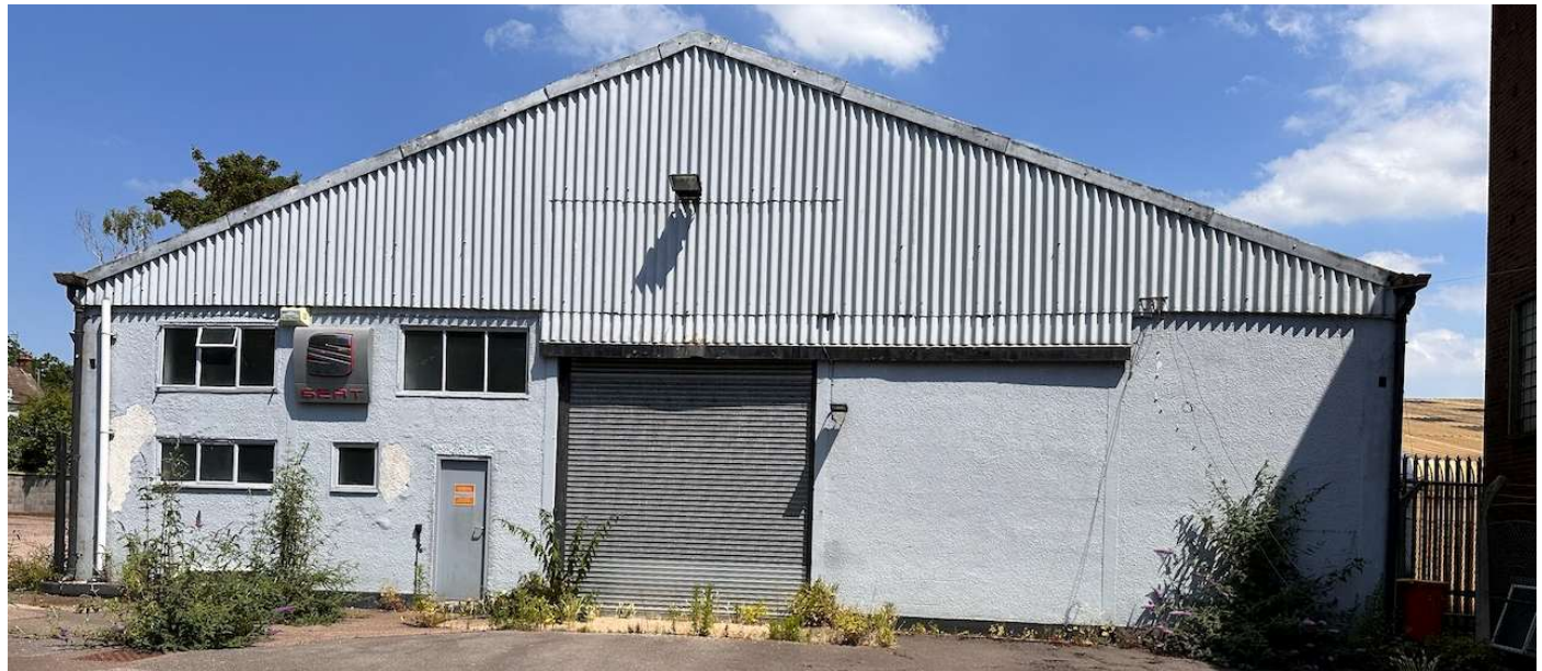
The existing west façade of the workshop
