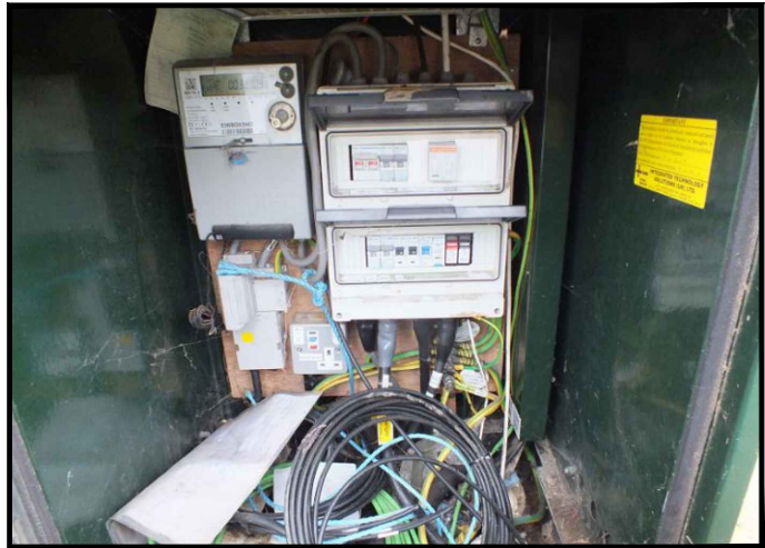
EXISTING THREE PHASE 100A REC SUPPLY
