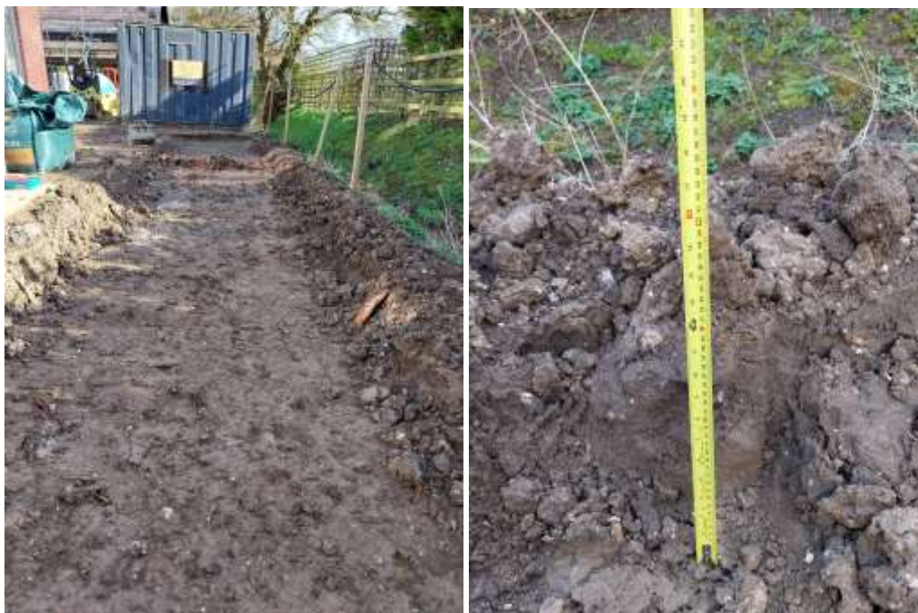
PHOTOGRAPHS 4 & 5 – FURTHER REDUCED DIG OF CELL 2
