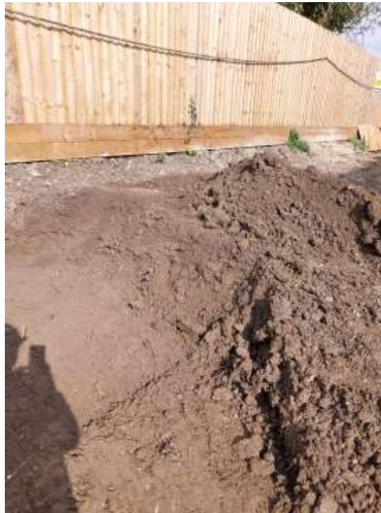
PHOTOGRAPH 7 – FURTHER EXCAVATION IN THE AREA OF SAMPLE 1 IN CELL 4
