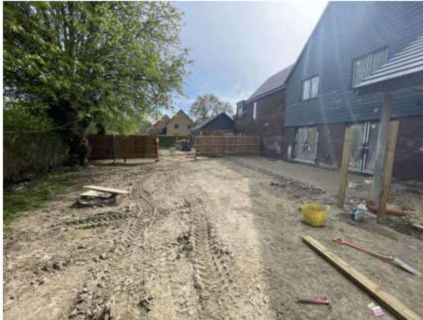
PHOTOGRAPH 13 – CELL 5 EXCAVATED DOWN TO NATURAL SOILS (LOOKING SOUTH)
