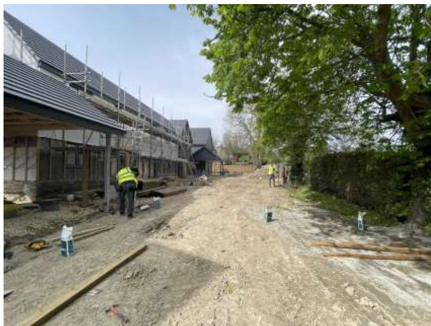
PHOTOGRAPH 12 – CELL 5 EXCAVATED DOWN TO NATURAL SOILS (LOOKING NORTH)
