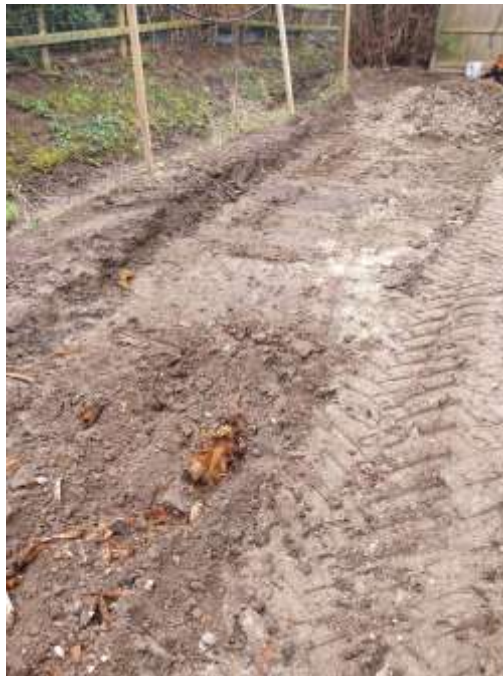
PHOTOGRAPH 3 - CELL 2 EXCAVATION – JANUARY 2024
