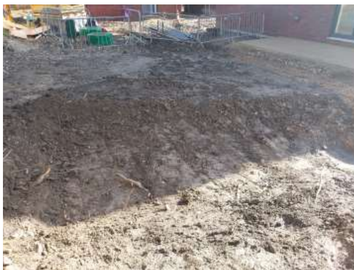
PHOTOGRAPH 6 – FURTHER REDUCED DIG OF CELL 4
