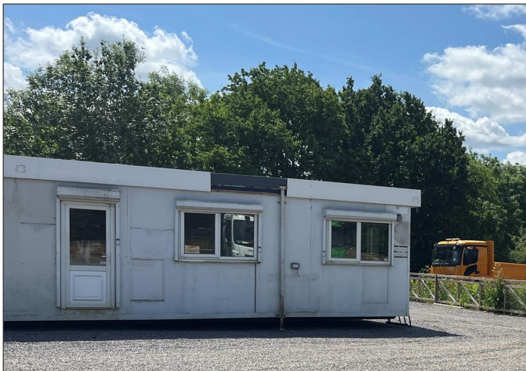
Figure 6: Building B1 located towards north-east of site.
