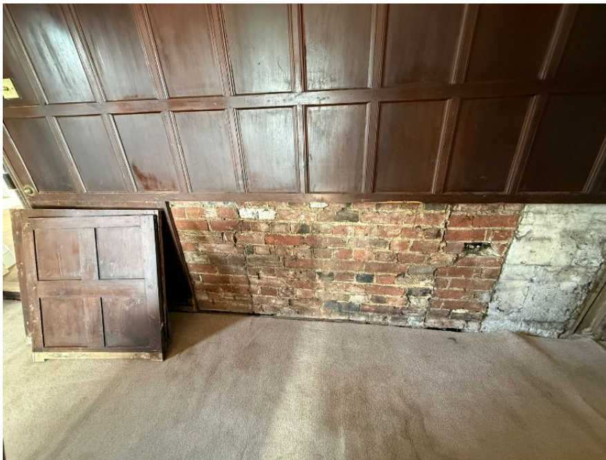
North wall of Living Room with modern panelling carefully removed. Evidence of historic hearth with brick infill. NB infill appears to be 'floating' with no clear structure below.
