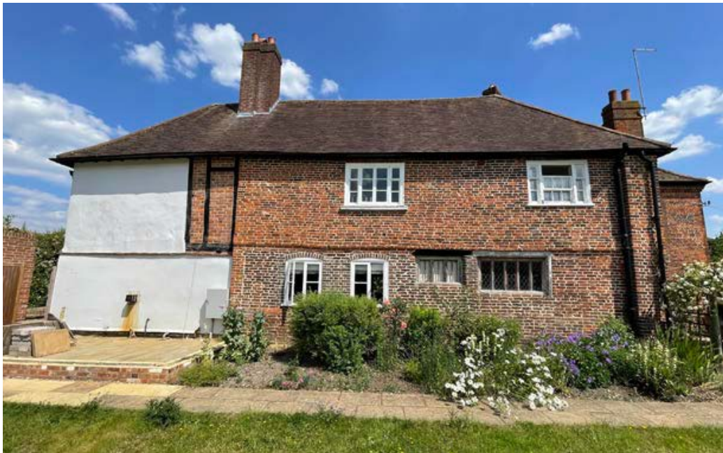
West Façade of the north range.
