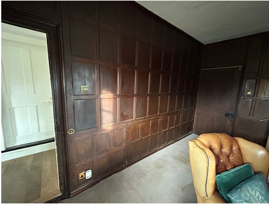
North wall of Living Room
