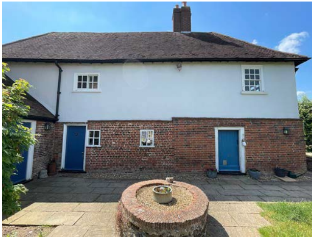
East façade of the north range
