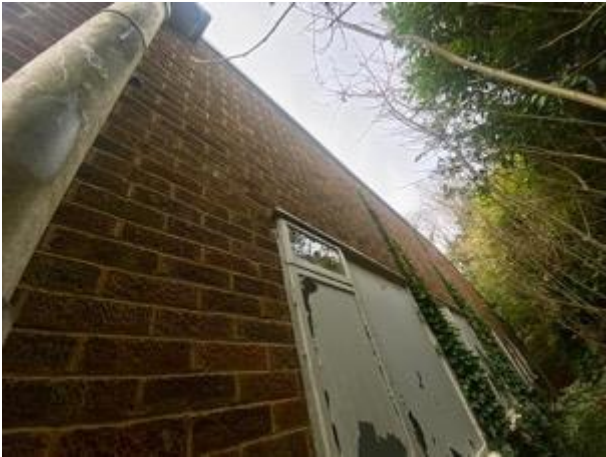
Photo 3. B1's E elevation.
