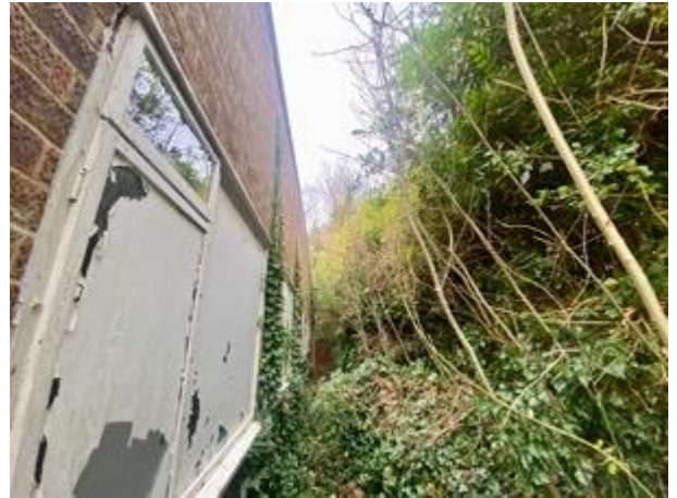
Photo 10. Eastern end of Site.
