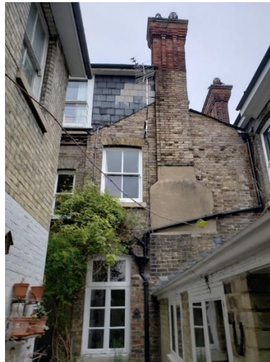
Lean-to and rear wall of no 44
