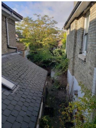
Lean-to from above
