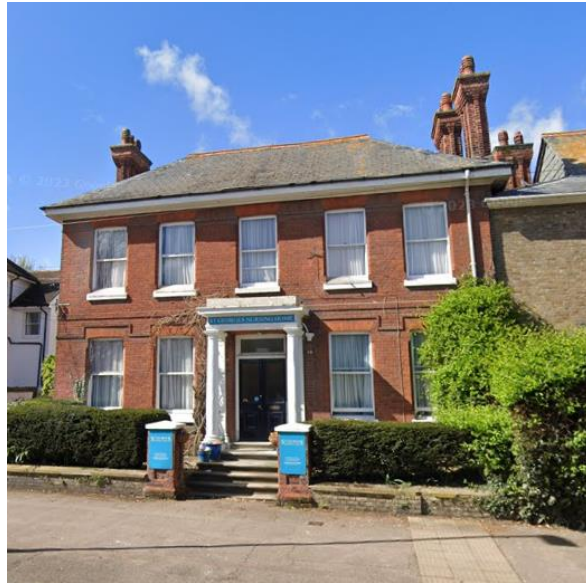
No 42 front elevation, east facing
