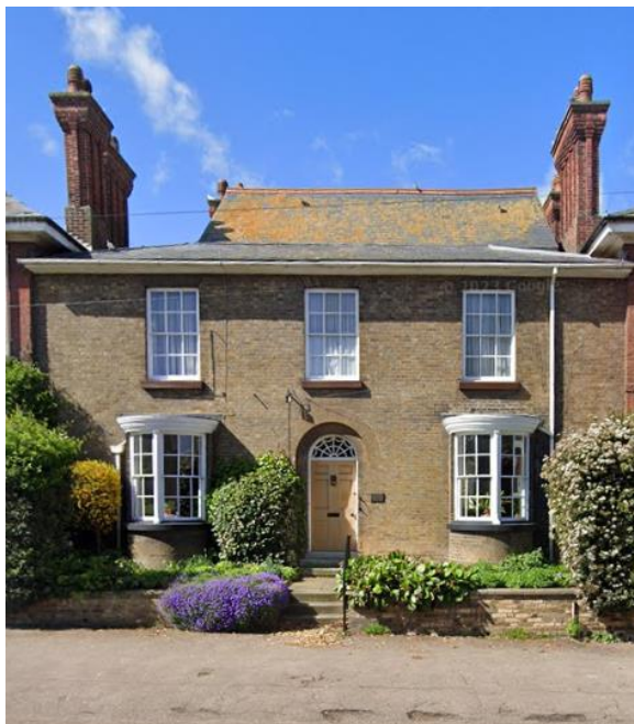
No 44, front elevation, east facing
