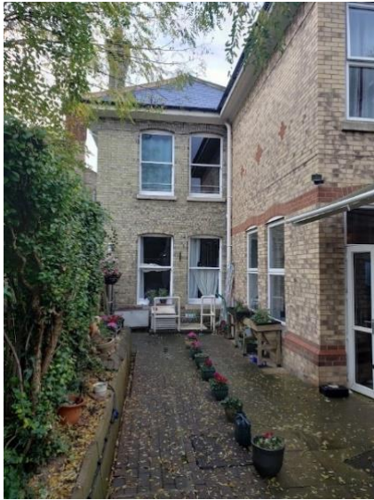
Side of extension, no 42: Looking towards house
