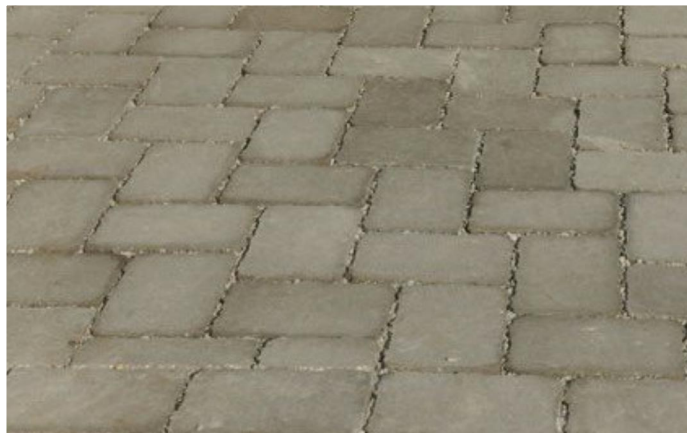
Hydropave Tobermore Tegula 240 x160 x 80mm in Slate colour in herringbone pattern to courtyard areas
