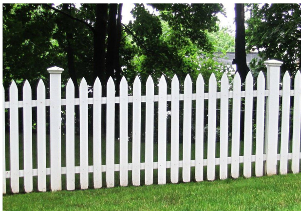
Timber Picket Fencing 900mm high (painted white).
