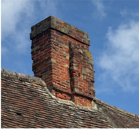
Fig 2: Detail of the Chimney Stack from the South
