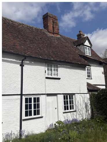
Fig 1: General view of the Chimney Stack from the front garden of 41 High Street looking South, 45 High Street to the right
