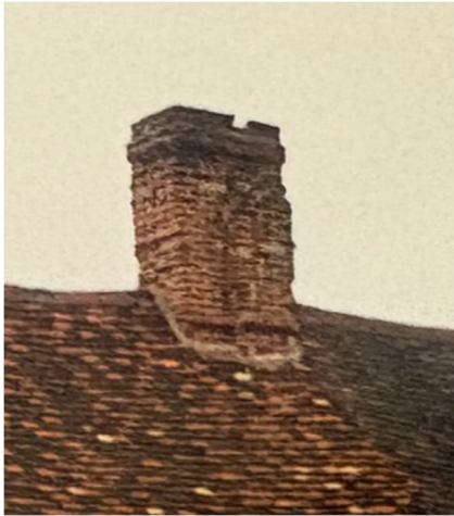
Fig 4: Detail of the chimney stack from the South taken (we estimate) in the 1970s before earlier repairs
