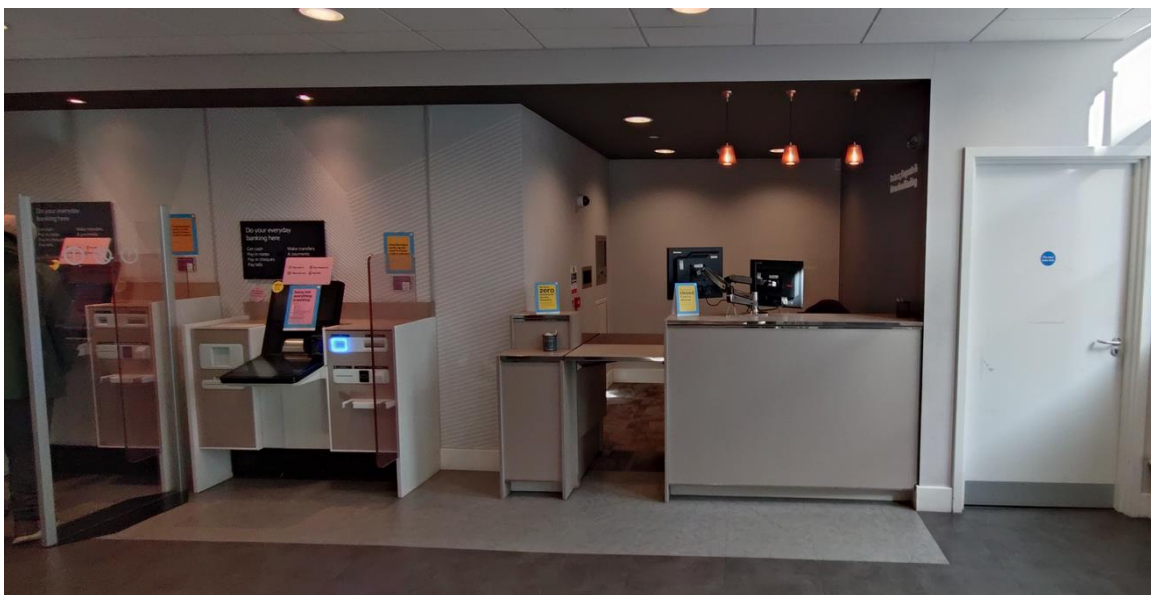
Image includes example of an Assisted Counter position – to be removed (3no.) and replaced with 3no. ATMs.
