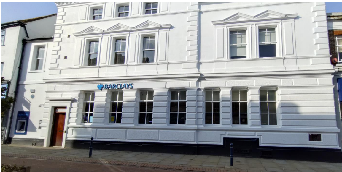
External Elevation – no planned works
