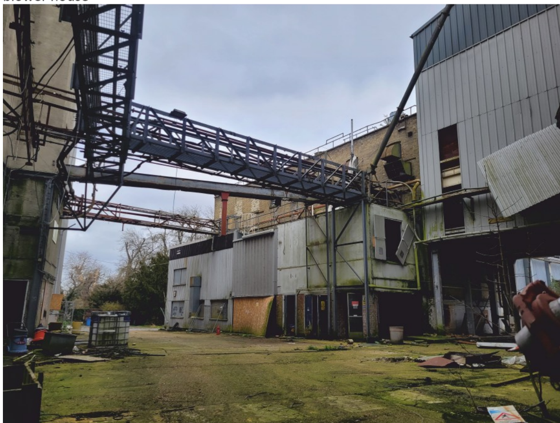
Pl. 16 North and west elevations of the roller mill looking south-east
