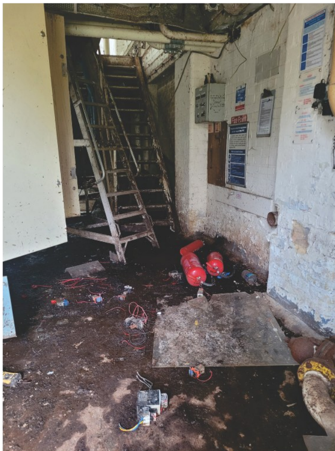
Pl. 28 Inside the east entrance to the mill, stair access to first floor, looking west 2026 (N. Field)
