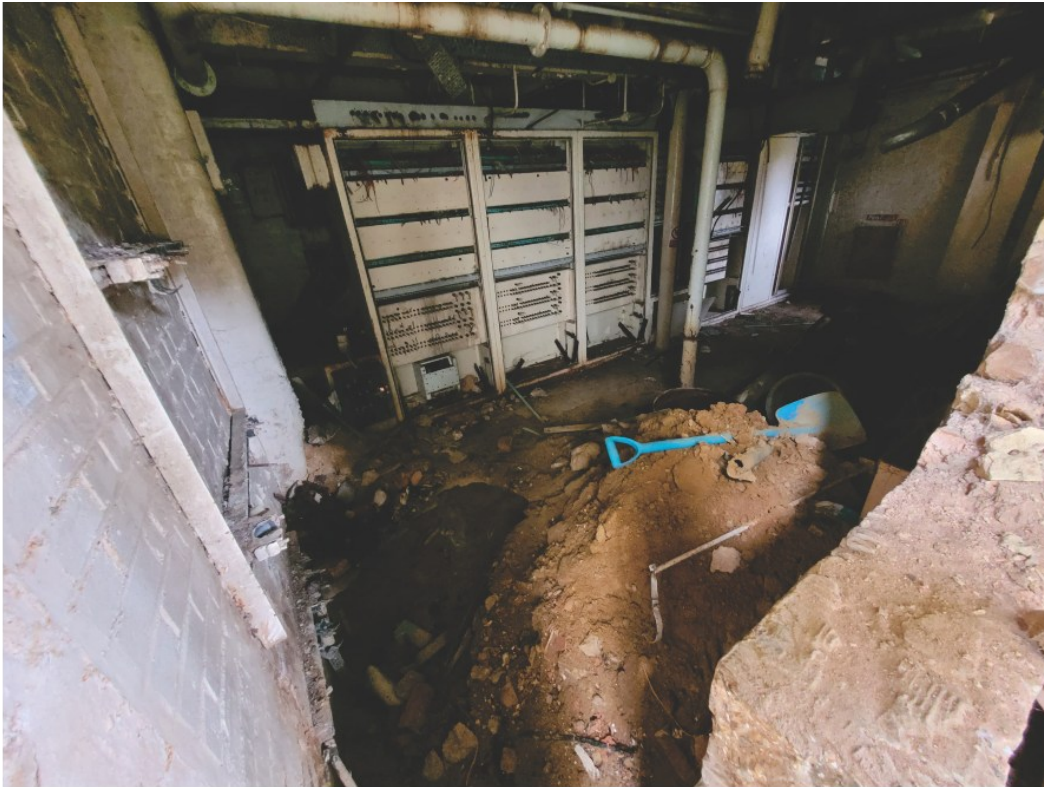
Pl. 25 Interior of the roller mill showing recent excavation to inspect foundations
