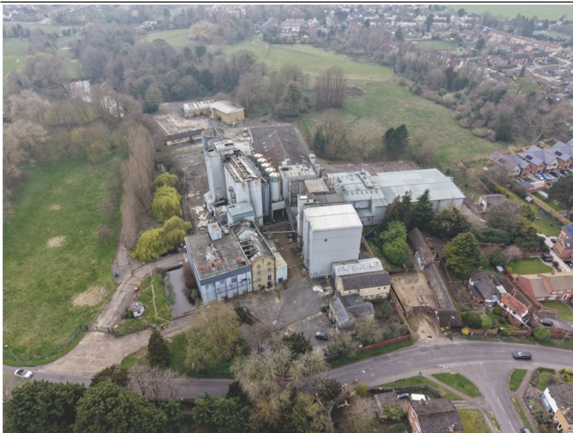
Pl. 1 Bowman's Mill, aerial view looking west (Reclaim Heritage)
