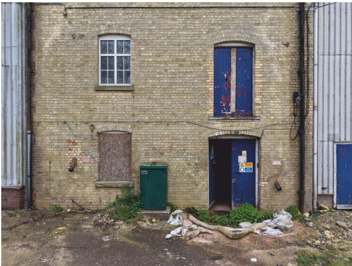
Pl. 20 East gable taking in door and entrance.
