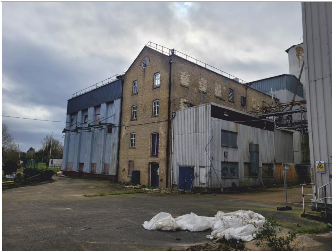
Pl. 15 General view looking south-west showing north elevation of the roller mill above the blower house
