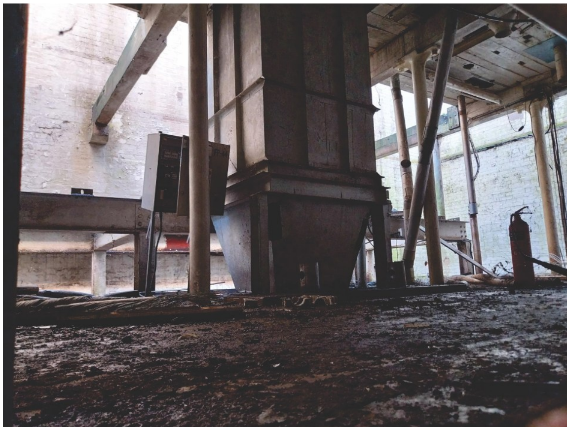
Pl. 42 Second floor looking south-west 2026 (Peter Bull)
