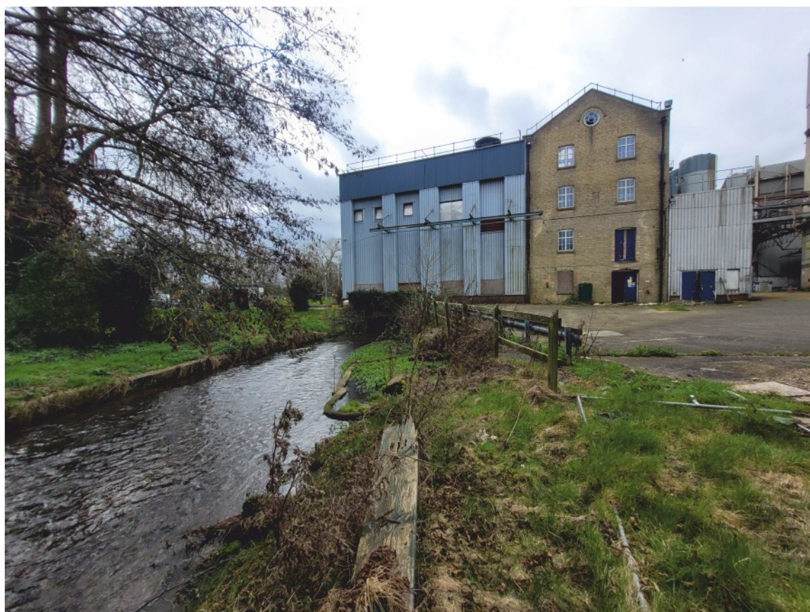
Pl. 6 B Mill (left), roller mill centre and blower room right, looking west
