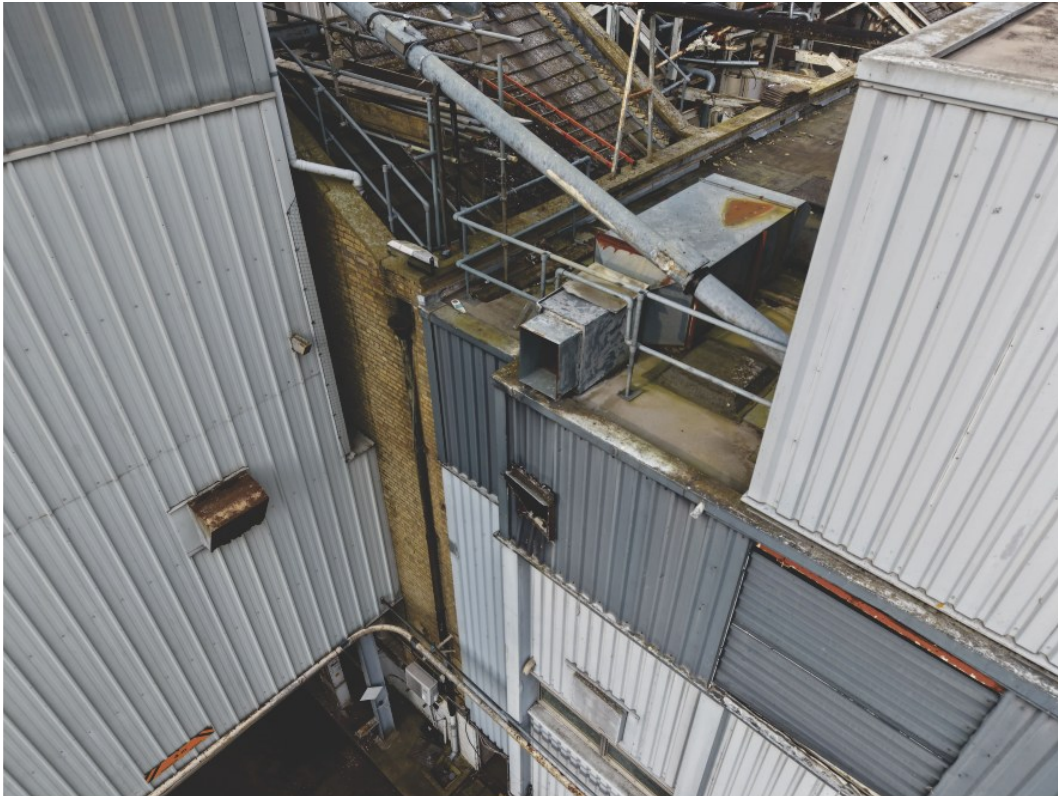
Pl. 27 The south-west corner of the building at roof height showing the low parapet capped with flat concrete slabs (Reclaim Heritage)
