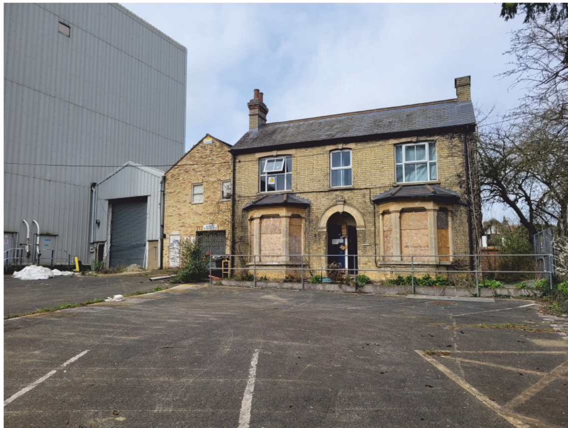
Pl. 8 Mill House, former manager's house, later used as offices, with two workshops to the left
