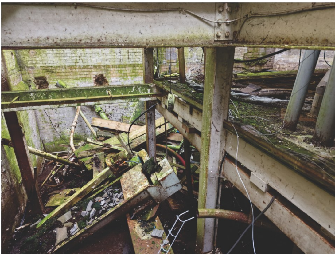
Pl. 34 Roller mill ground floor interior south side 2026 looking west (Reclaim Heritage drone image)
