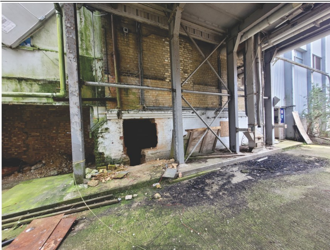
Pl. 23 West gable looking south-east
