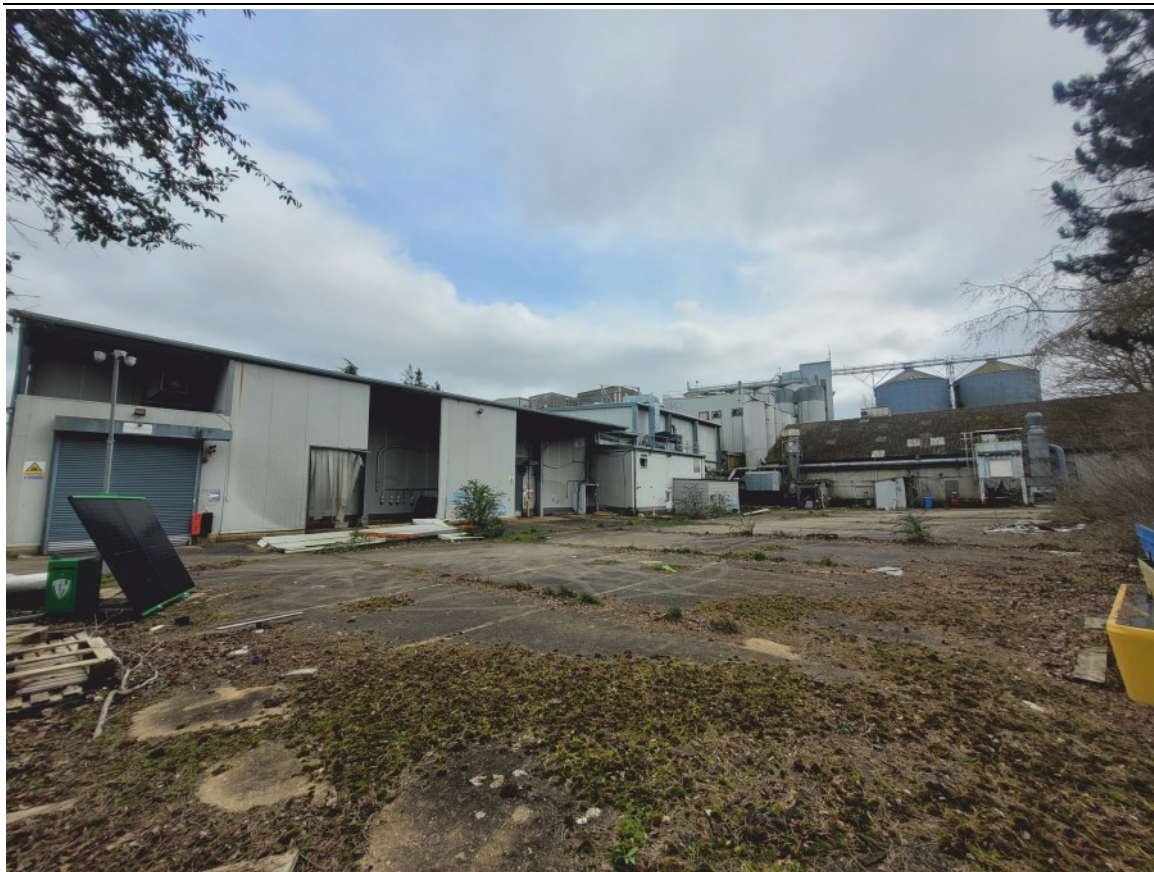
Pl. 5 BI warehouse (left) looking south towards the warehouse with silos to the rear.
