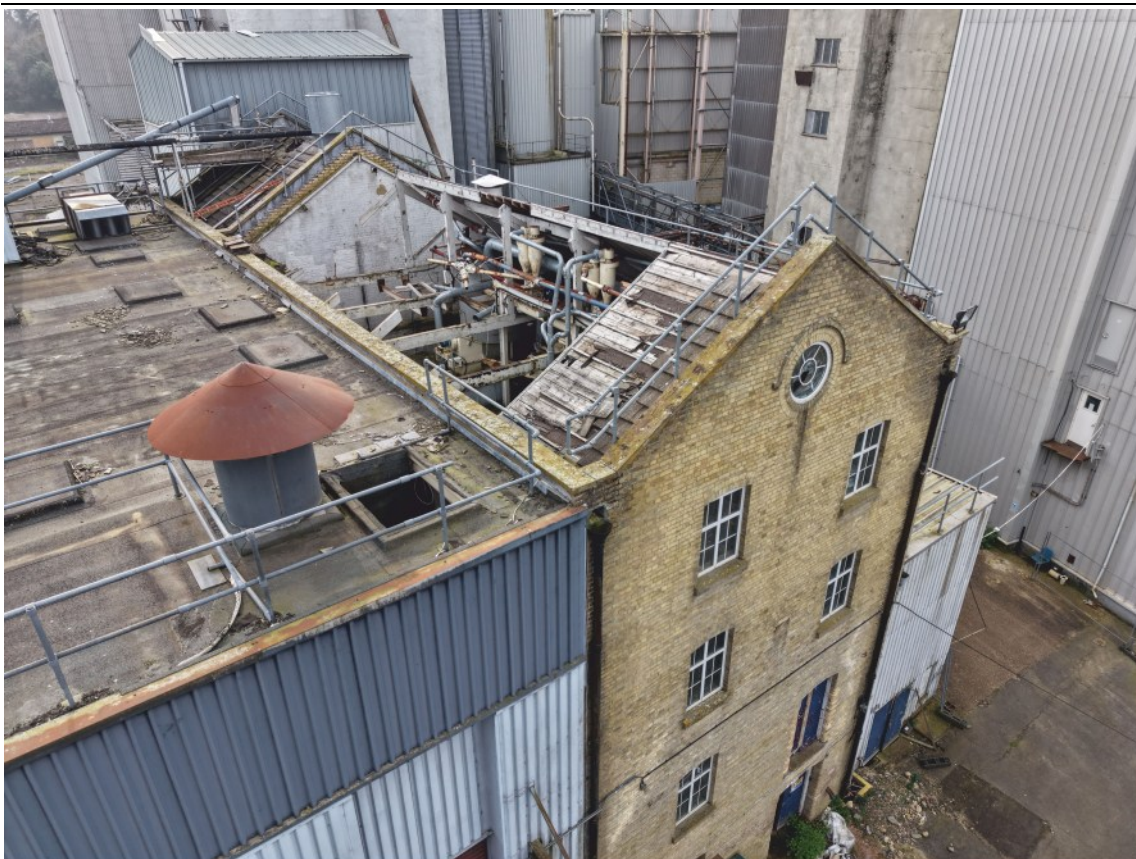
Pl. 17 View across the roof looking north-west
