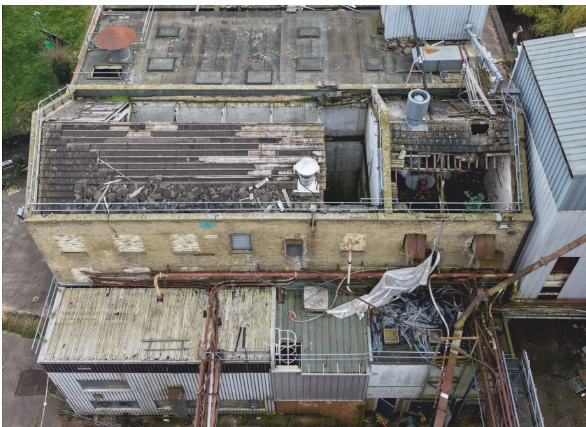
Pl. 18 The roof looking south
