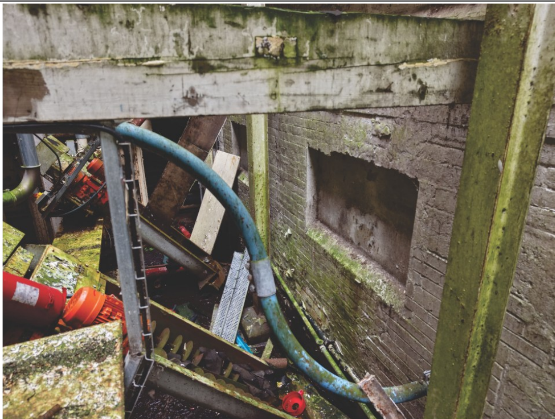
Pl. 33 Roller mill ground floor external south elevation 2026 looking west (Reclaim Heritage drone image)
