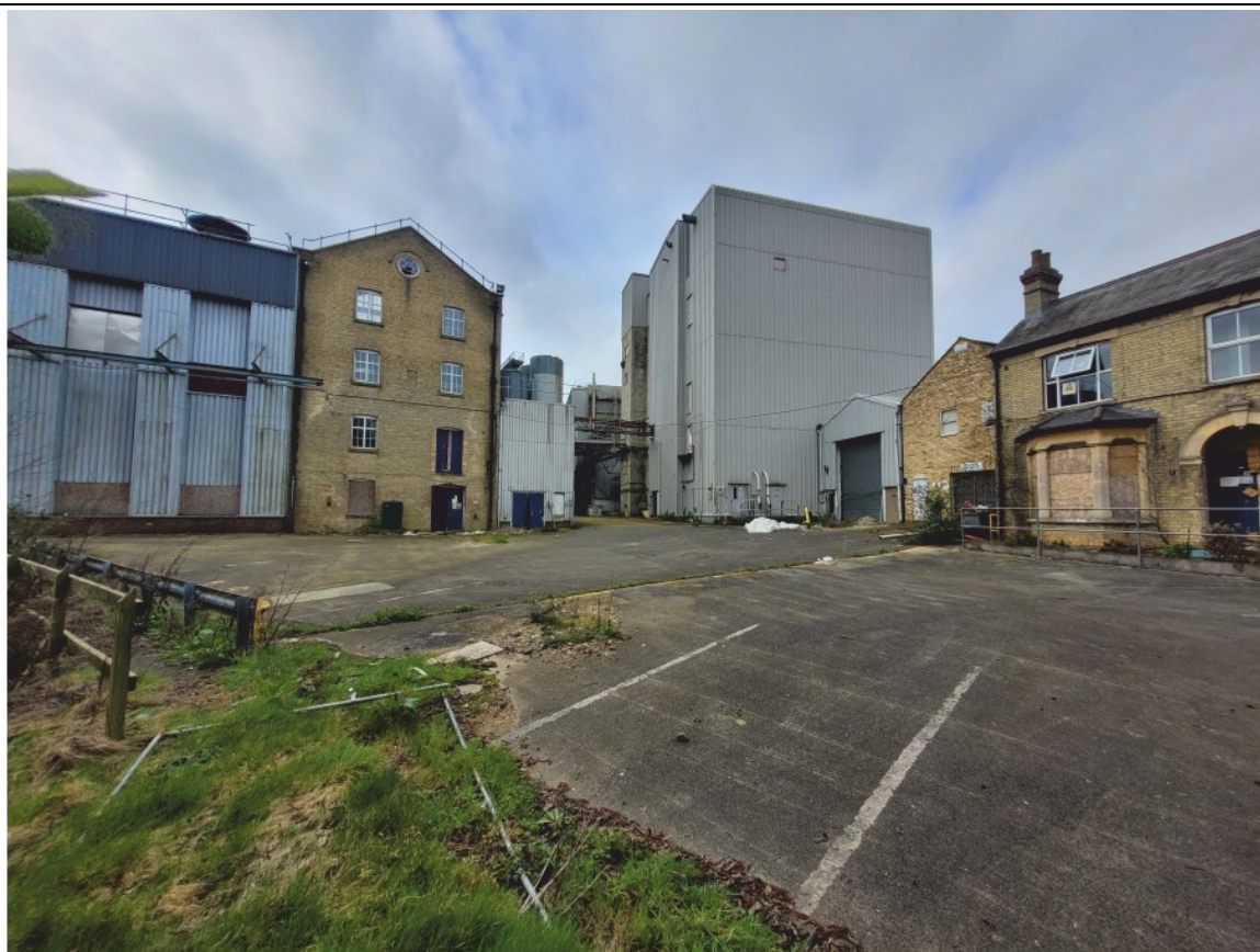
Pl. 7 General view across yard towards the warehouse
