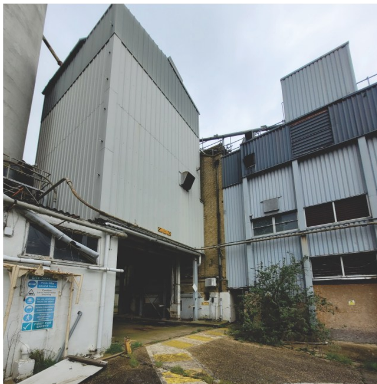
Pl. 26 South west corner of the roller mill masked by adjacent conditioning bins (left) and C Mill (right)
