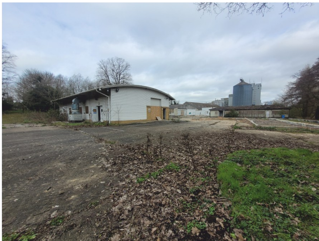
Pl. 4 Bowmans Mill looking east, with modern BI Pilot plant centre in foreground with warehouse centre rear and silos to right behind lab and office buildings
