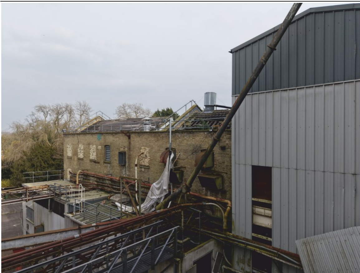
Pl. 21 North elevation showing blocked windows and vents looking south-east
