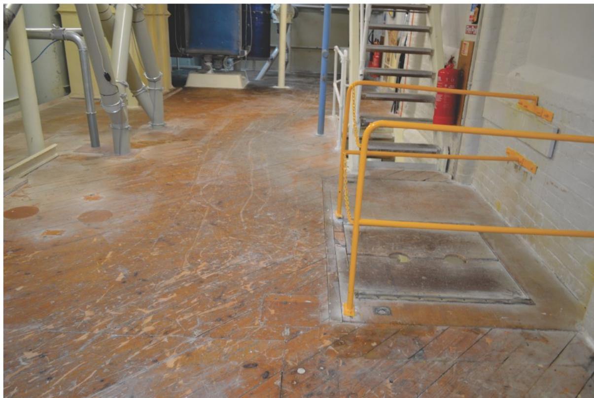
Pl. 38 Second floor trapdoor with stair to third floor behind, looking west 2017 (N. Field)
