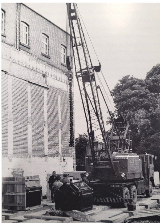
Pl. 12 Construction of the new mill 1969-70 showing the south elevation of the roller mill, looking north-east (Bowman 1997).
