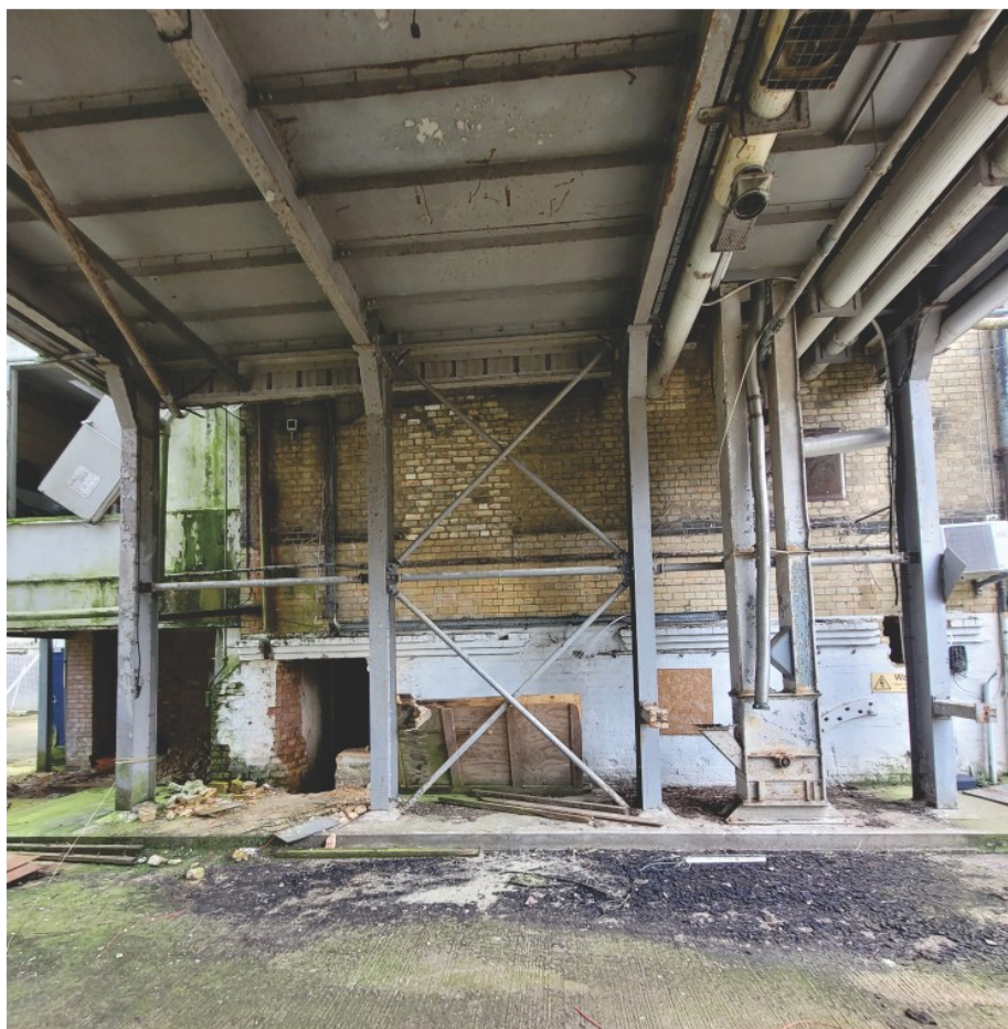
Pl. 24 West gable looking east
