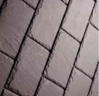
NEW ROOFS: NATURAL SLATE
