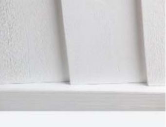
PAINTED TIMBER FEATHER EDGE TO MODERN RANGE AND UPPER GABLE OF HISTORIC RANGE.
