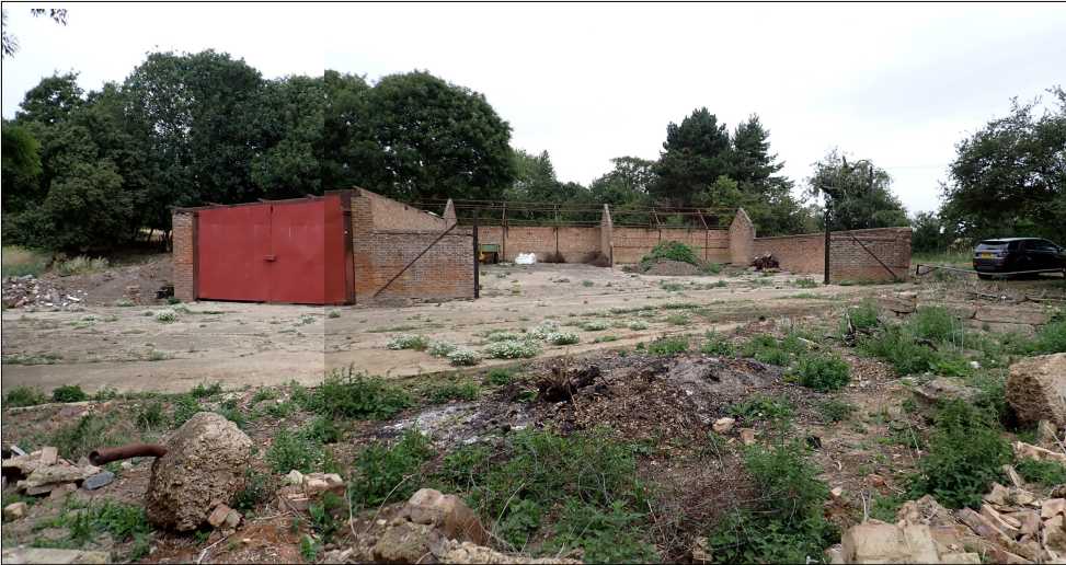
VIEW NORTH TOWARDS BUILDING – LEAN-TO (LEFT) & FORMER CATTLE SHED (RIGHT)
