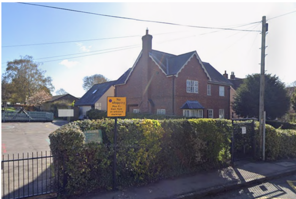
Figure 2. Google Streetview of site.
