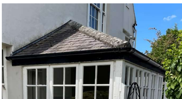
Concrete hip tiles to be removed
