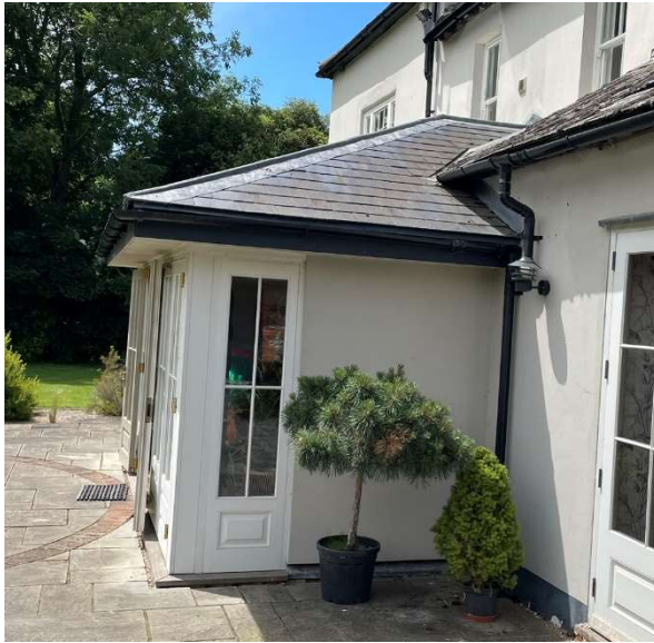
Lead roll hips on the 2013 rear extension
