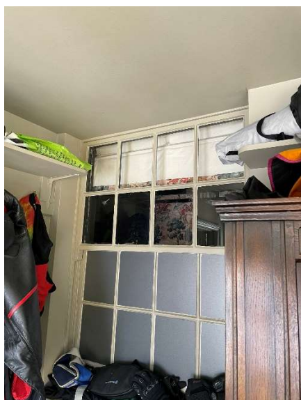
Internal window with adjoining plasterboard ceiling which is to be removed to create a tapered shallow shaft for the new rooflight
