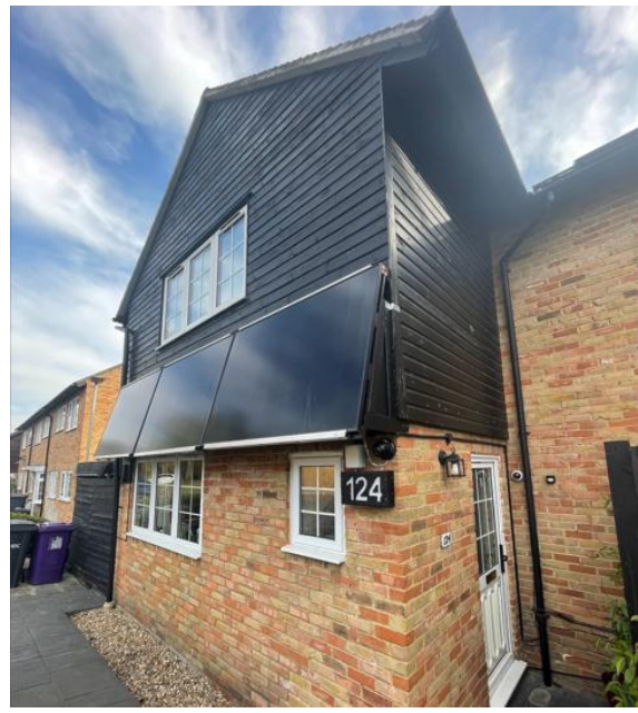
Solar panels in-situ on the front elevation of the property
