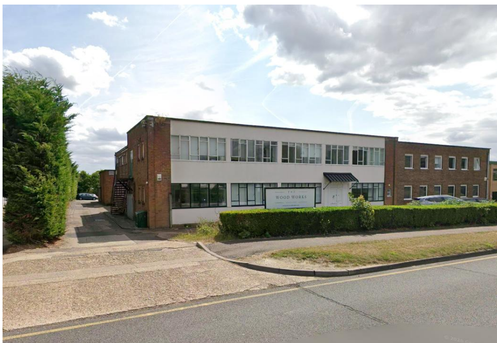
Figure 2: Principal Elevation of the site from Blackhorse Road, showing front office area and side access to service yard
