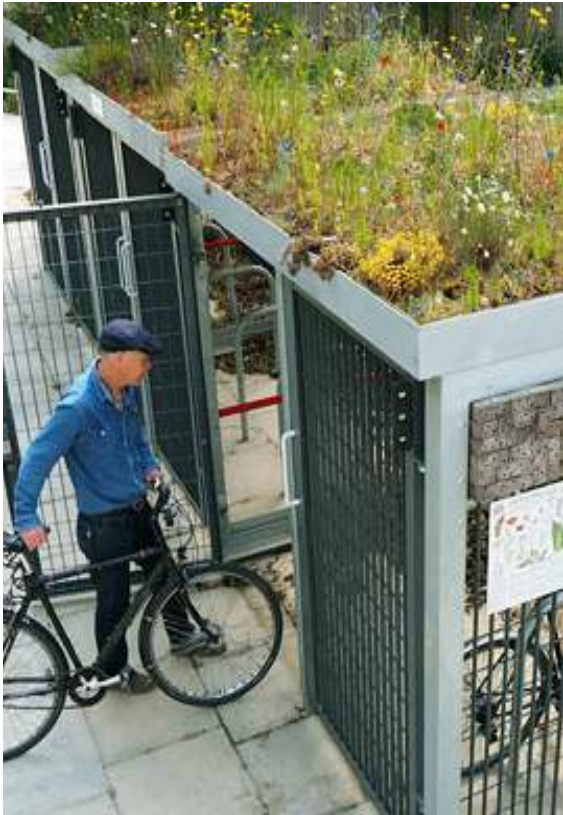
Green Roof to Cycle Shelters
