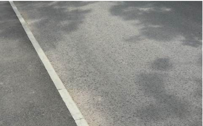
Tarmac access road and Maintenance footpath
