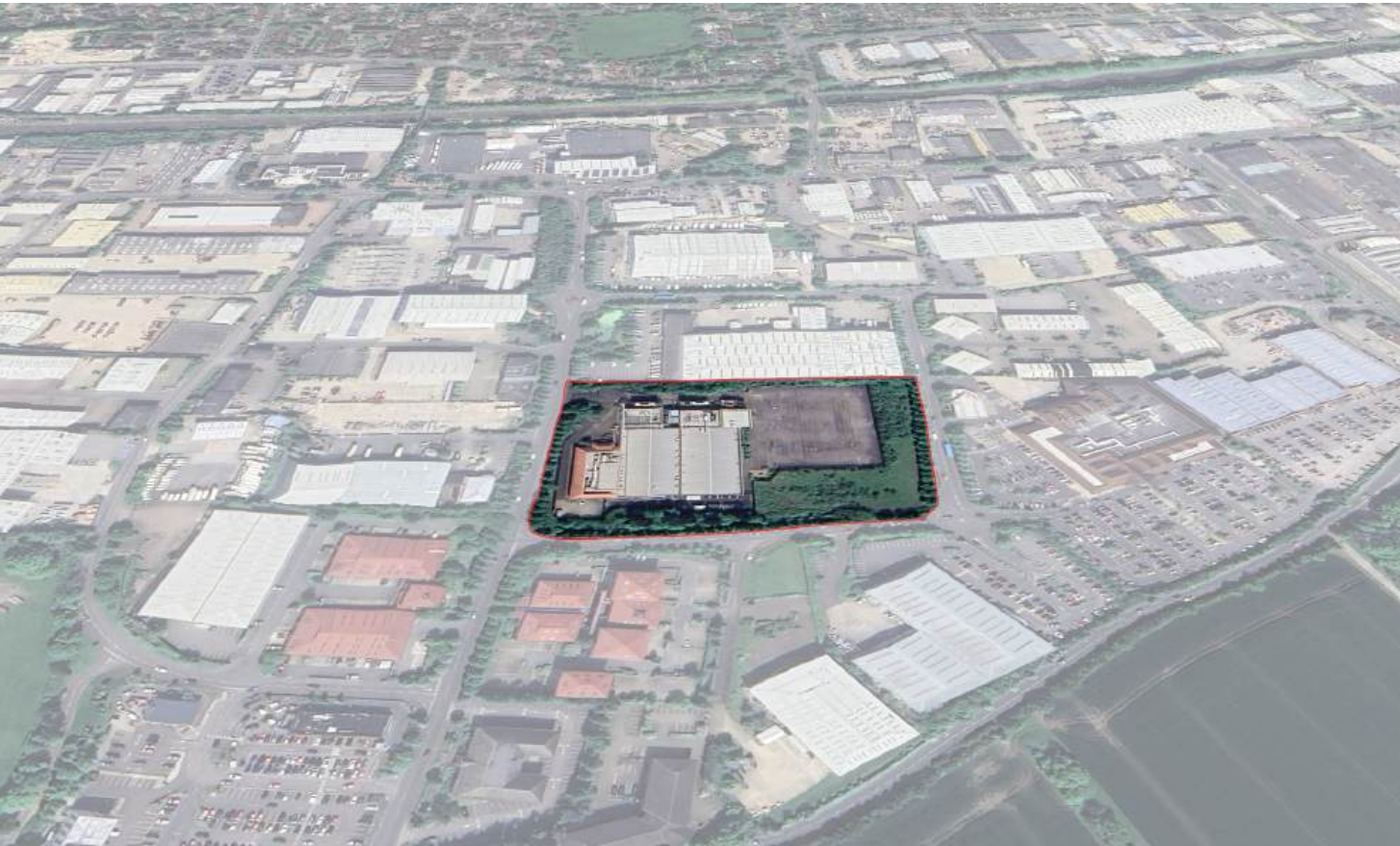
AERIAL LOOKING NORTH
