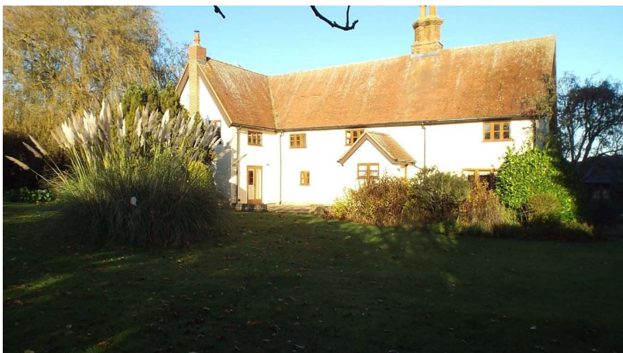
Mill End Farmhouse rear elevation with large willow tree to the left, Propbar
