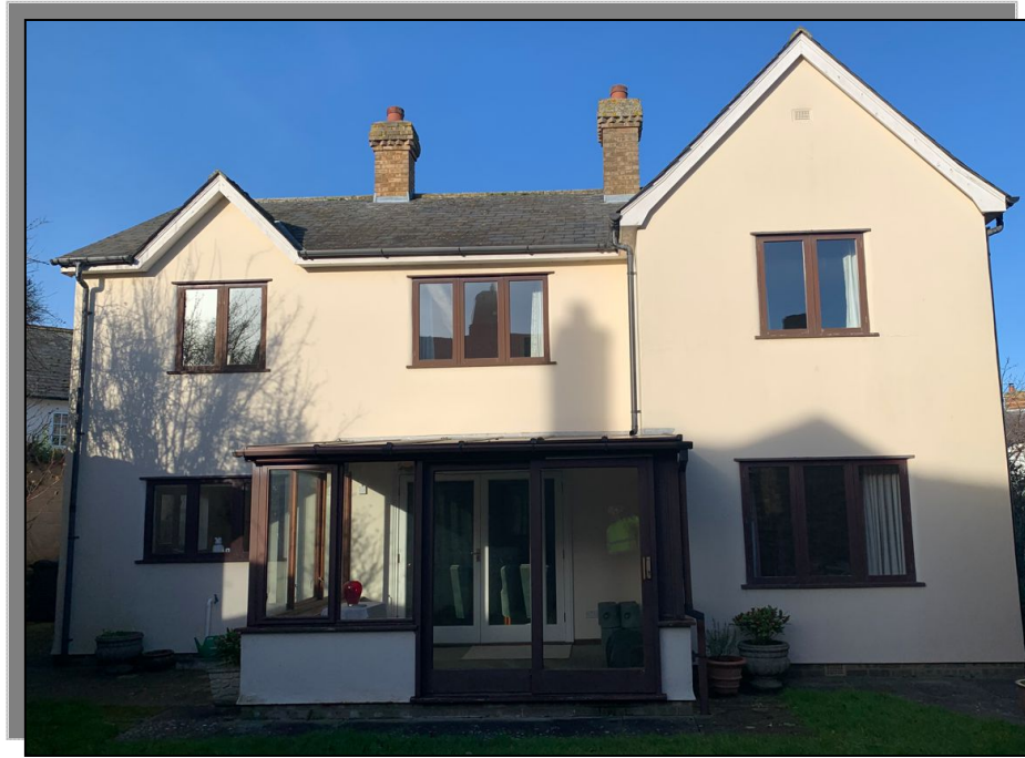
Photograph indicating the south-east elevation of the property overlooking the rear garden.
