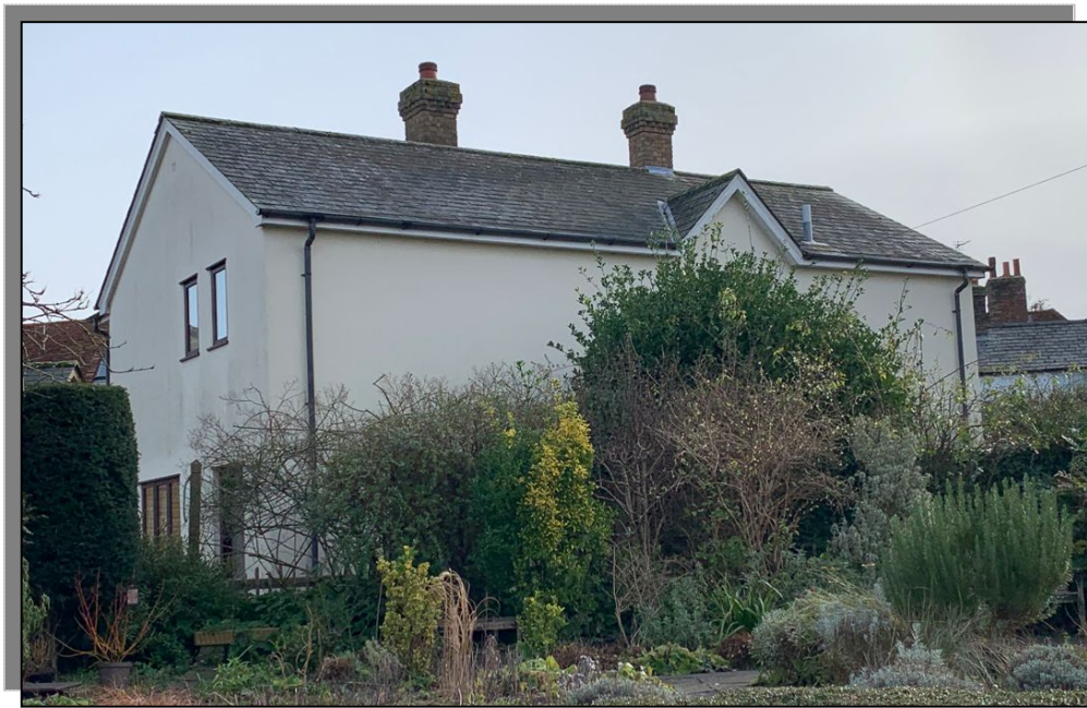
Photograph indicating the north-west elevation of the property.
