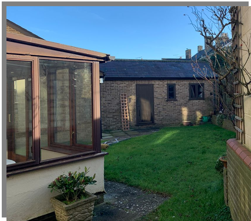
Photograph indicating the side elevation of the existing store facing the rear lawn and to the rear of the double garage to be converted into ancillary residential accommodation (guest bedroom/study).
