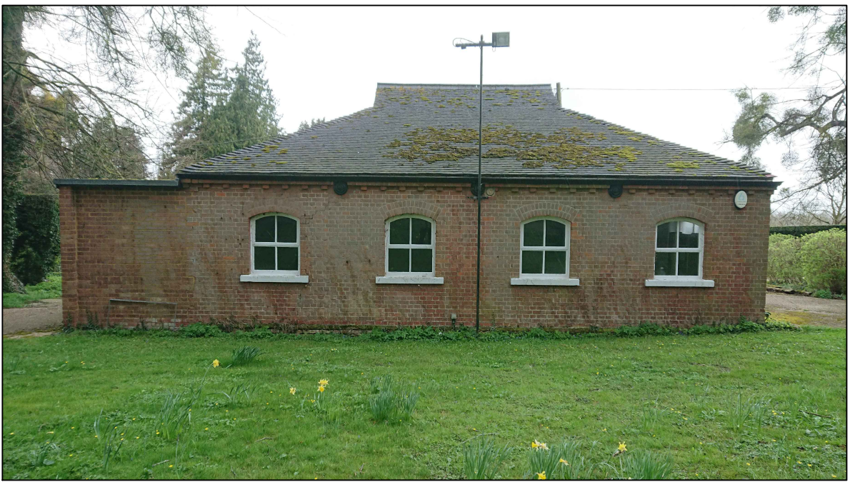
Existing Bothy Image (South)
