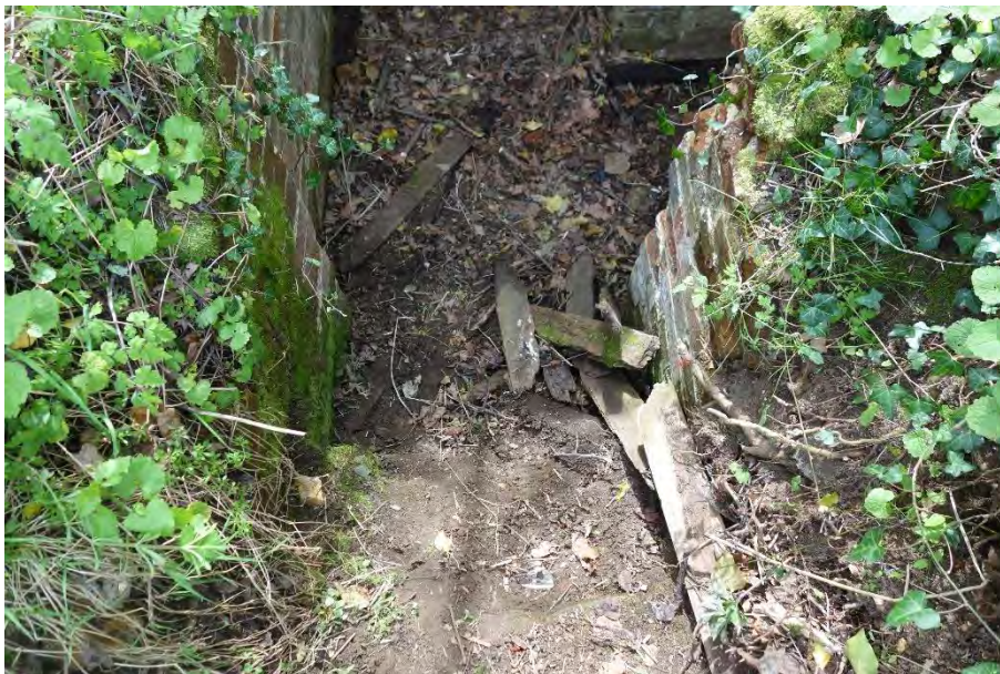
Photograph 2: Remains of step access down into the passageway
