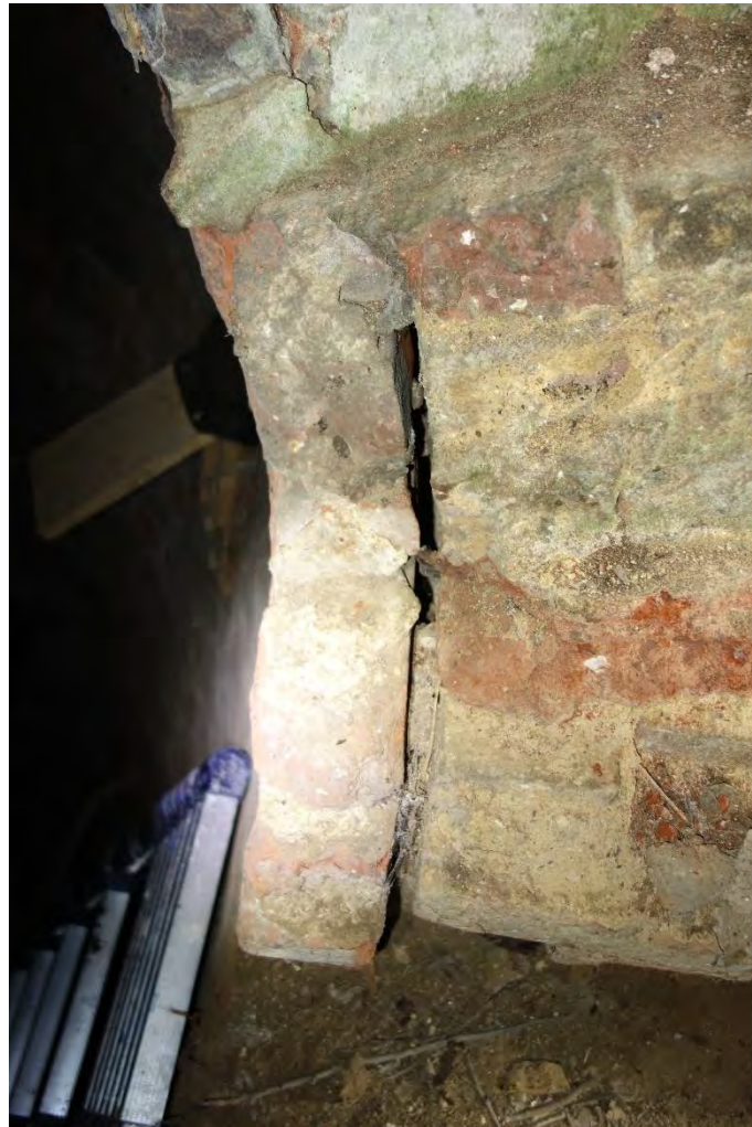
Photograph 9: Partial section view through the dome brickwork showing separate inner leaf
