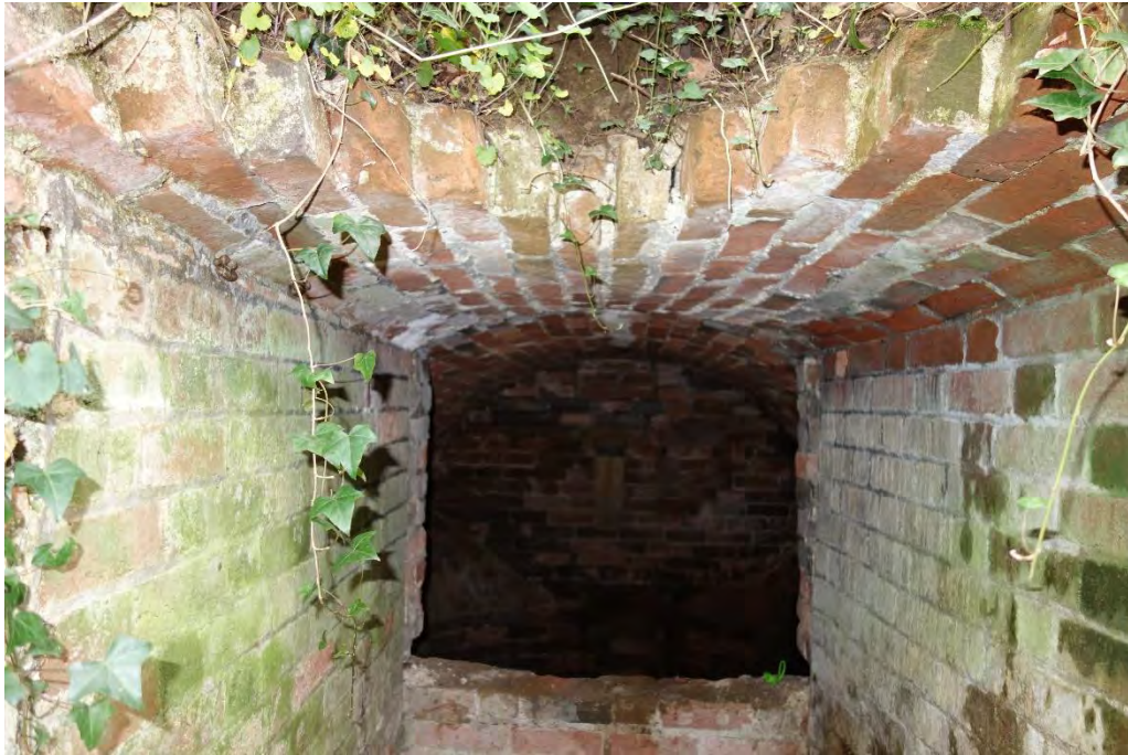
Photograph 6: Flattened arch at the entrance passage to No.2
