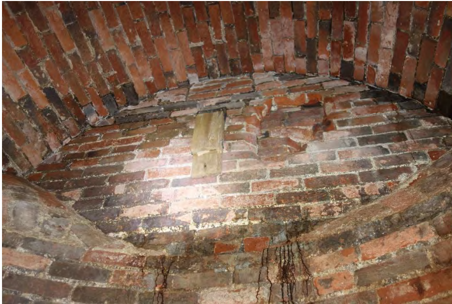
Photograph 11: Chamber interior showing part of the barrel vault roof, infill wall and corners.
