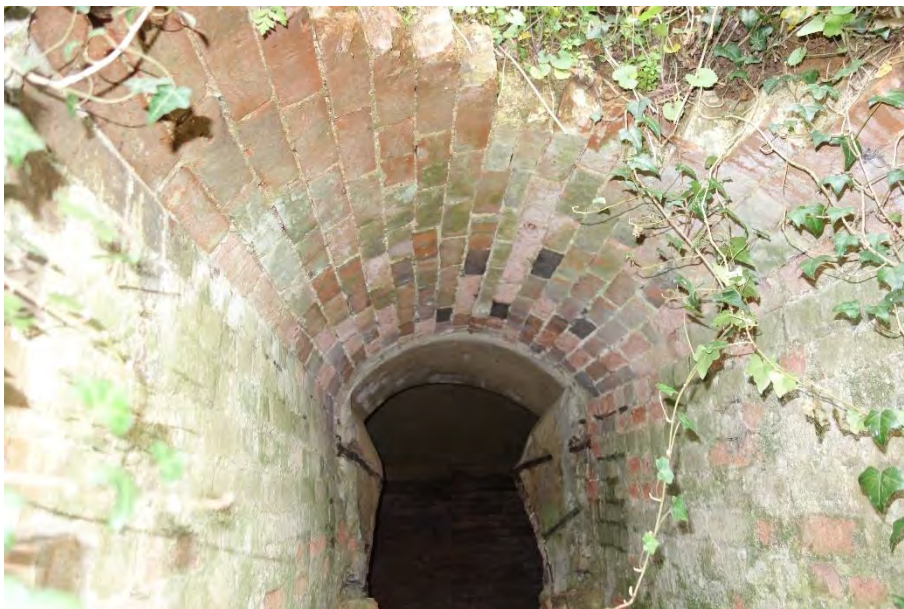
Photograph 4: Access passage to No. 1
