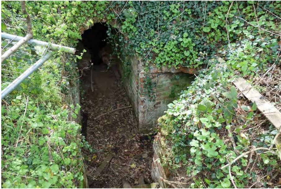
Photograph 3: General view of the access passageways
