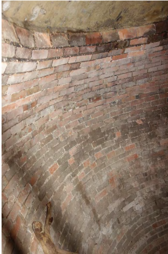
Photograph 7: General view of the chamber showing inward taper at lower level with the dome brickwork returning inwards.
