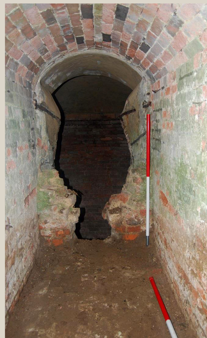
Looking into Ice House 1 through the brick-vaulted entrance passage. The domed chamber can be seen beyond (2m scale)
