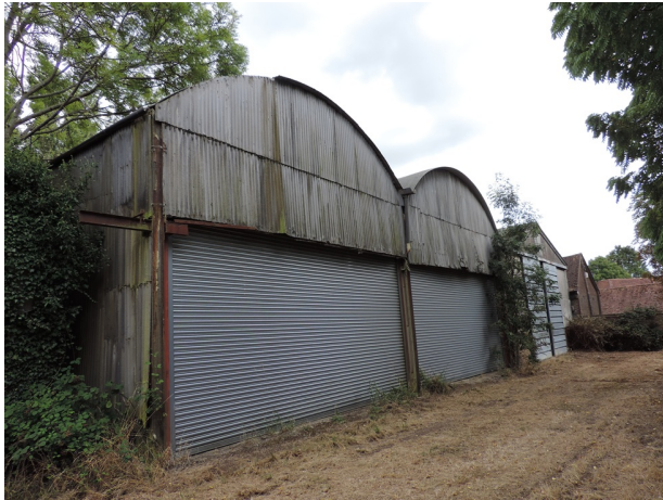
Photo 4. West end (front) of northern barn.
