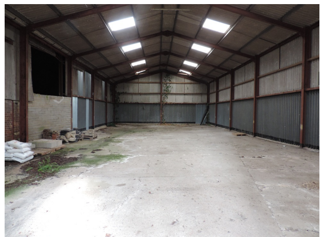
Photo 7. Interior of southern barn looking east.
