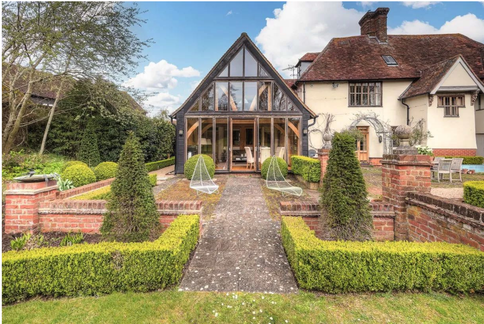
SOUTH ELEVATION OF 'GARDEN ROOM'
