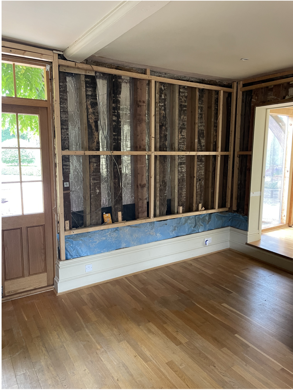
INTERIOR OF CURRENT GROUND FLOOR SITING ROOM
