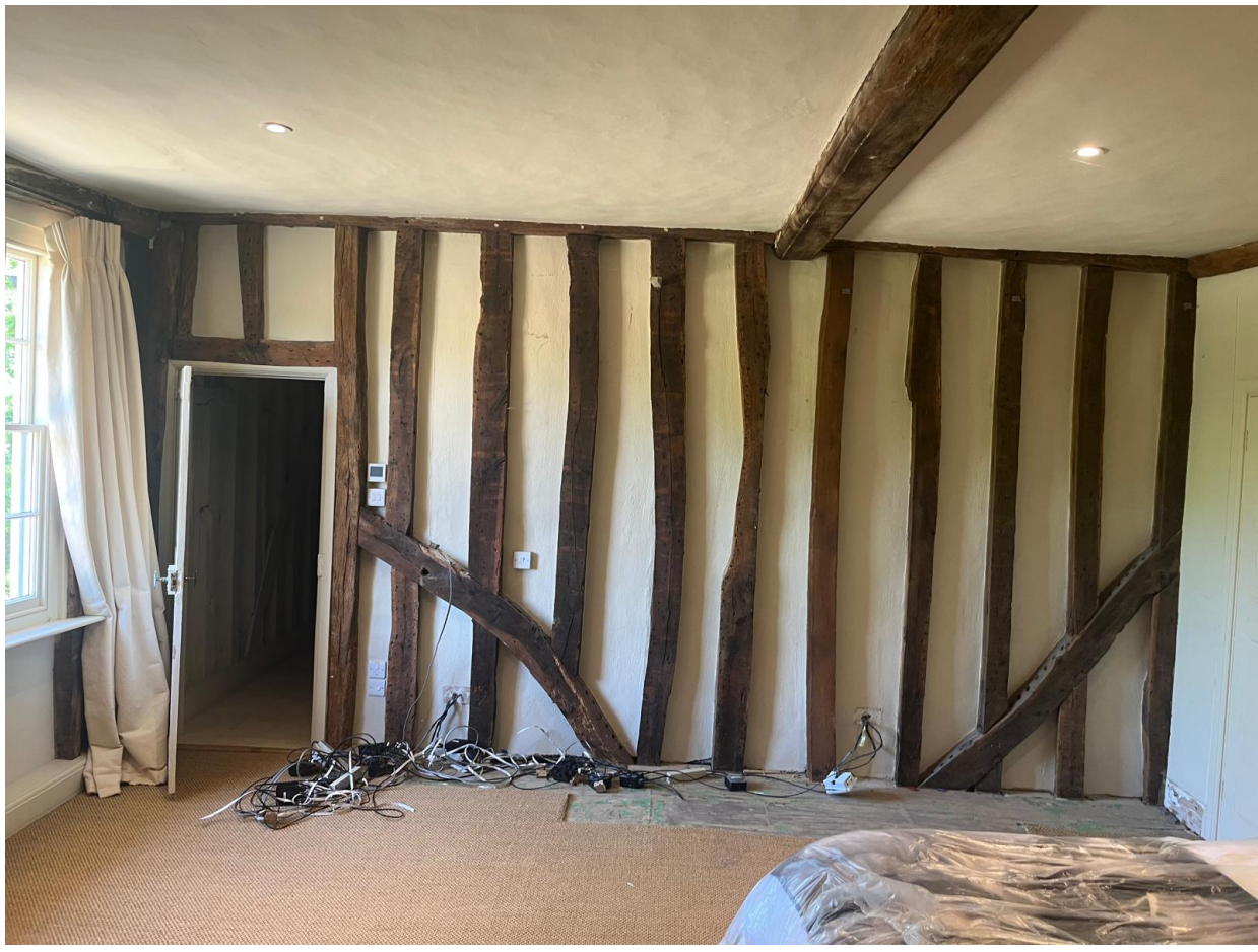
EAST INTERIOR WALL OF FIRST FLOOR BEDROOM 2
