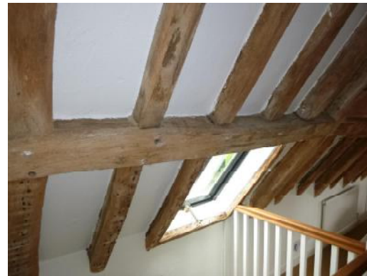
Window set above stairwell
