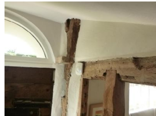
Timber header cut out at door head
