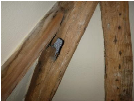
Empty mortise in hip beam, packed with wire mesh (17)
