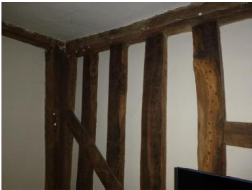
Heavy timber framing in bedroom 2
