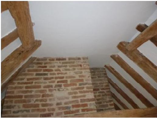
Ceiling, looking towards chimney
