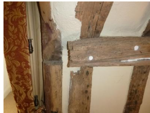
Detail of eaves rail - no intervention required (5)
