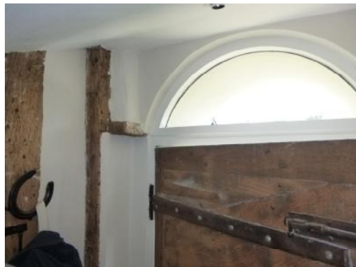
Arched fanlight above front door, with timber header cut out to make way
