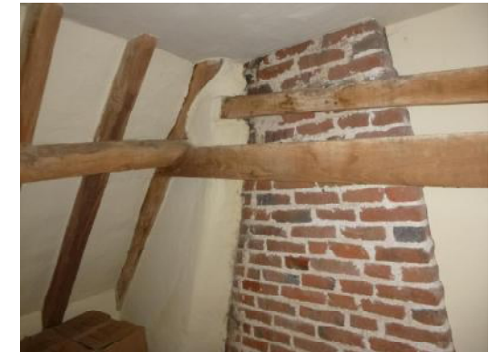
SE corner of bedroom, with collars in front of chimney breast
