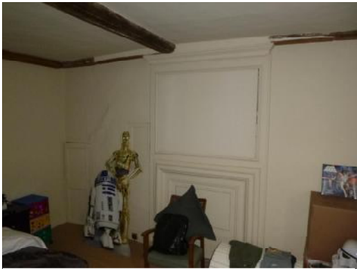
Panelled-over fireplace in first floor bedroom
