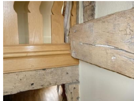
Side rail of stairwell tower
