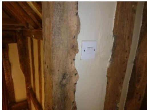
End of eaves rail visible in plastered face
