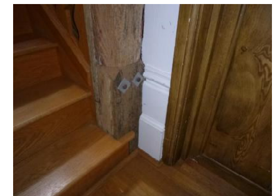
Repaired rot damage to principal post (7)
