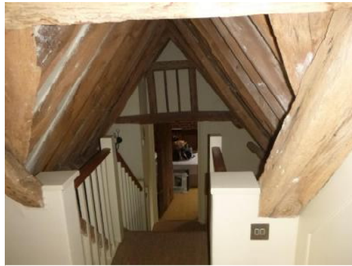
View from main attic into link, SE wing beyond down stairs
