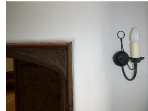
Gothic head of internal doorway, possibly relocated
