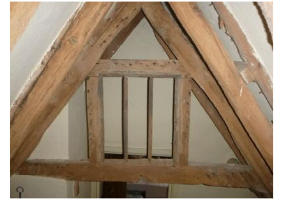
Historic gable framing and window of SE wing left in place above stairwell (20)
