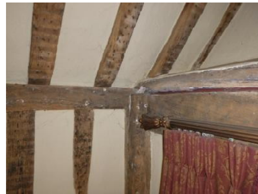
Tie beam at gable of stairwell dormer
