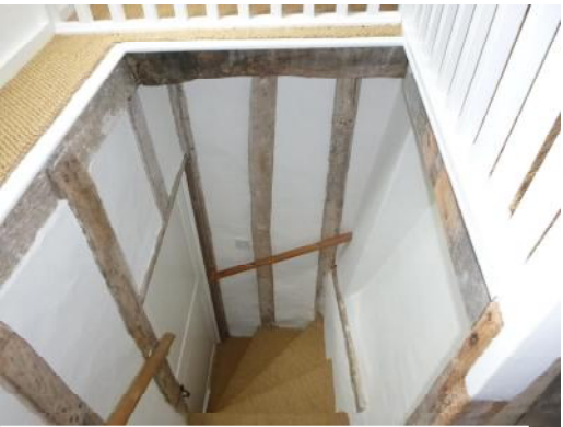
View down stairwell from bedroom
