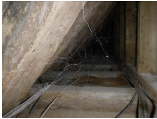
Front eaves, showing eaves wall (non-structural) supported on attic floor joists
