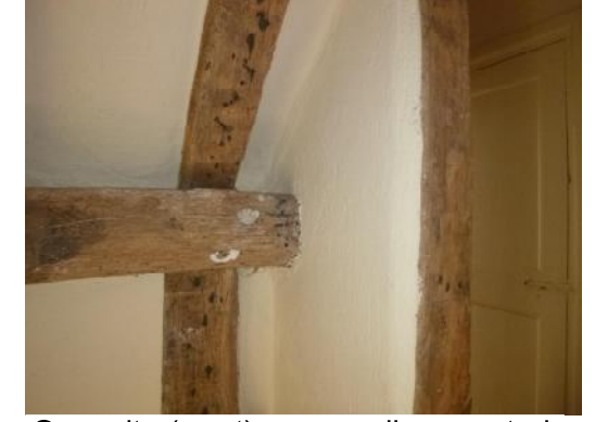
Opposite (west) eaves rail supported at stud in landing wall
