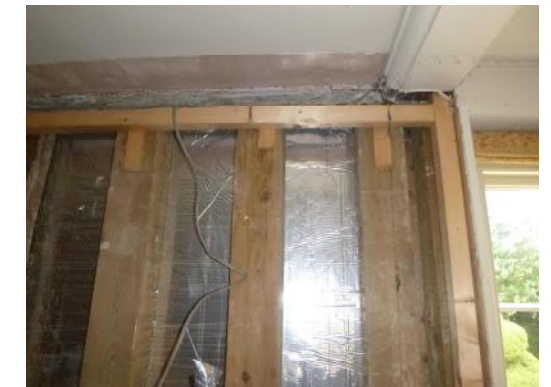
Replacement studs with foil-faced insulation and lined with softwood battens (2)
