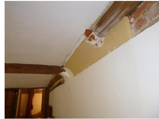
Repair at chimney end - possible related to removal of hearth at first floor level
