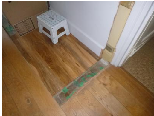
Repaired floor in first-floor bedroom
