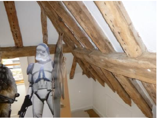
Purlins meeting at hipped corner
