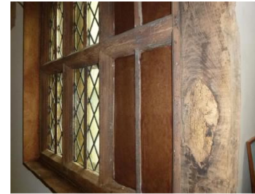
Window boarded up
