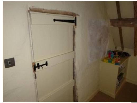
Doorway to stairwell adjacent to chimney
