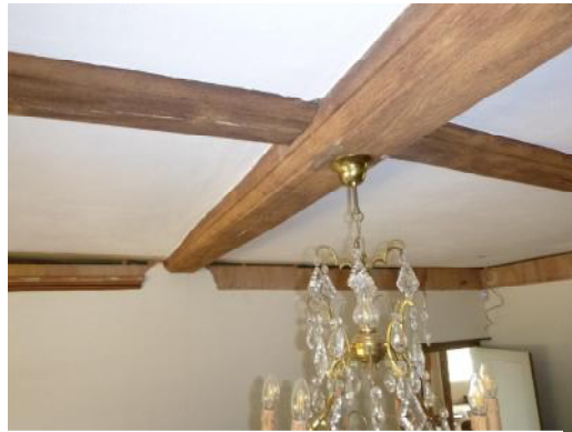
Beams at first floor level - no problems reported
