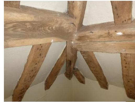
Empty mortise on hip beam (17)
