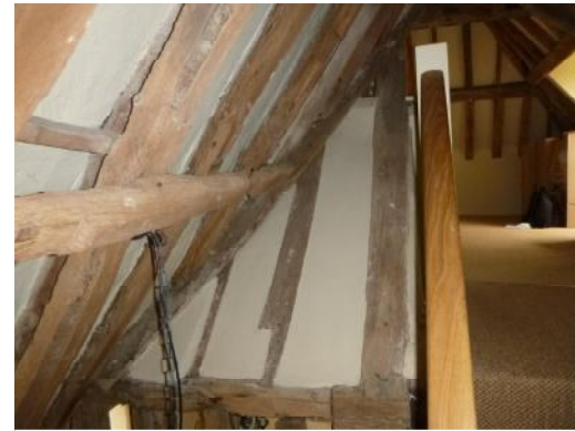
View towards main roof, showing rafters, eaves rail and handrail to stair
