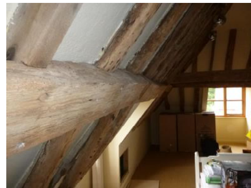
View along front (south) purlin (13)
