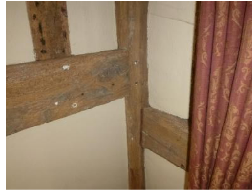
Framing of stairwell
