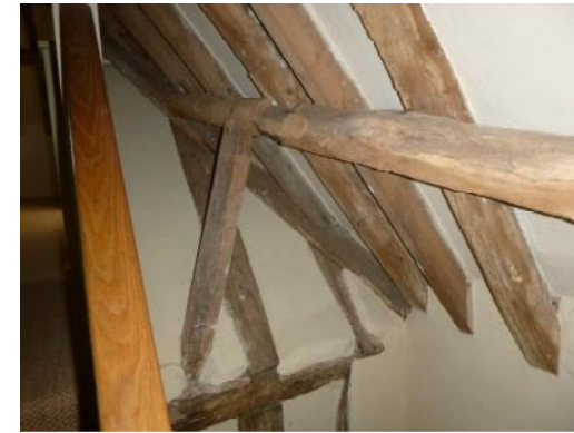
East purlin to link roof, propped from south wall of main house (19)
