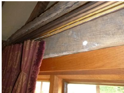
Head of replacement window to east of stairwell
