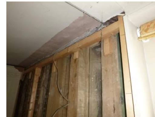
Replacement wall studs covered by modern softwood battens (2)
