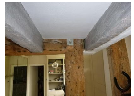
Stud-framed wall in east lobby near kitchen (9)
