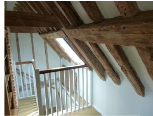
View towards stairwell, with collar above (4)
