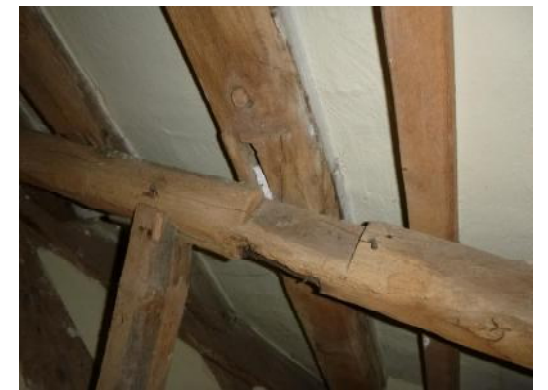
Detail of strut to purlin and empty mortise from removed collar (19)
