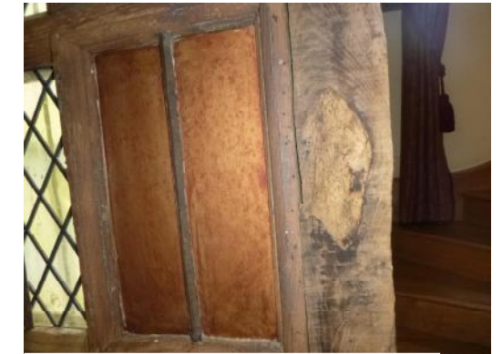
Rear window boarded up
