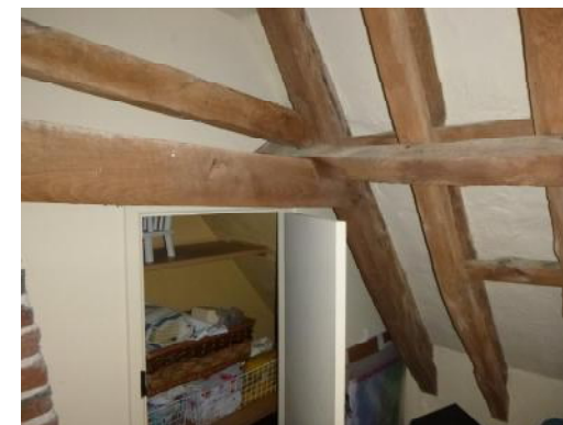
Cupboard between chimney breast and gable wall, above kitchen
