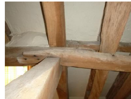
Collar in bedroom, with scarf joint in supported purlin
