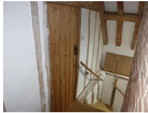
Stairs down to first floor, with limed timbers
