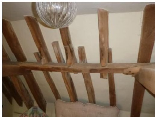
Purlin with rafters jointed over, suggesting position of former dormer
