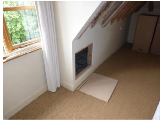
Hatch to front eaves
