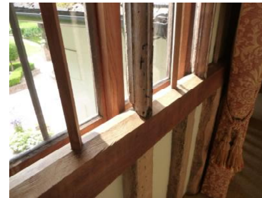
Repaired sill of older window to west of stairwell
