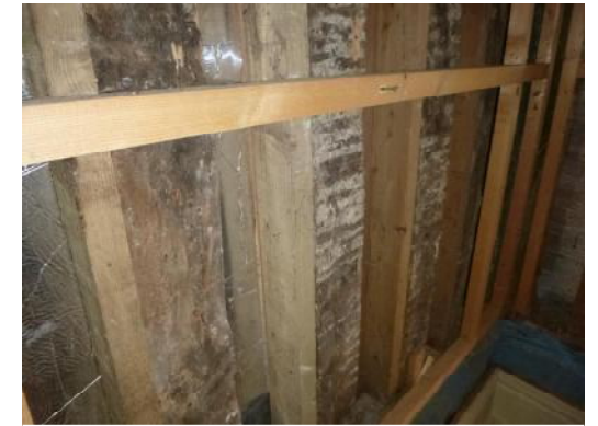
Replacement Oak studs lined with softwood battens (2)
