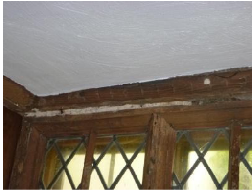
Mortar filler to gap above window head
