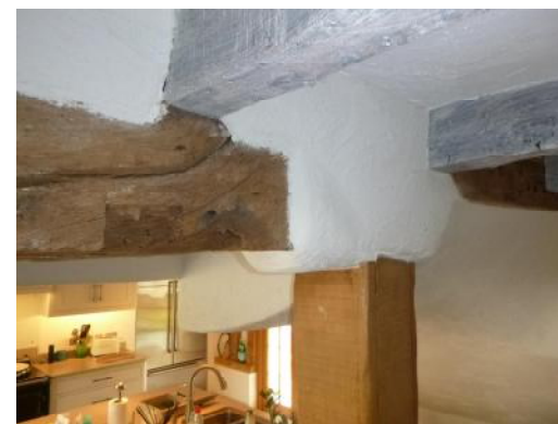
Support post and beam in kitchen (9)
