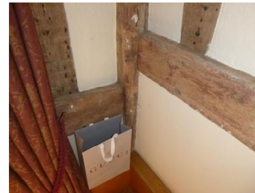
Framing of stairwell
