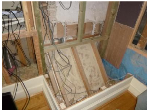
Framing of stairwell down to cellar. (The cellar was not inspected.)
