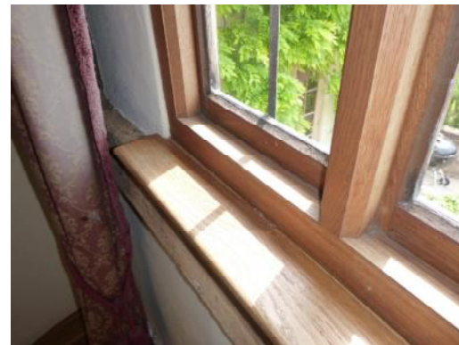
Replacement window to east of stairwell
