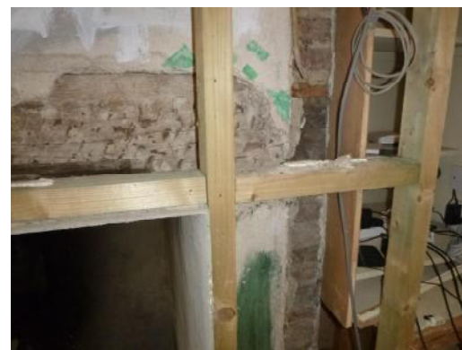
Softwood battens concealing adze-hewn bressumer
