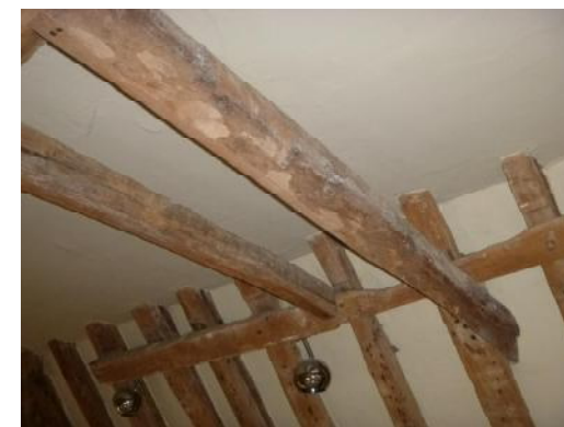
Collars repositioned at high level (11)
