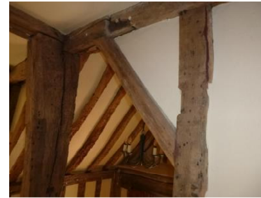
Framing to stairwell (4)
