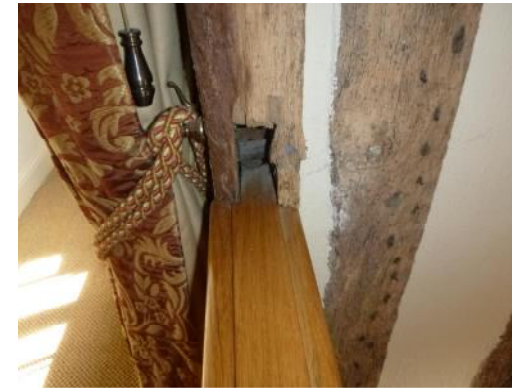
Handrail fitted into empty mortise
