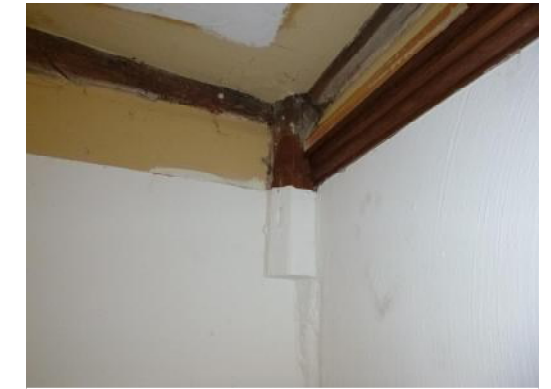
Pendant post at corner of ceiling
