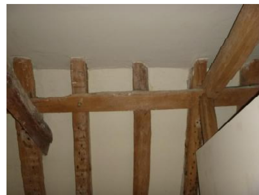
Collars repositioned at high level (11)
