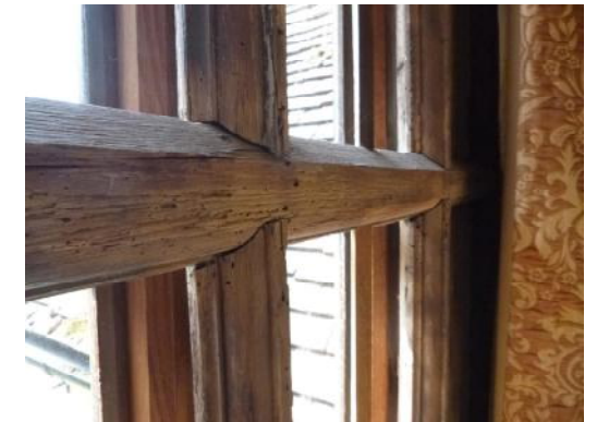
Transom of older window to west of stairwell
