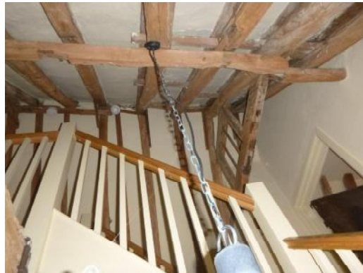
View up stairwell showing former gable with window, now enclosed
