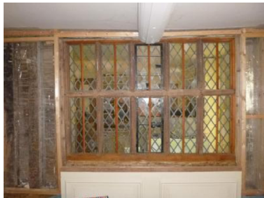
Window in west wall, with spine beam bearing on window head
