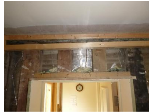
Modern framing to door head
