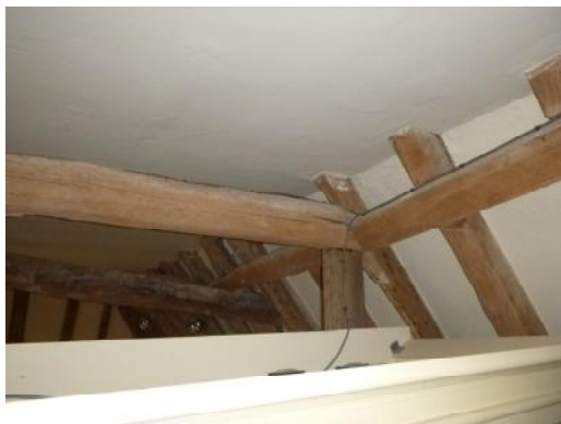
Framing above wardrobe/ partition (11)
