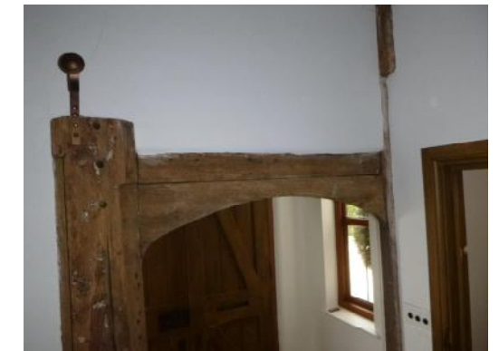
Truncated post used as jamb of internal doorway, possibly relocated
