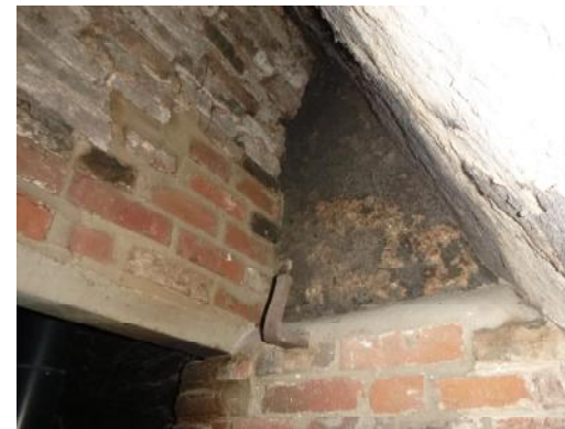
View from inside fireplace, showing concrete lintel supporting withy
