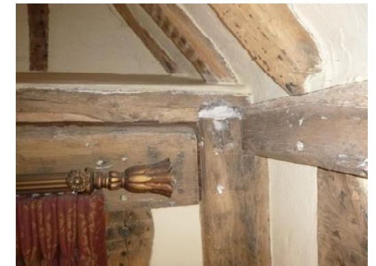
Detail at corner of stairwell
