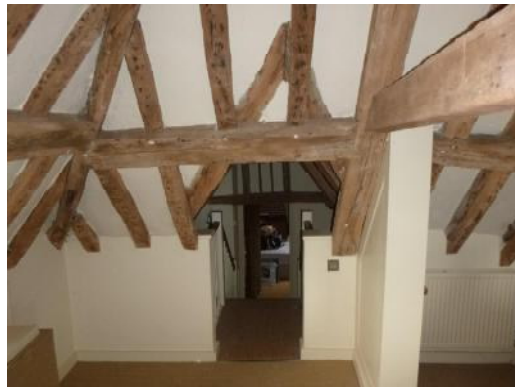
Looking into stairwell to SE wing (18)
