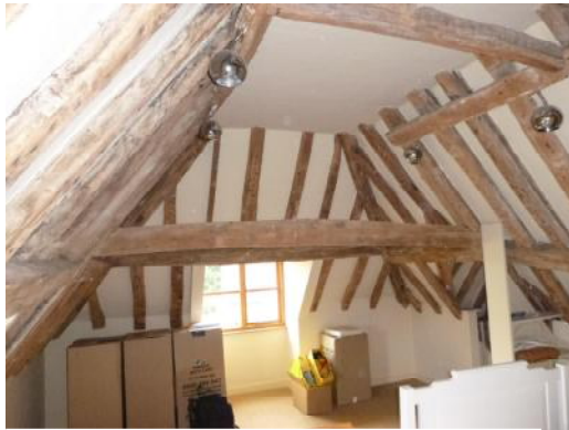
East attic bedroom, looking east
