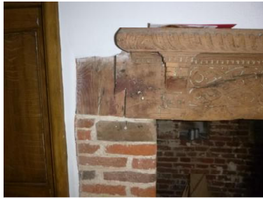
Left end of bressummer over dining room fireplace extended - possibly due to introduction into wider fireplace
