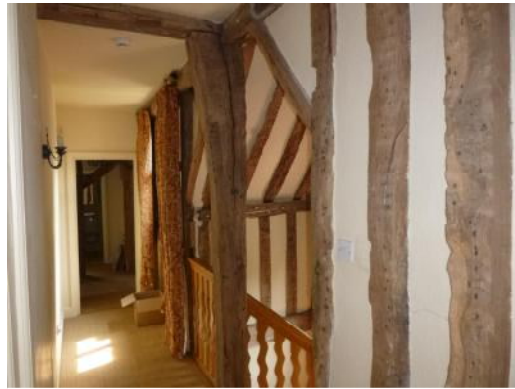
View along first-floor landing
