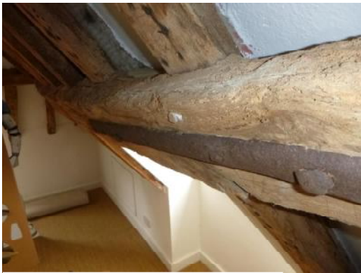
Wrought iron repair strap to front purlin (5)
