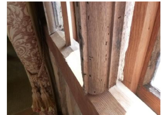
Repaired sill of older window to west of stairwell
