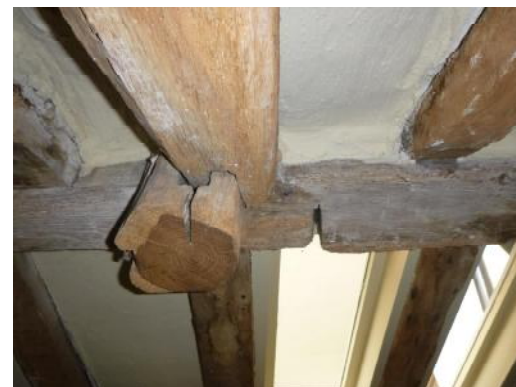
Stub of rail from former gable, severed when stairwell link was constructed
