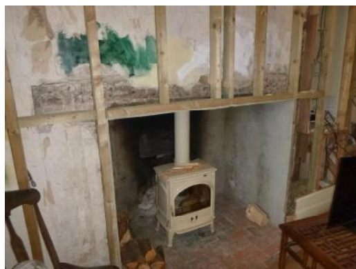
Chimney faced with softwood battens, with stove in fireplace
