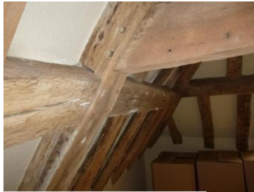
Principal rafter with tenoned purlins and collar (15)
