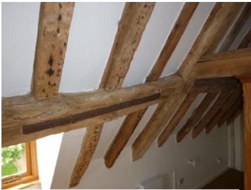
Front purlin with repair strap (5)
