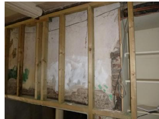
Modern softwood battens covering older fabric
