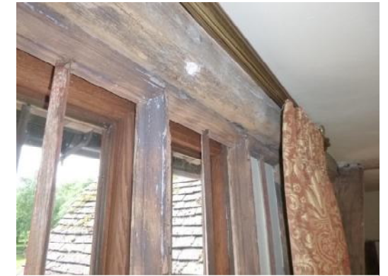
Head of older window to west of stairwell
