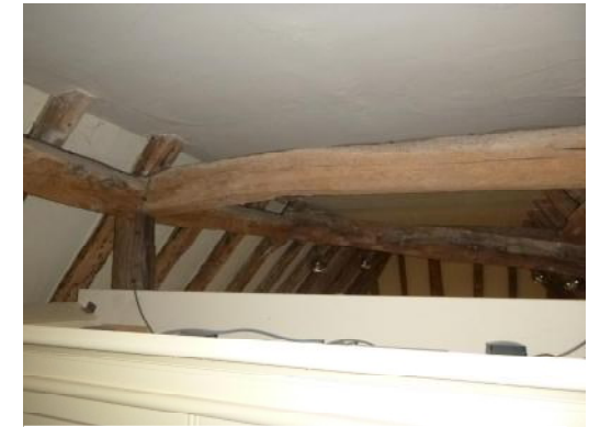
High-level collar above wardrobe, with posts introduced beneath (mainly to frame out wardrobe) (11)
