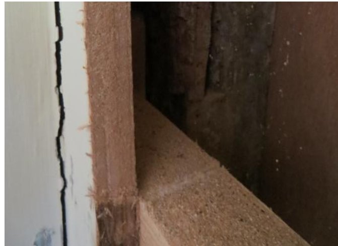
Figure 4.199: Showing the plywood and modern batten behind the historic corner cupboard.
