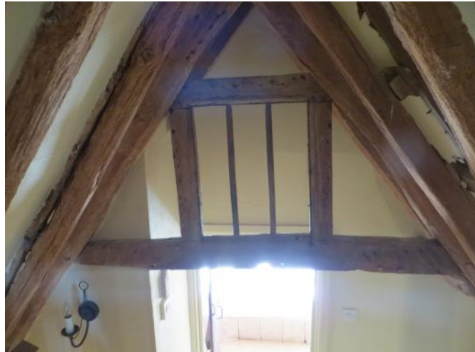
Figure 4.179: Showing the 16th century window on the northern wall of the south-eastern bedroom at loft level.
