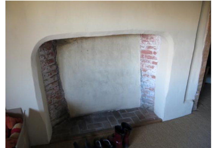
Figure 4.170: Showing the fireplace in the south-eastern bedroom.
