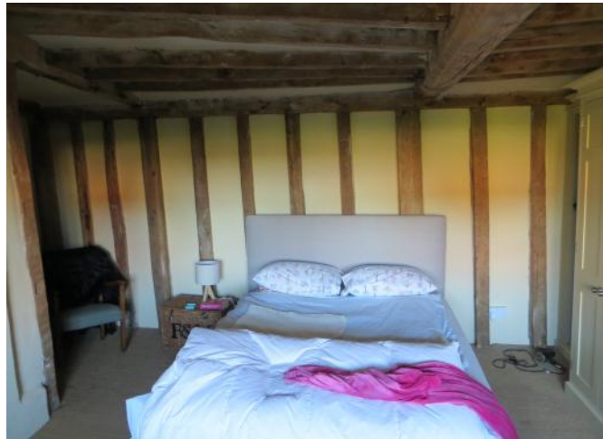
Figure 4.171: Showing the western wall of the south-eastern bedroom.
