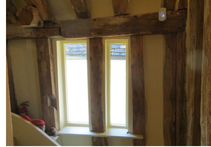
Figure 4.168: Showing the modern pair of single light windows inserted at first floor level adjoining the staircase.
