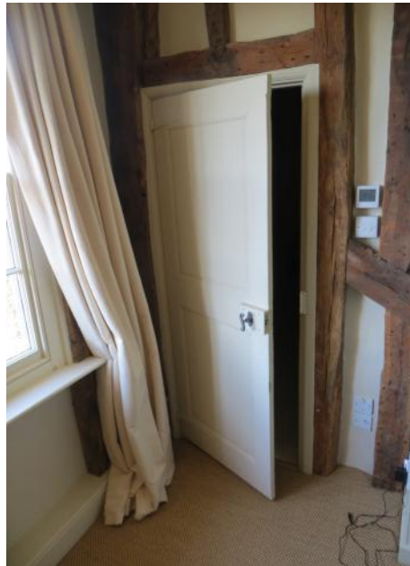
Figure 4.156: Showing the 2-panelled door into the shower room to the eastern side of the north-eastern bedroom.
