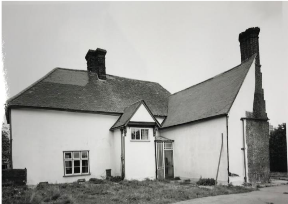
Figure 4.7: 1992-94 photograph showing the southern elevation of the main range and the kitchen cross wing (Source: Historic England Archives).
