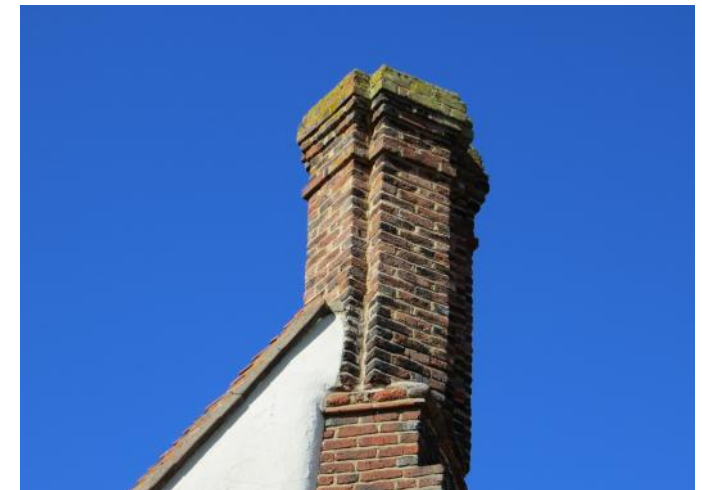
Figure 4.66: Showing the uppermost part of the stack at the southern end of the kitchen cross wing.
