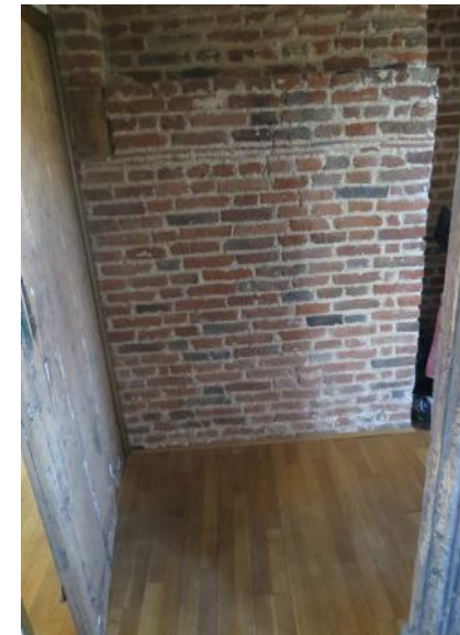
Figure 4.87: Showing the chimneybreast that lies opposite the main entrance.
