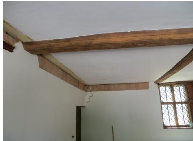
Figure 4.195: Showing the after modern cornices had been removed from the western side of the room.
