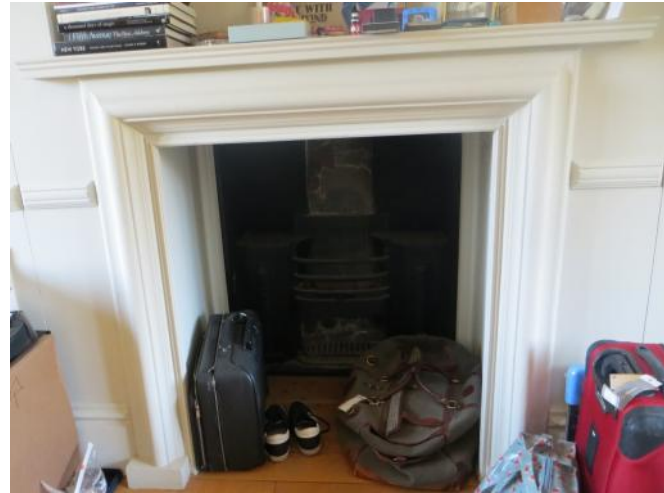
Figure 4.135: Showing the chimneypiece and hob grate.
