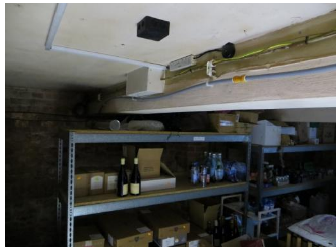
Figure 4.111: Showing the concrete beam in the cellar.
