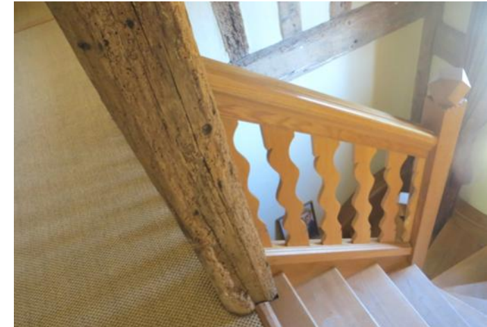
Figure 4.128: Showing the new splat balusters in the stair wing.
