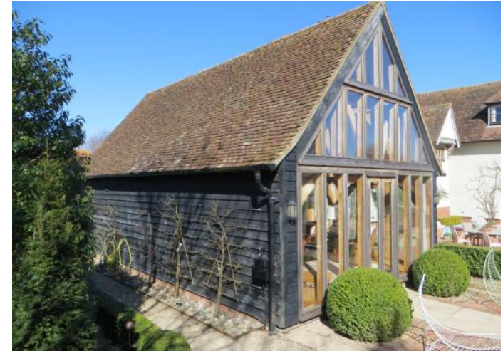
Figure 4.85: Showing the western and southern elevations of the sun room.
