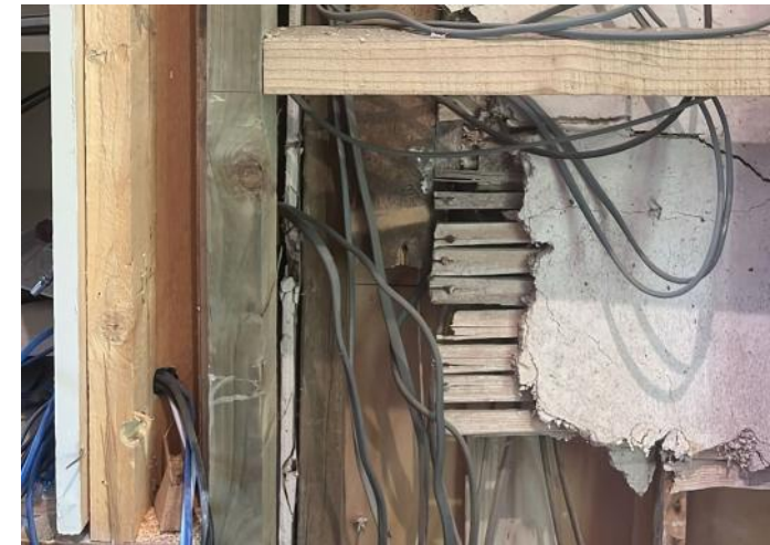
Figure 4.211: Showing the lath and plaster shown in Figure 4.210 in detail.
