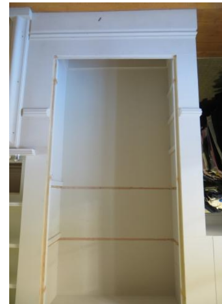
Figure 4.207: Showing the modern built-in wardrobe on the southern side of the chimneybreast. We can see that its rear wall is formed of plywood.
