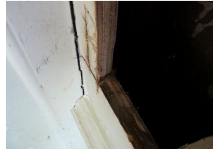
Figure 4.198: Showing the plywood behind the historic corner cupboard.
