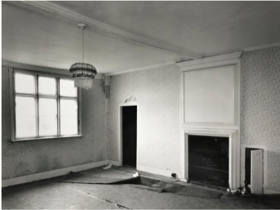
Figure 4.15: 1992-94 photograph showing the western bedroom at first floor (Source: Historic England Archives, Reference: BB92/06147). Note the overmantel and cornice above the fireplace.
