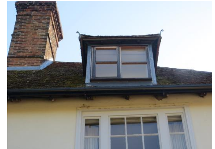
Figure 4.56: Showing the western front dormer.
