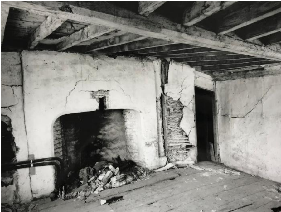
Figure 4.19: 1992-94 photograph showing the south-eastern bedroom at first floor level within the kitchen cross wing (Source: Historic England Archives).
