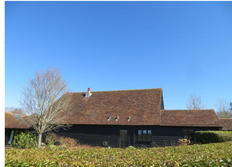
Figure 5.1: Showing the aisled barn west of the Old Manor Farm House.
