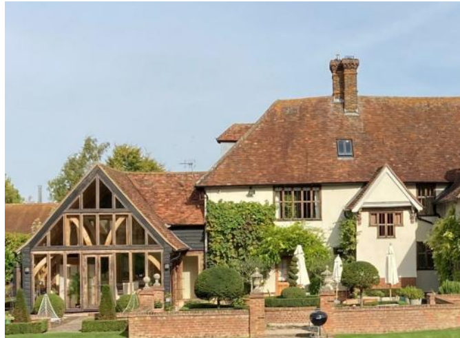
Figure 4.70: Showing the southern elevation of the main range and the sun room.
