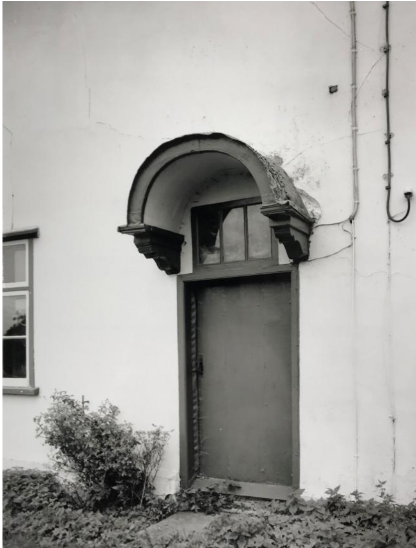
Figure 4.5: 1992-94 photograph (Source: Historic England Archives). Showing the canopy, moulded brackets and door on the northern (front) elevation. Also showing the historic 3-plank door in the main entrance.
