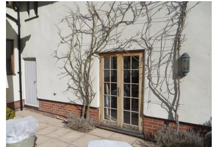
Figure 4.68: Showing the French windows installed on the western elevation of the kitchen cross wing.
