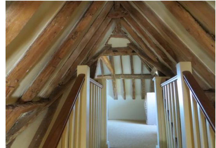
Figure 4.180: Showing the former hipped roof at the south-eastern corner of the main range. Note the mortice holes.
