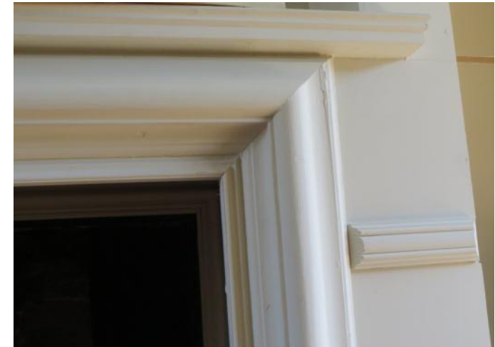
Figure 4.201: Showing the bolection moulding.
