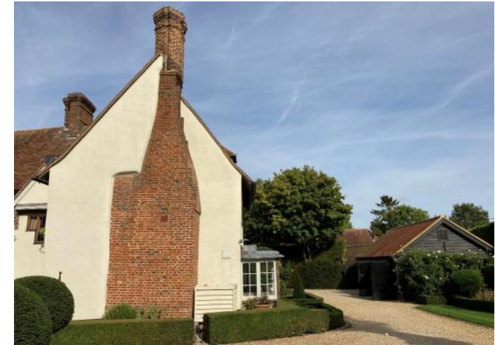
Figure 4.65: Showing the southern elevation of the kitchen cross wing.
