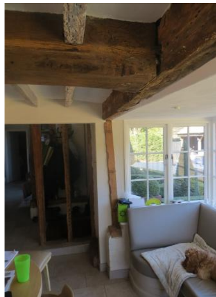
Figure 4.122: Showing the beam adjoining the bay window on the kitchen cross wing's eastern elevation.
