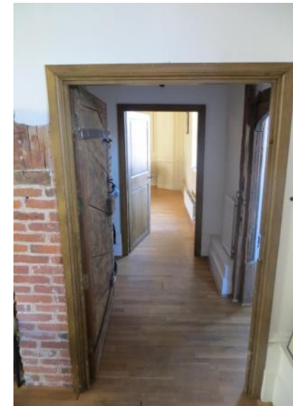
Figure 4.106: Showing the doorway from the dining room into the lobby.
