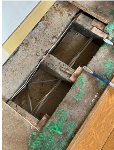
Figure 4.214: Showing the historic boards revealed below the modern floor in the first floor Western Bedroom.
