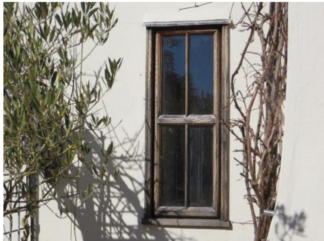
Figure 4.76: Showing the ground window serving the cellar stairs.
