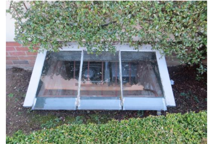
Figure 4.54: Showing the cellar window.
