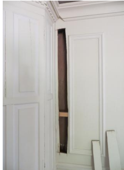
Figure 4.197: Showing the historic corner cupboard in the sitting room. A channel was cut in the modern panelling alongside.
