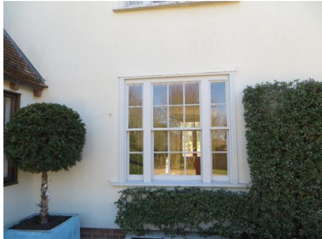
Figure 4.53: Showing the western ground floor window.
