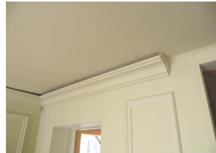
Figure 4.100: Showing a length of modern cornice.
