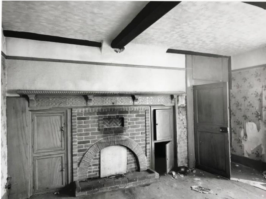
Figure 4.9: 1992-94 photograph showing the interior of the ground floor eastern central room (dining room) looking north-west (Source: Historic England Archives, Reference: BB92/06140).
