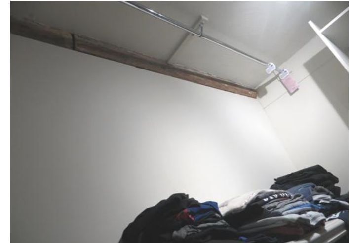
Figure 4.140: Showing the historic timber rail/wallplate on the northern wall of the dressing room.
