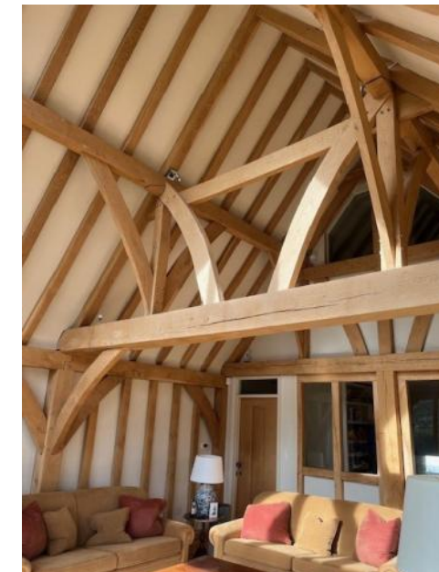
Figure 4.124: Showing a typical purlin roof truss within the interior of the sun room.
