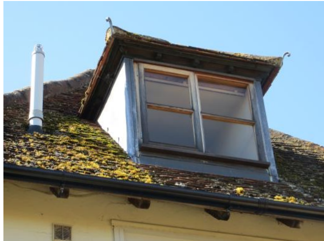
Figure 4.61: Showing the dormer on the eastern hip of the main range's roof.
