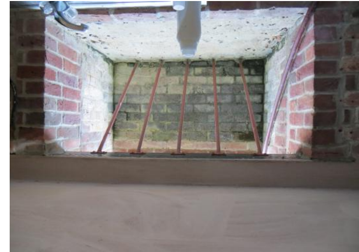
Figure 4.110: Showing the window jambs of the cellar window.
