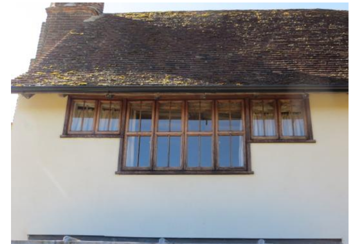
Figure 4.63: Showing the first floor southern window.
