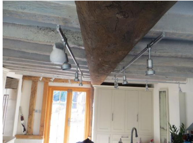
Figure 4.120: Showing the chamfered beam in the kitchen.
