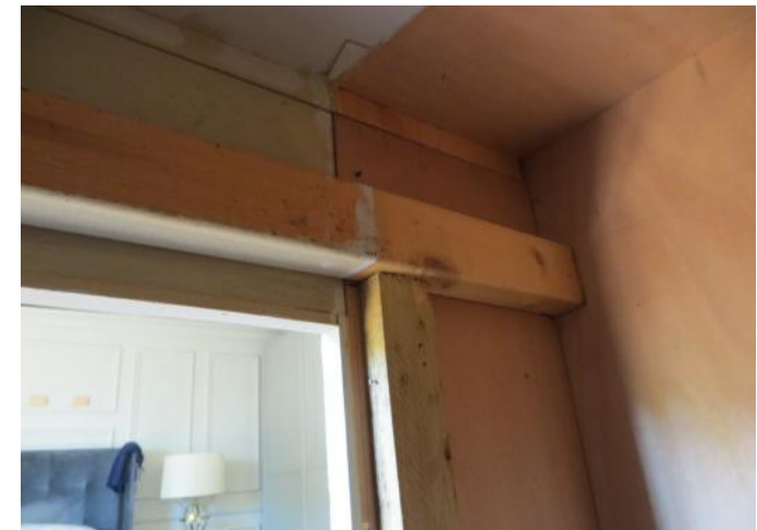
Figure 4.203: Showing the rear side of the chimneypiece.
