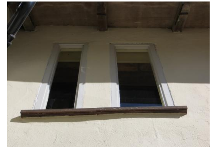
Figure 4.69: Showing the first floor windows at the northern end of the kitchen cross wing.
