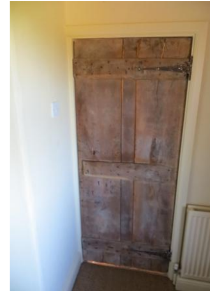
Figure 4.174: Showing the 3-plank door into the room.
