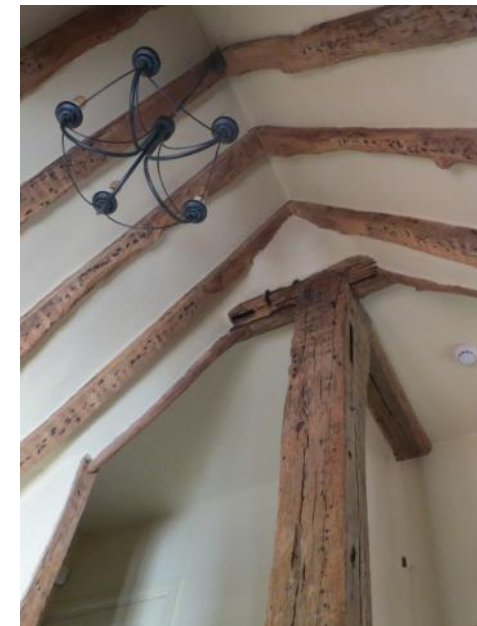
Figure 4.130: Showing the historic rafters in the stair wing's roof.
