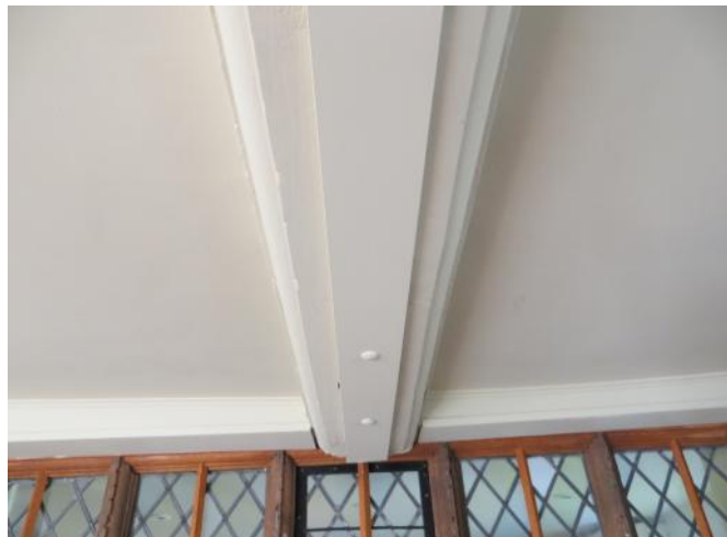
Figure 4.99: Showing one ovolo moulded ceiling beam.
