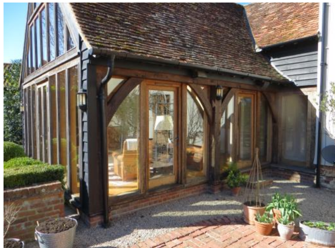
Figure 4.82: Showing the eastern return elevation of the sun room.
