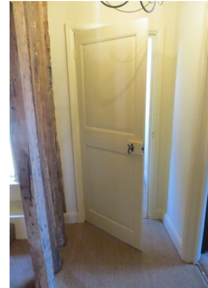
Figure 4.147: Showing the same door as seen at Figure 4.146 as shown from the opposing side.
