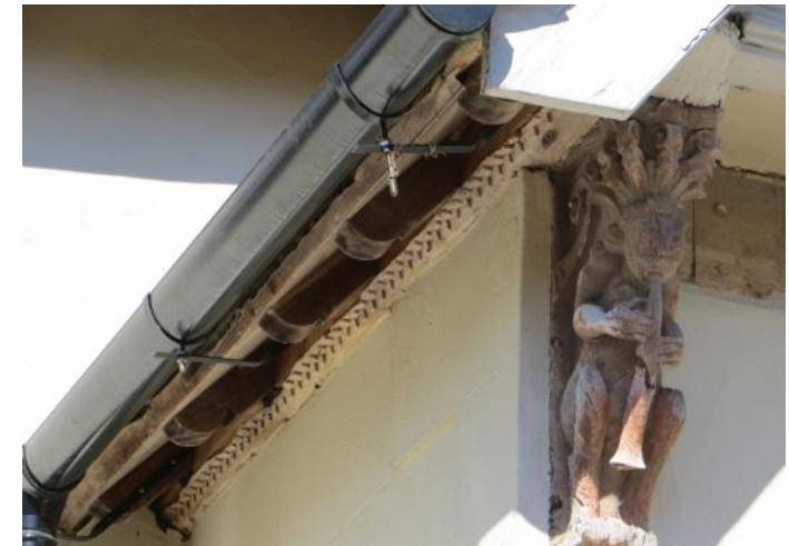
Figure 4.74: Showing dentilled cornice on the western elevation of the stair wing. Note the carved satyr.
