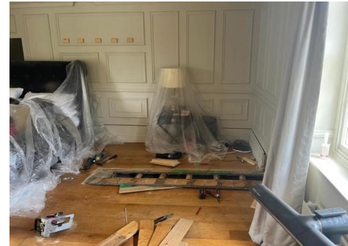
Figure 4.215: Showing the location of the opening up works in the first floor Western Bedroom floor.
