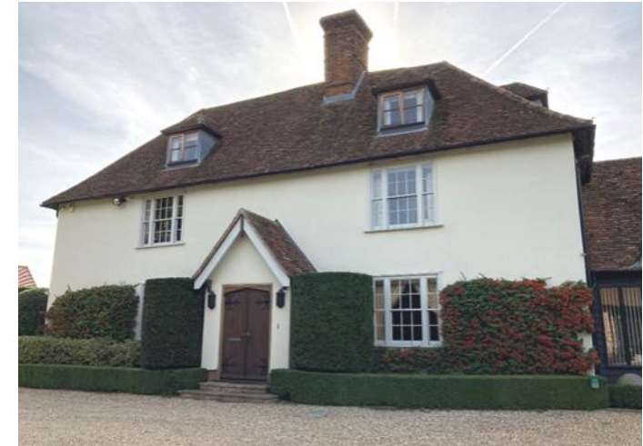
Figure 4.51: Showing the northern (front) elevation.
