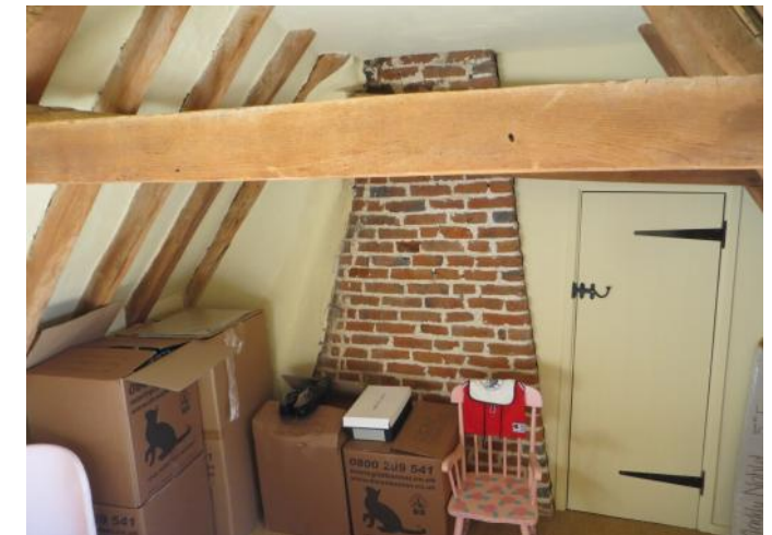
Figure 4.185: Showing the chimneybreast on the western wall does not have a fireplace.
