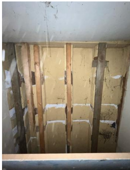
Figure 4.212: Showing the historic timber frame studs revealed on the southern wall of the existing kitchen. Modern battens had been affixed to their northern sides.
