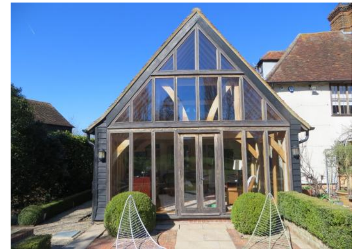
Figure 4.83: Showing the southern elevation of the sun room.
