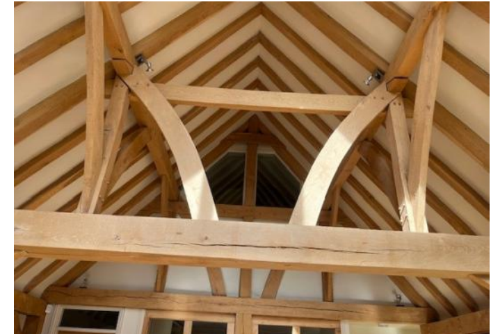
Figure 4.124: Showing a typical purlin roof truss within the interior of the sun room.
