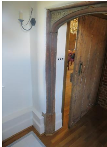
Figure 4.86: Showing the c. 1600 doorframe for the main entrance.
