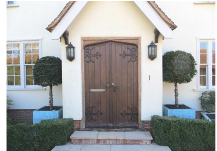
Figure 4.52: Showing the front porch.
