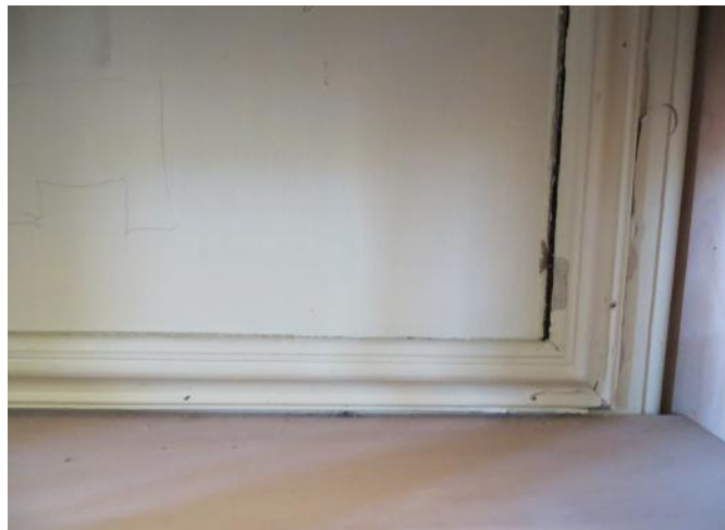
Figure 4.206: Showing part of the 18th century overmantel that survives behind the modern panelling.
