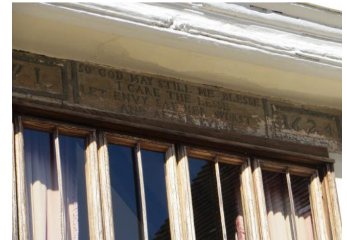
Figure 4.75: Showing the inscription above the first floor window on the stair wing.
