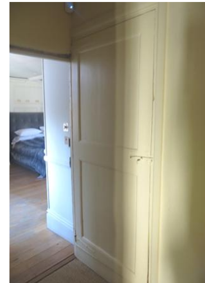
Figure 4.143: Showing the doorway leading to the western loft attic staircase.
