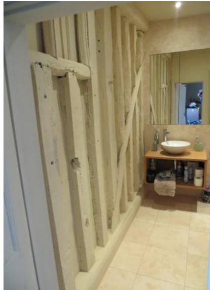
Figure 4.157: Showing the northern wall of the shower room adjoining the north-eastern bedroom.
