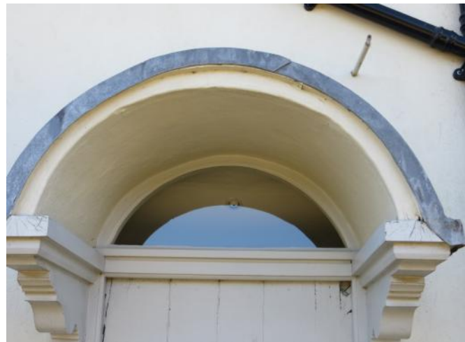
Figure 4.59: Showing the renewed canopy on the eastern elevation.
