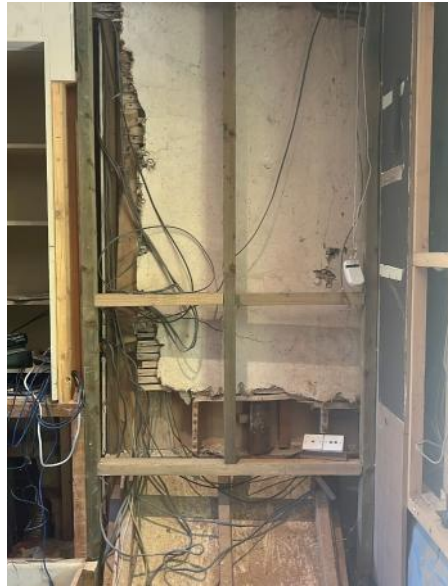
Figure 4.210: Showing the lath and plaster wall found on the wall between the Sitting Room and the cellar staircase wall.
