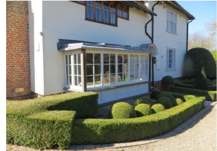
Figure 4.62: Showing the 1990s bay window at the southern end of the eastern elevation.
