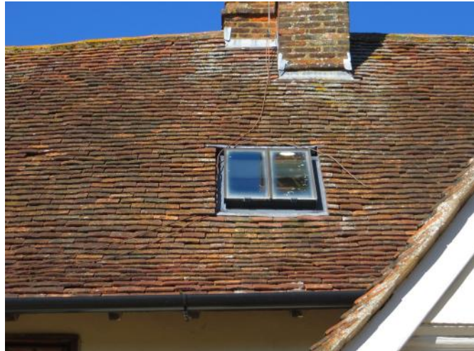
Figure 4.80: Showing the conservation rooflight on the main range's southern roofslope.
