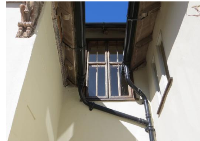
Figure 4.72: Showing the first floor window at the eastern end of the main range.
