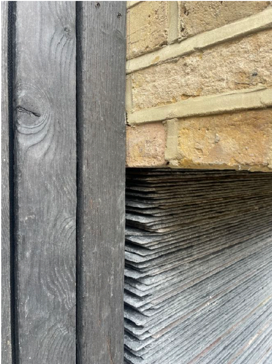
An example of charred larch rain screen cladding (left of photo)
