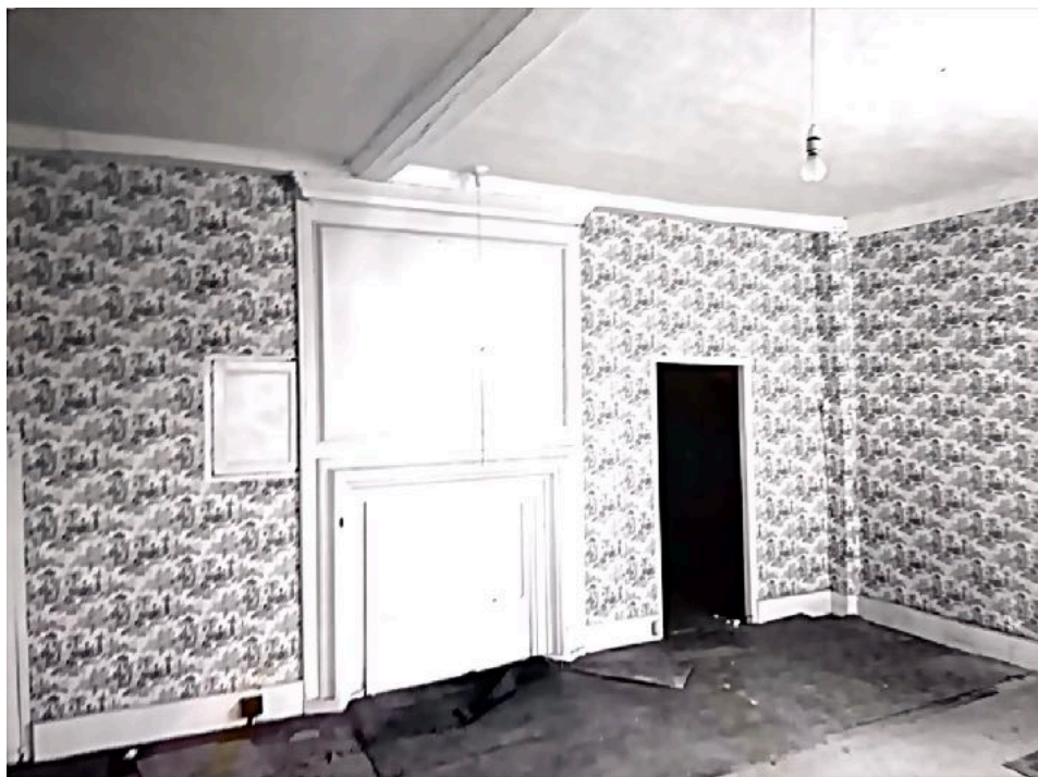
North-west corner of bedroom 2 pre 1990 showing a previous door opening to be reinstated.
