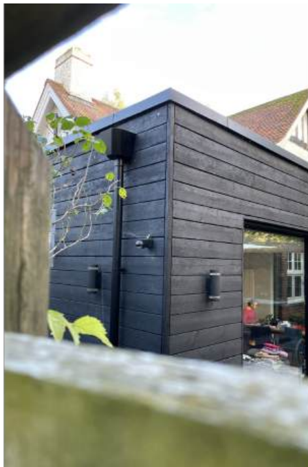
5 Norton Road timber used on side viewable from the street – older house
