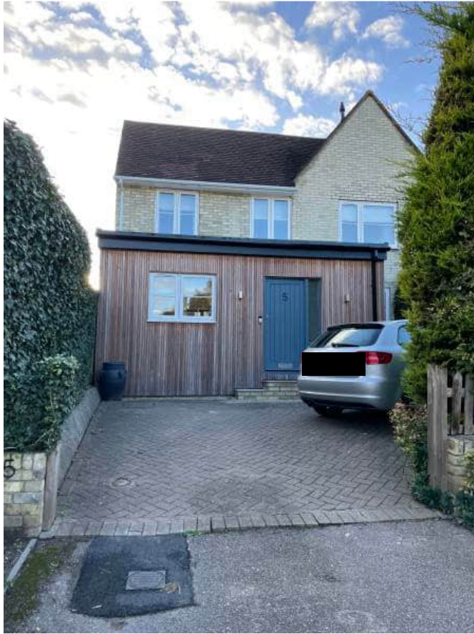
3 Norton Road – timber used on a porch
