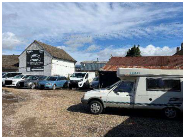
Photograph Six: Courtyard area in centre of site. Covered with gravel (i.e. No hardstanding)
