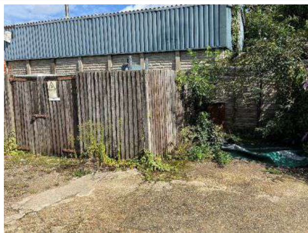
Photograph Seven: Electrical sub-station, just beyond site boundary.
