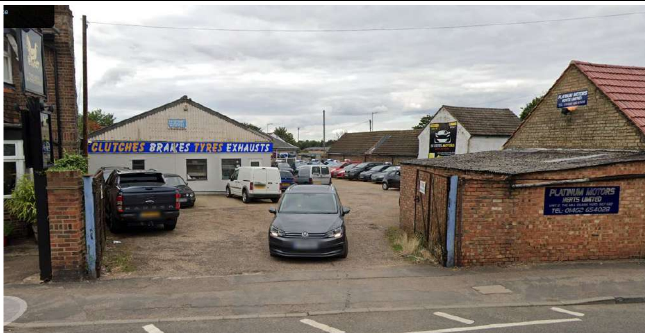
Photograph One: Site view from South Road, with main workshop on left hand side.
