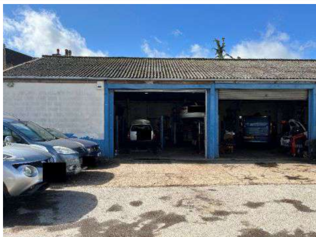
Photograph Two: Main workshop building, currently in use for vehicle maintenance / repair, located towards the western end of the site.
